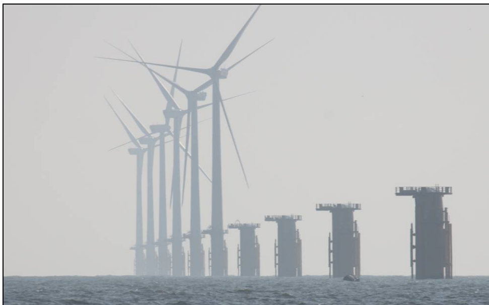
Wind turbines (in construction) at Thanet © Vattenfall Wind Power Limited
