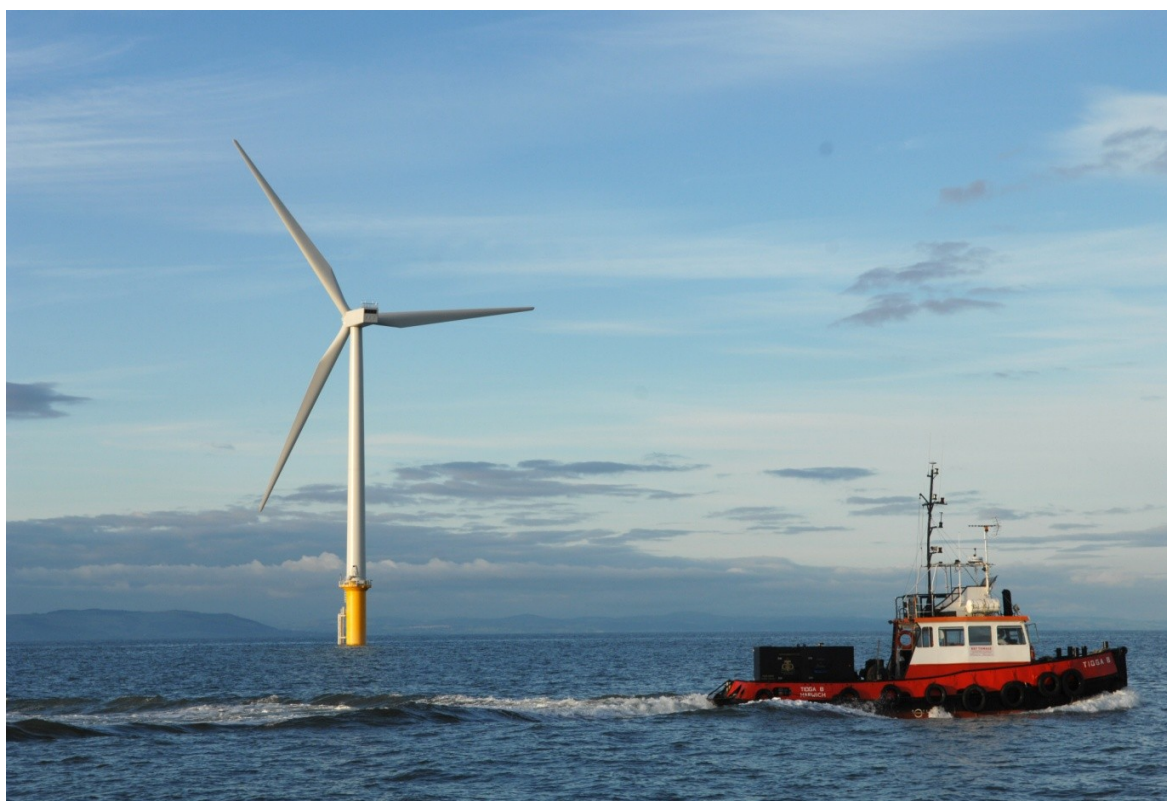
Figure 6: Maintenance vessel at the existing Burbo Bank offshore wind farm
