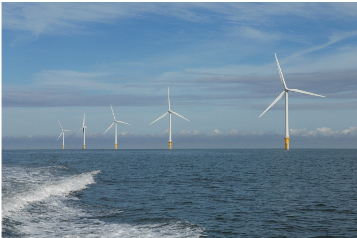
Figure 3: Wind turbines at the operational Burbo Bank offshore wind farm
