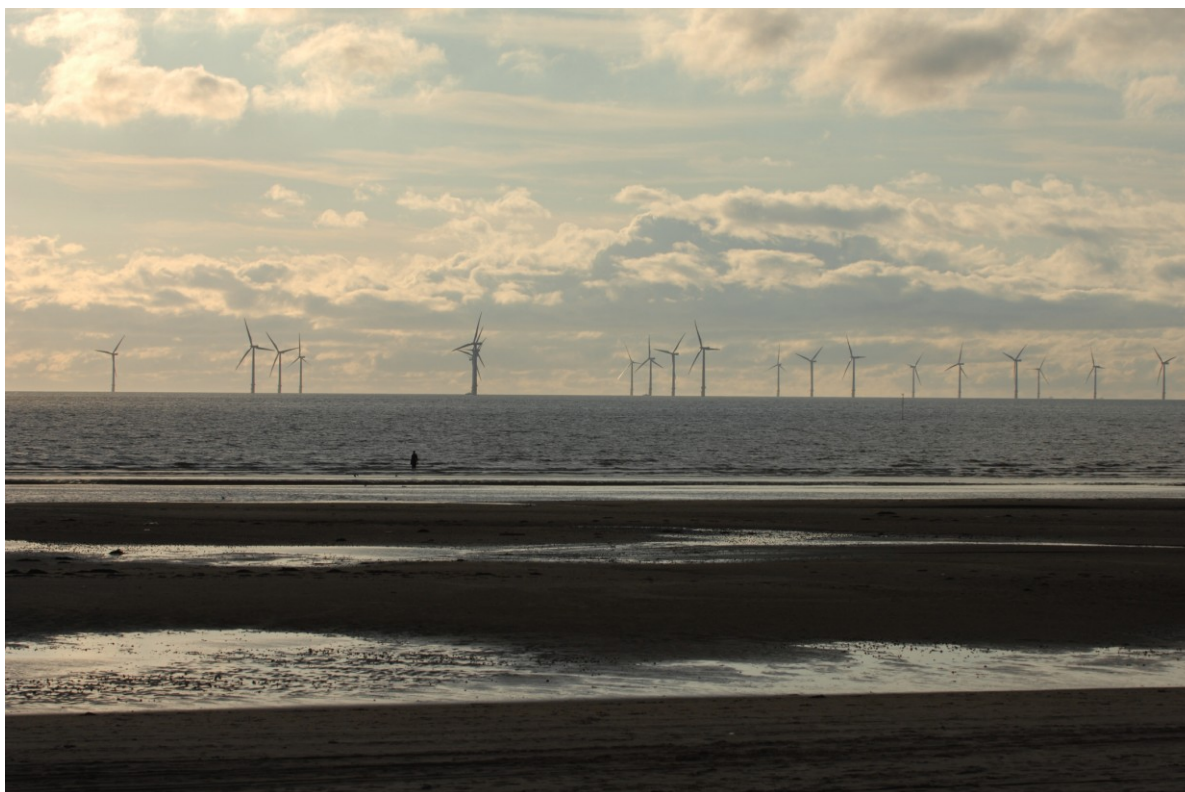
Figure 1: Wind turbines at the operational Burbo Bank offshore wind farm
