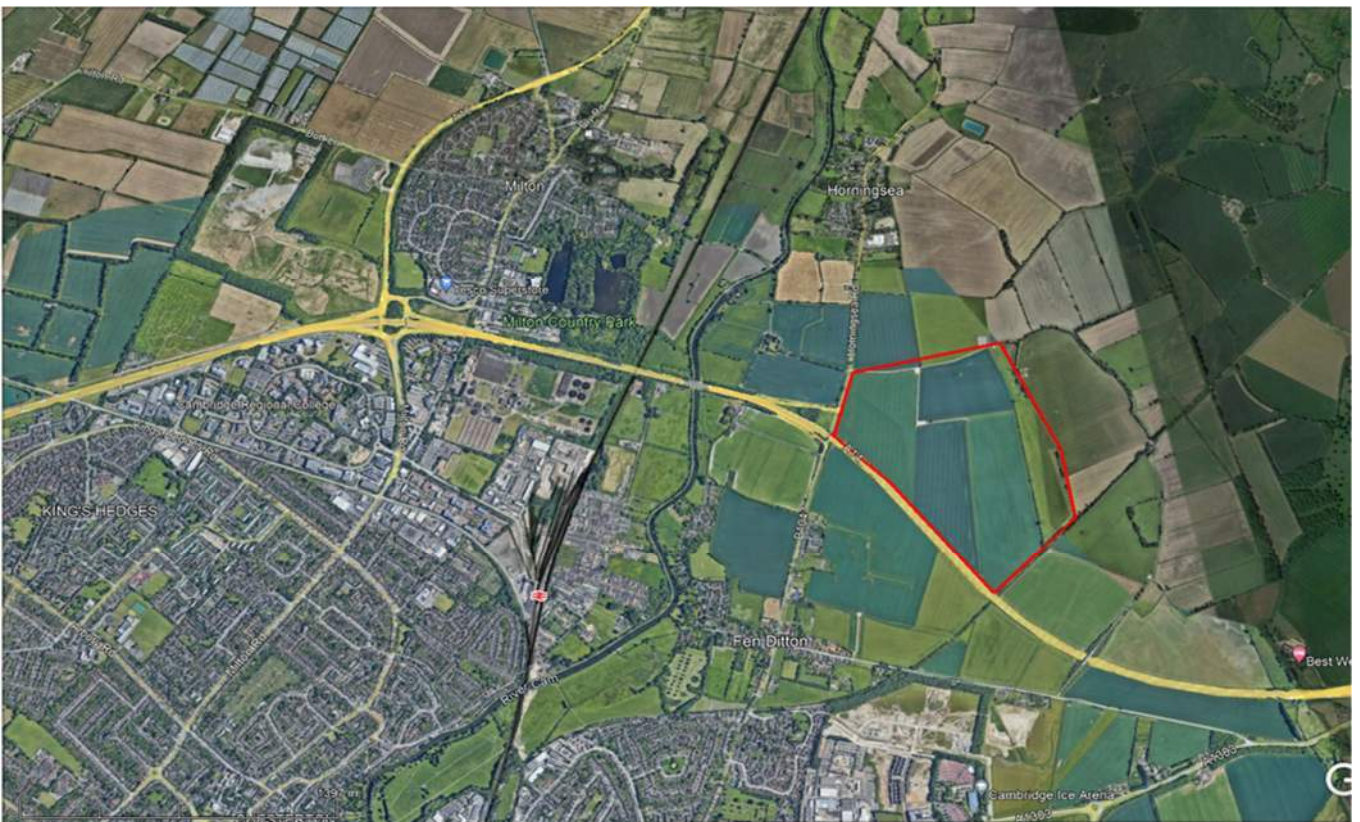
Figure 3: Aerial view of proposed relocation site.
