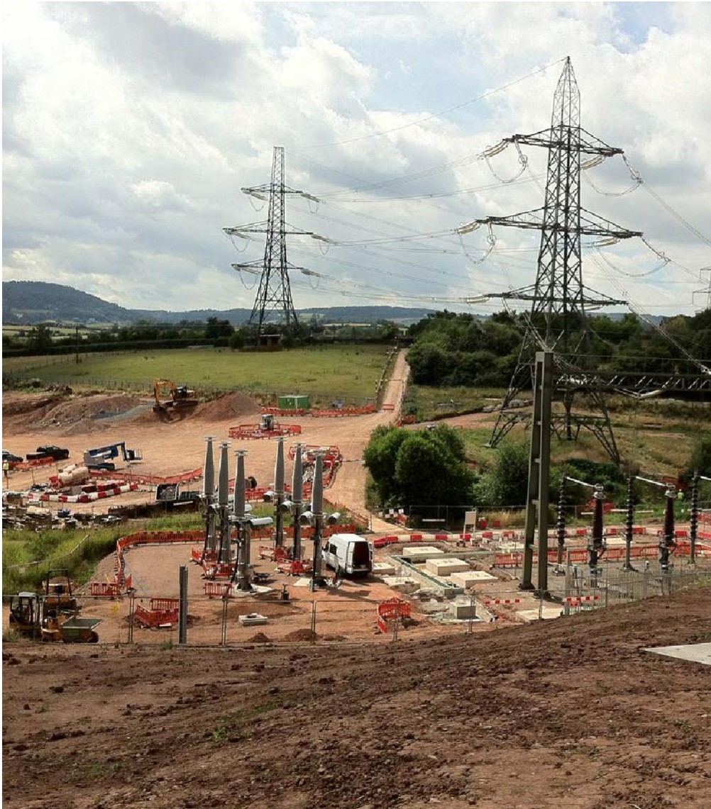
The undergrounding of electricity cables at Ross-on-Wye
