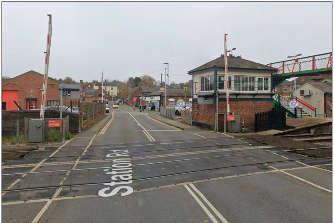
Figure 2.3: View of Existing Site Carriageway
