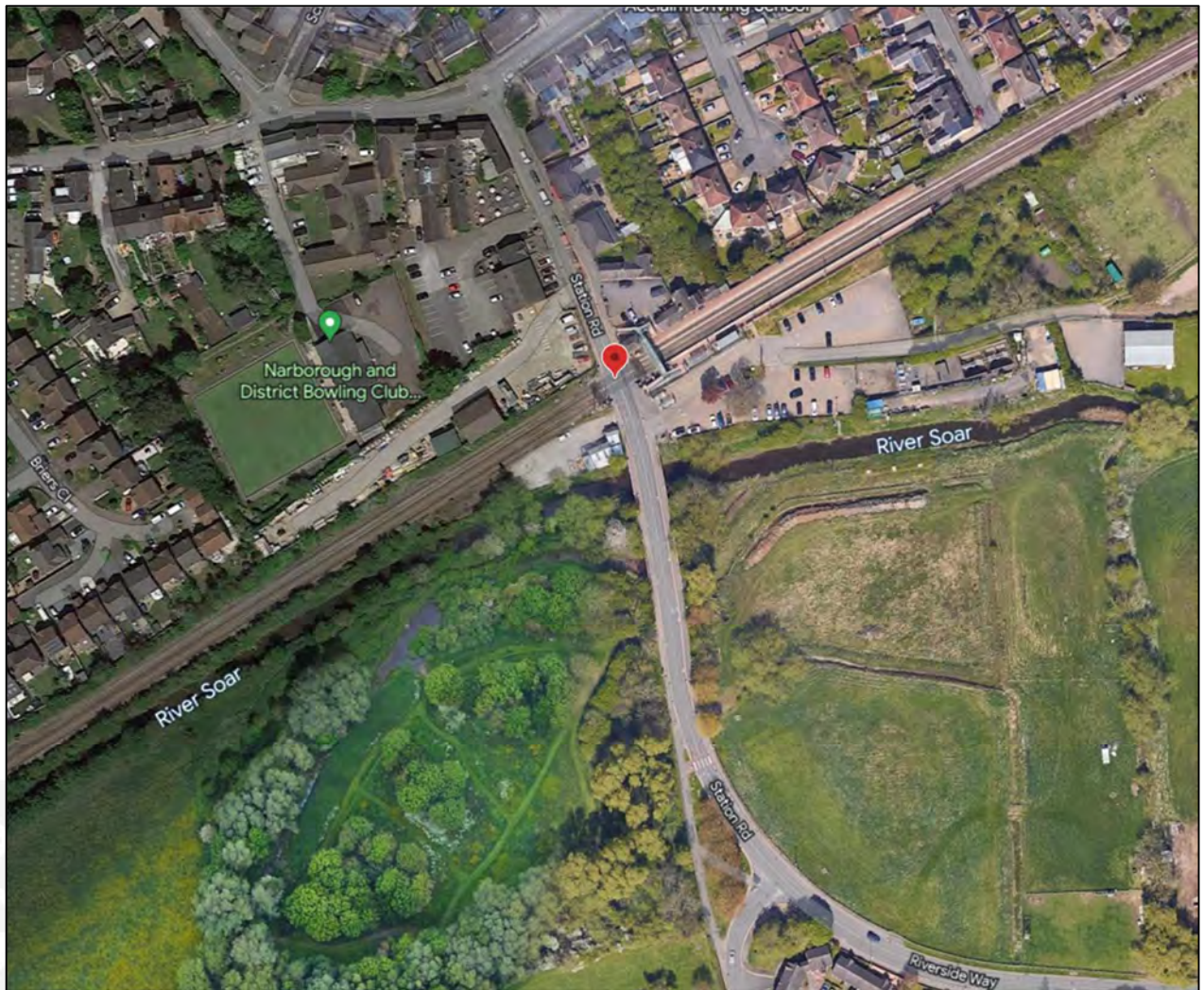
Figure 2.1: Aerial View of Level Crossing and Local Junctions
