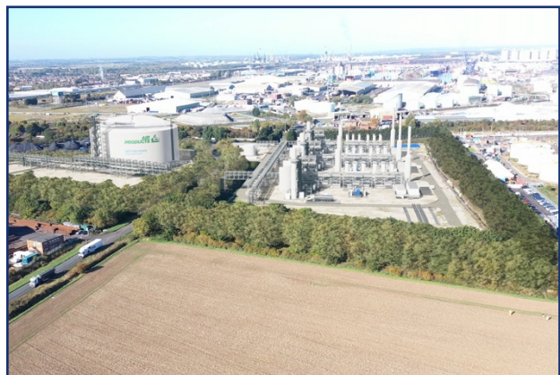
Proposed East Site, including hydrogen processing facility and temporary construction area in the foreground
