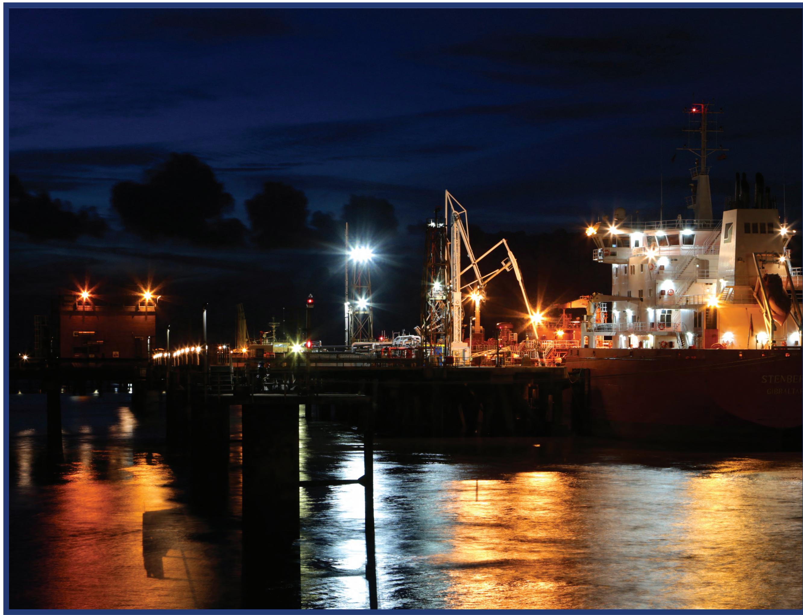
Immingham gas jetty. Photo Credit: David Lee Photography
