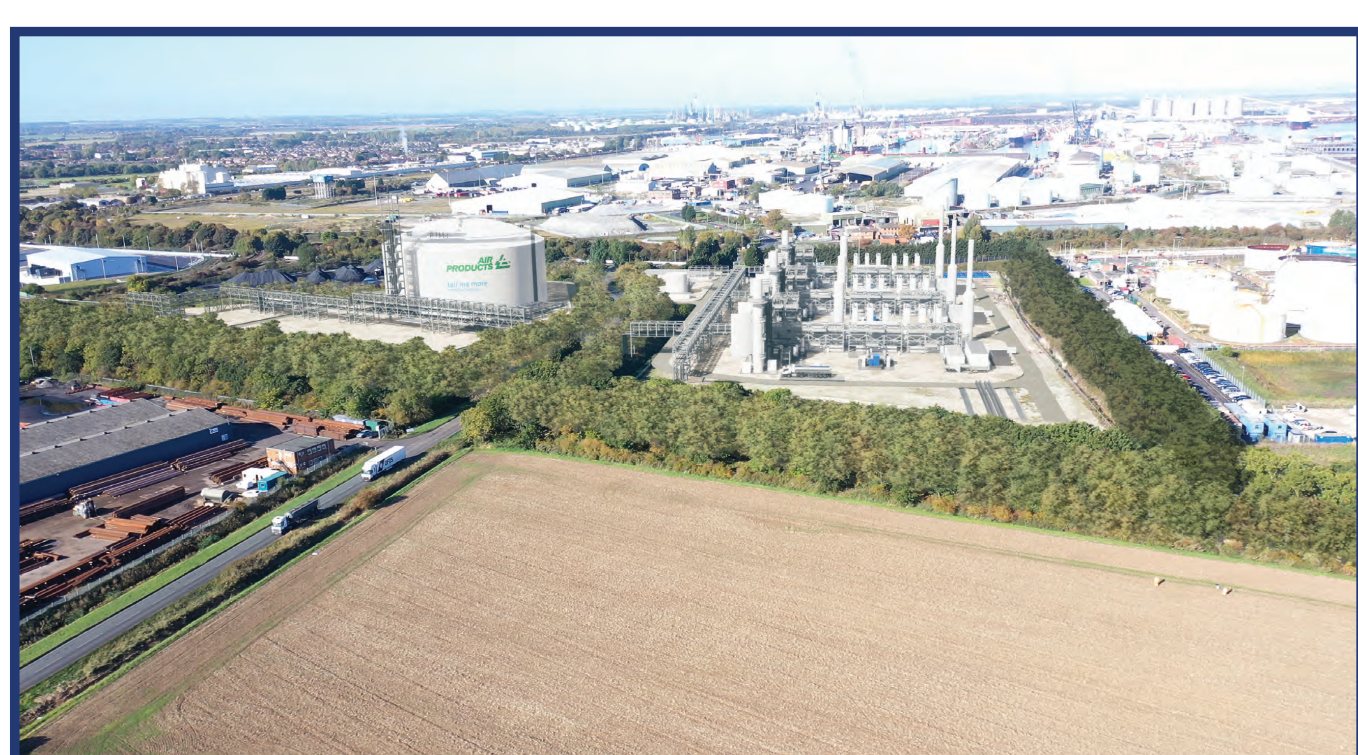
Proposed East Site including hydrogen processing facility and temporary construction area (foreground)
