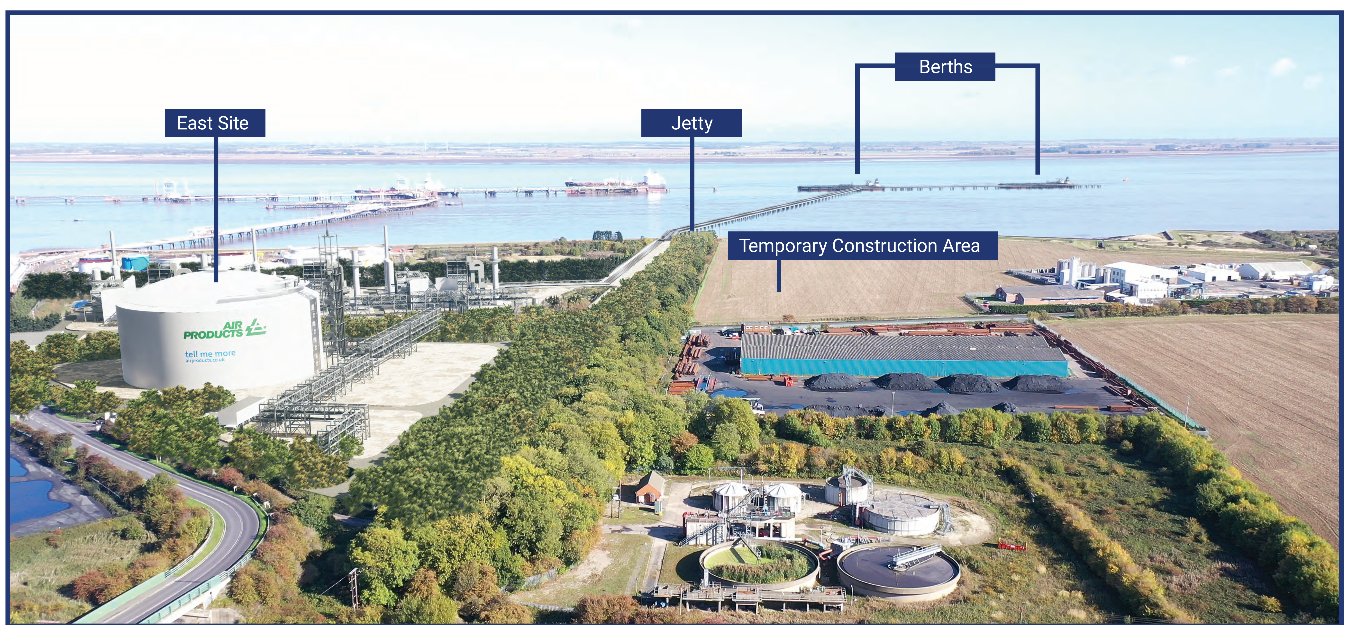
This image shows the proposed Jetty, East Site and Temporary Construction Area, looking towards the Humber
