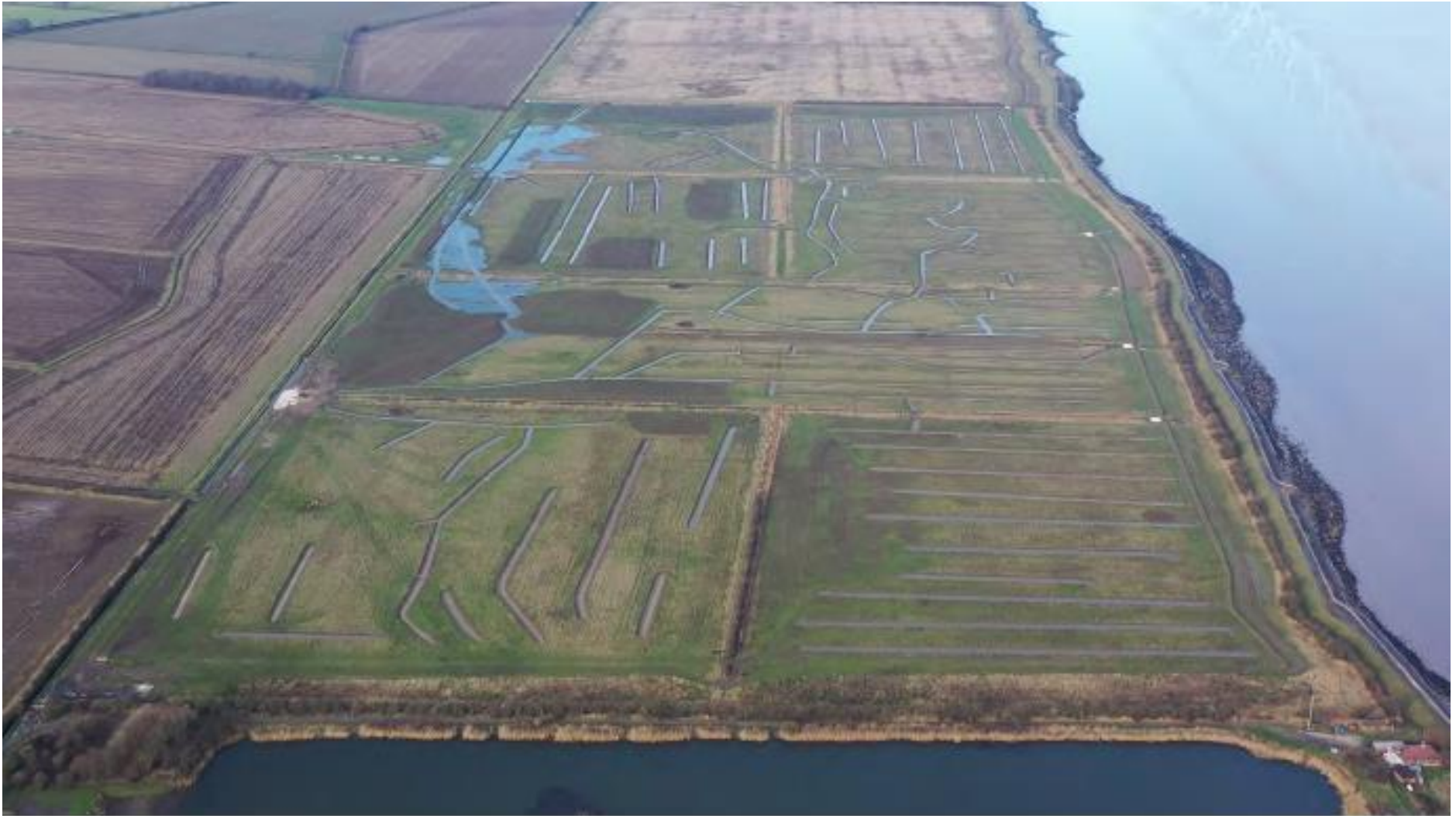
Figure 3. Aerial view of completed HMWGS
