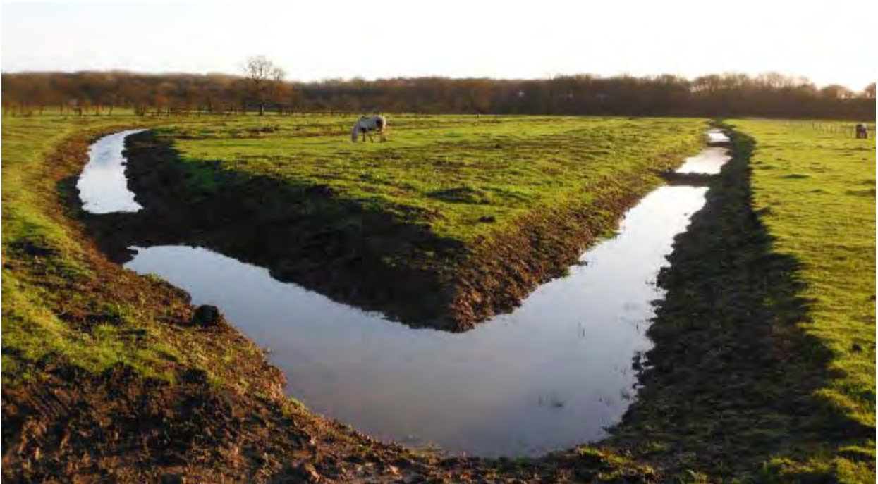
Figure 6-5: Linear scrapes at same site with saddles one month after installation
