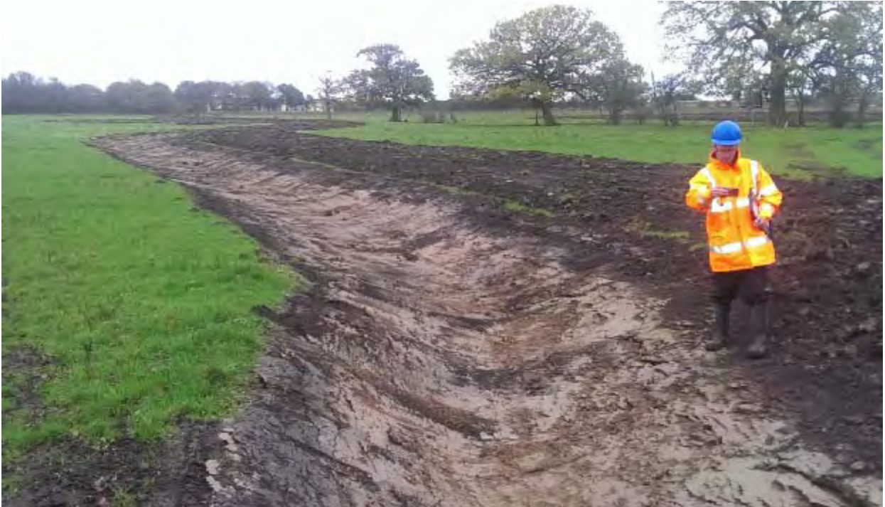
Figure 6-5: Linear scrapes at same site with saddles one month after installation
