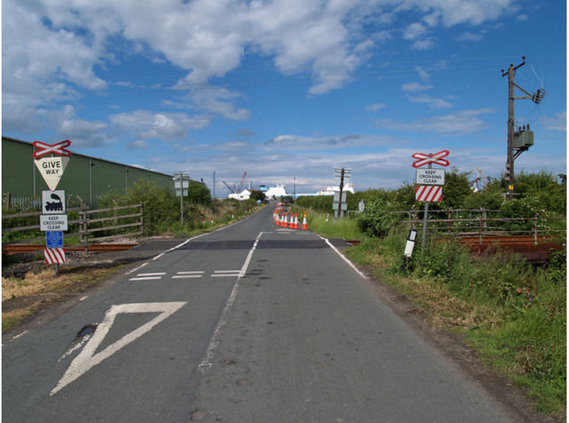
Plate 1: Haven Road Level Crossing looking towards the Estuary. This would be improved but retained within the Killingholme Loop. Note: it is ungated
