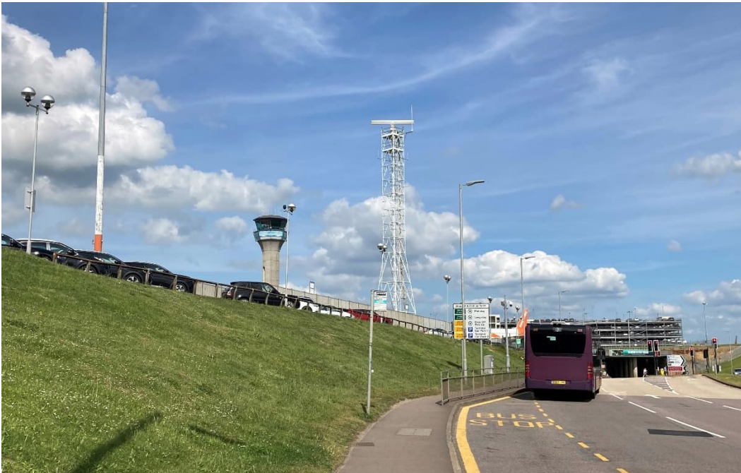
Figure 5.28: Photograph showing existing Surface Movement Radar (centre) with ATC to the left
