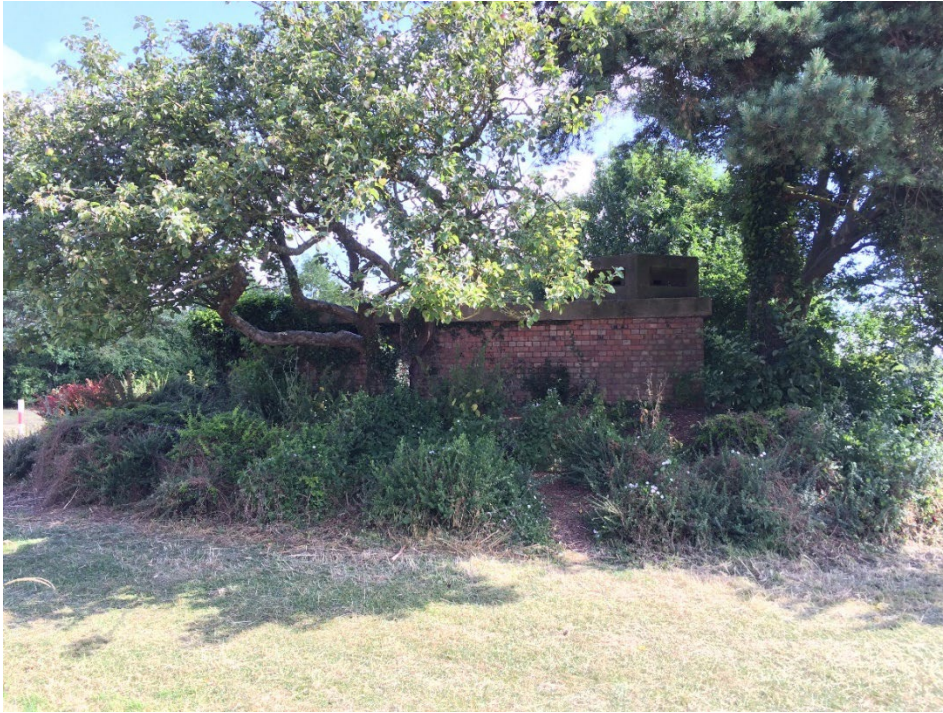
Photograph 1: Pillbox supporting common pipistrelle roost
