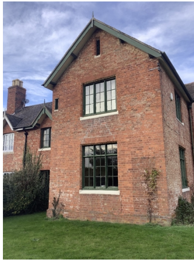
Photo 2-3 BU_638 confirmed common pipistrelle hibernation roost within the roof void.
