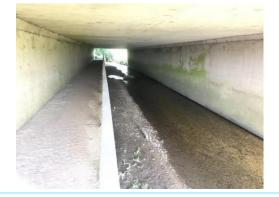
Photo 8 (2019): View through the <u>Riverthe</u> <u>River</u> Chelt Culvert showing fine sediment deposition. Trash and vegetation which were assumed to be flood deposits observed on the concrete walkway indicates flows have been much higher within this reach.
