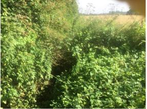
Photo 18 (2019): Drain 18 at its source alongside Hayden Lane. The channel was overgrown with vegetation and there was no perceptible flow. There were fine sediments on the bed and vegetation on both banks.
