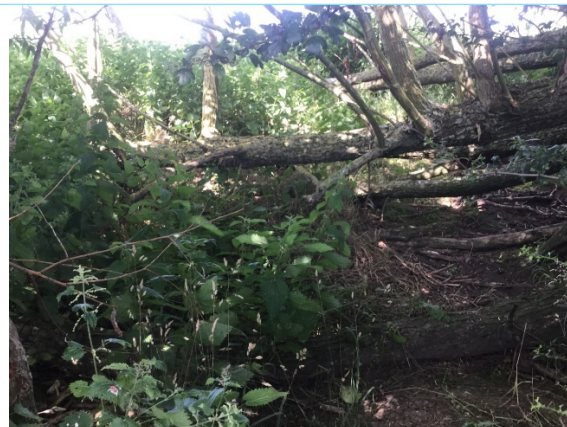
Photo 16 (2019): Drain 12 upstream of Withybridge Lane. There was no flow within the
