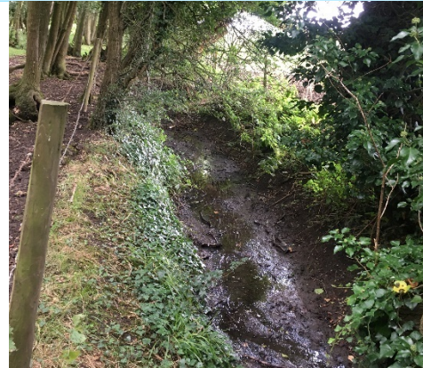
Photo 14 (2019): The channel was heavily shaded by dense scrub and woodland downstream of the Leigh Brook Culvert. The earth banks were shallow sloping and sparsely vegetated, and no vegetation was recorded within the channel. The channel was almost dry with some pools of standing water. Cattel poaching was recorded. (Image taken by ecology team: September 2019).
