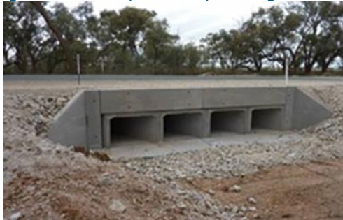
Figure 5-3 - Example multi-span bridge/culverts
