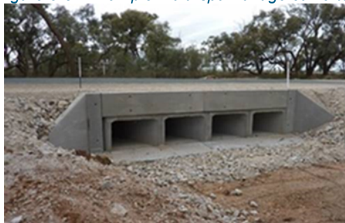
Figure 5-3 - Example multi-span bridge/culverts
