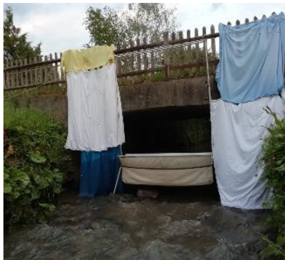
Figure 2-4 – Bat Trapping Location 3, River Chelt M5 Culvert
