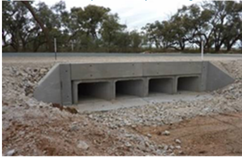
Figure 5-3 - Example multi-span bridge/culverts
