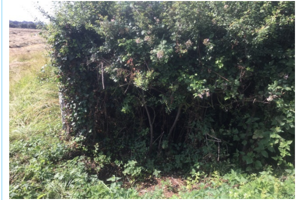
Photo 11: Drain 16 at confluence with Drain 20. Drain 16 is culverted under a farm access track at this location, but runs parallel to the Old Gloucester Road B4634 acting as road drainage (SO 90620 23925)
