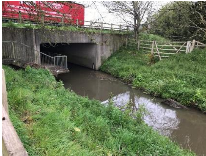
Figure 2-3 – Bat Trapping Location 2, River Chelt M5 Culvert
