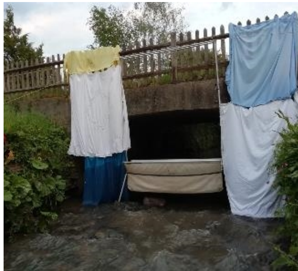
Figure 2-4 – Bat Trapping Location 3, River Chelt M5 Culvert
