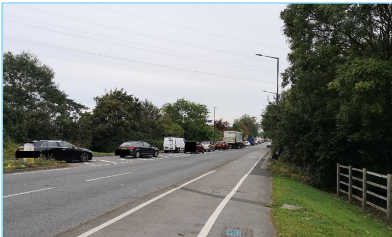
Figure 6-5 - Queues from A46-Shannon Way junction
