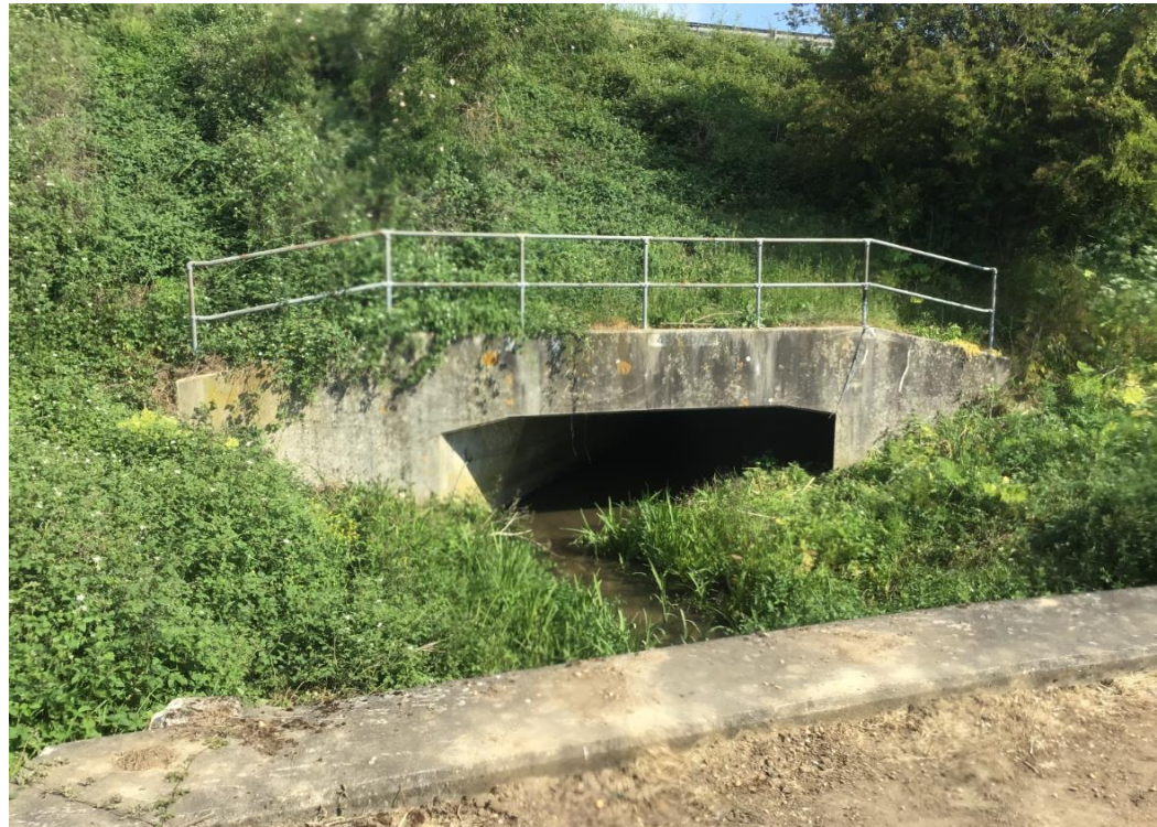
Plate 1: Boreham Brook Culvert
