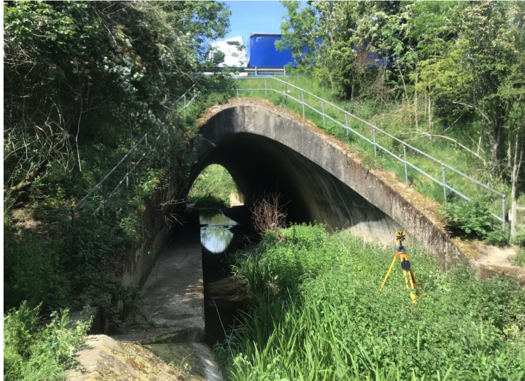
Plate 5: Domsey Brook Bridge (west)
