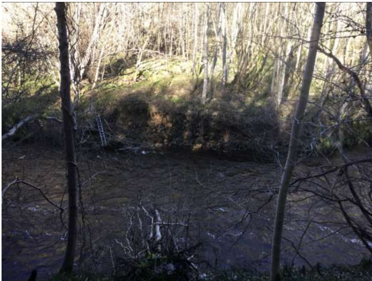
Figure 2 - Eroding Toe of Landslide approx. 500m Upstream of Existing Bridge
