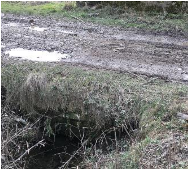
Figure 7-2 – Tributary of Embleton Burn Culvert (Outlet)
