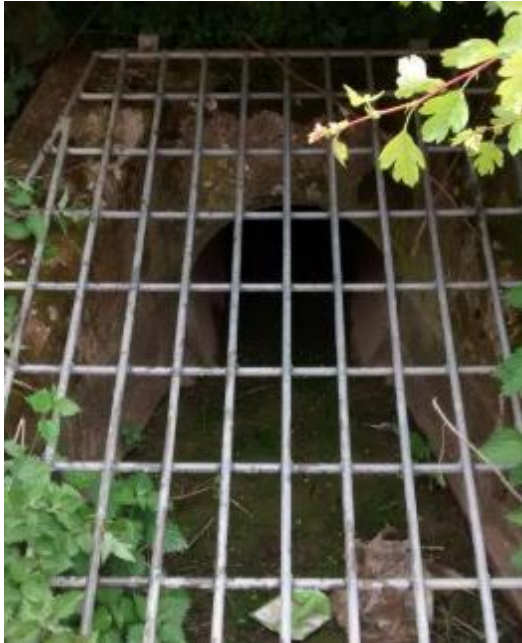
Figure 6-2 – B6347 Western Culvert (Inlet)
