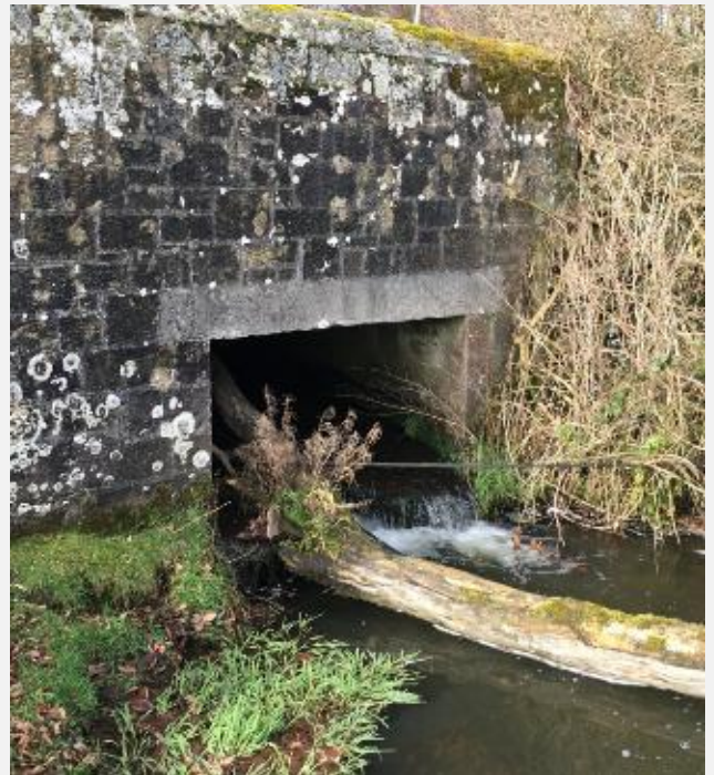
Figure 8-5 – Shipperton Bridge (Outlet)
