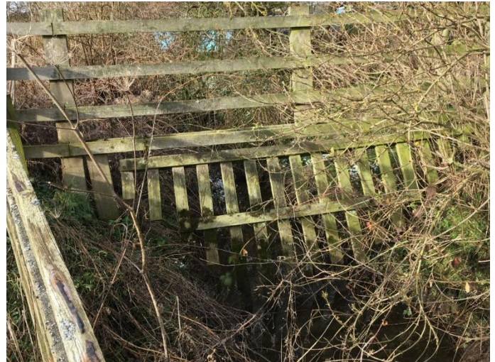
Figure 6-7 – Debris Fence along Unnamed Western Tributary of Kittycarter Burn
