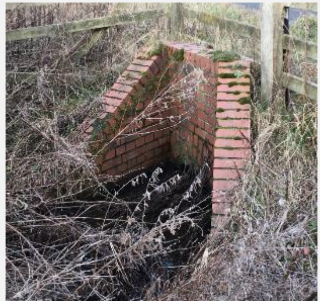
Figure 6-5 – B6347 Eastern Culvert (Inlet)
