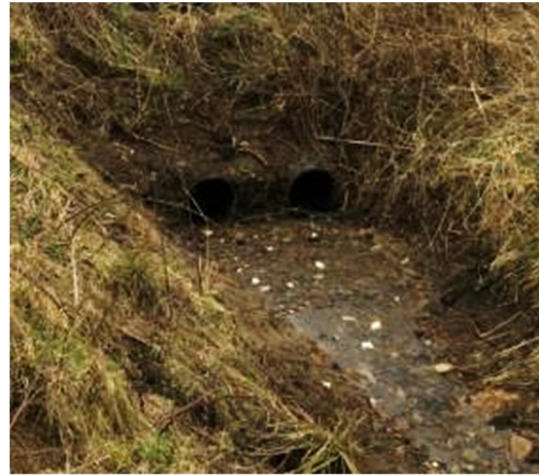
Figure 4-12 – Farm Access Culvert One Inlet
