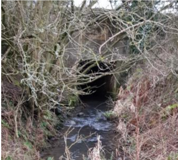
Figure 5-5 – Culvert Underneath the B6341 (Inlet)
