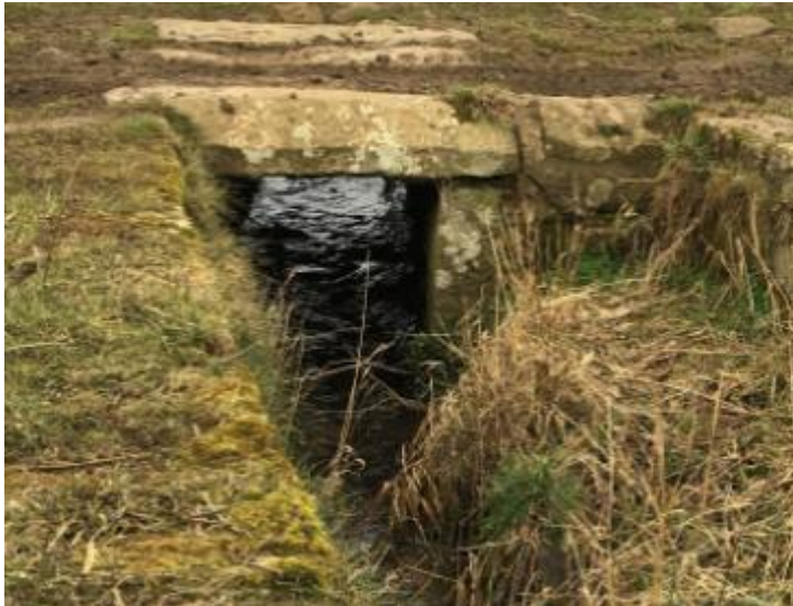
Figure 4-5 - Public Right of Way Denwick Burn Crossing
