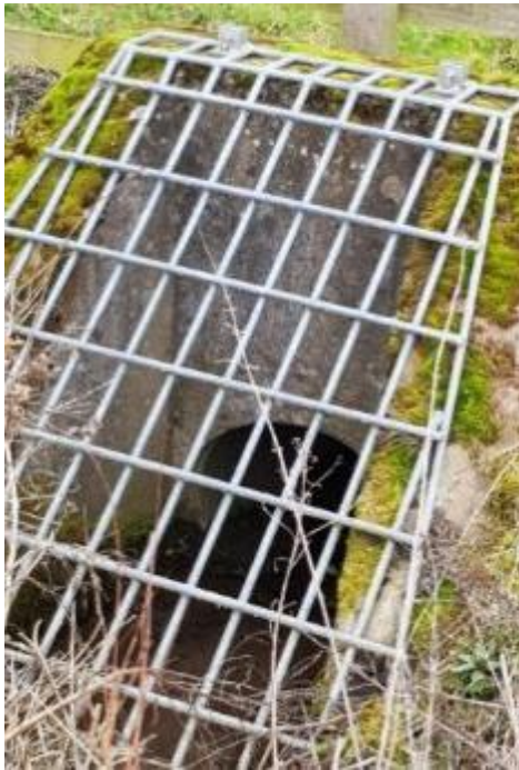
Figure 4-2 - Heckley Fence Culvert Inlet
