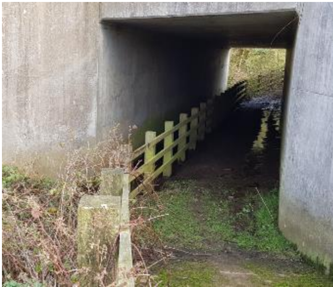
Figure 5-2 – White House Burn A1 Culvert (Outlet)
