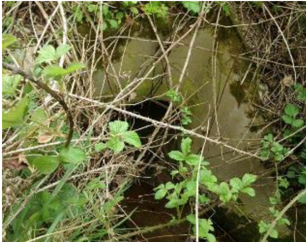
Figure 4-11 – Denwick Burn A1 culvert One inlet
