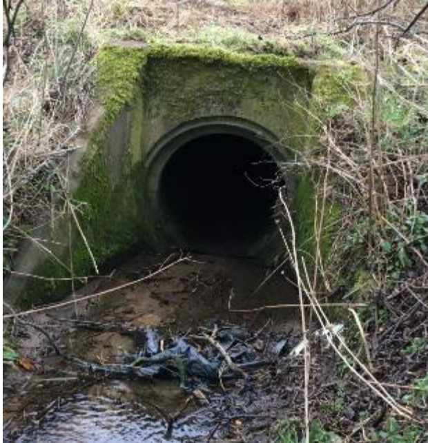
Figure 4-7 - Denwick Burn A1 Culvert Three Inlet
