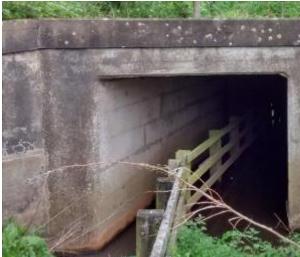
Figure 6-6 – Western Tributary of Kittycarter Burn Culvert Underneath A1 (Inlet)
