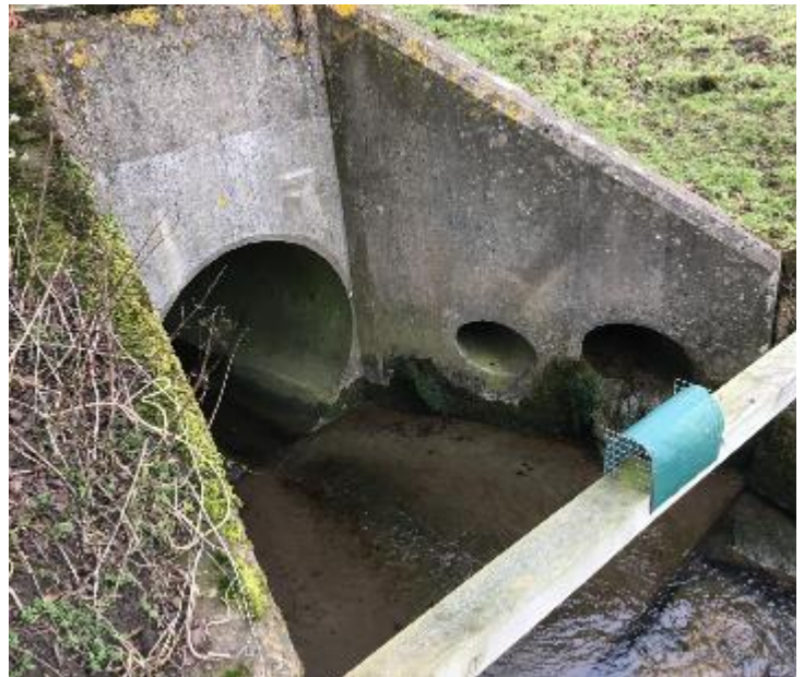
Figure 4-4 - Denwick Burn A1 Culvert Four Outlet
