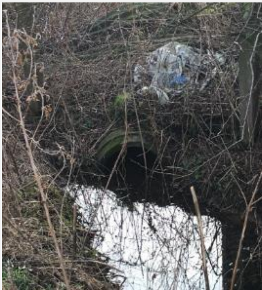
Figure 6-4 – Small Access Track Culvert (Outlet)
