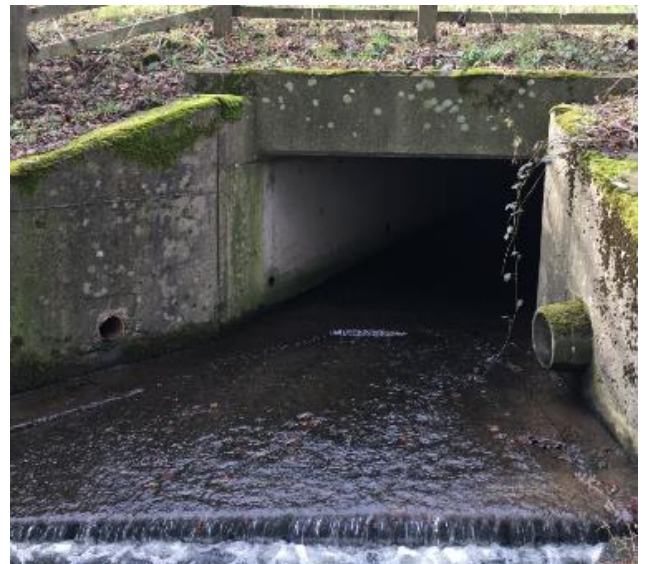
Figure 8-3 – Shipperton Burn A1 Culvert (Outlet)
