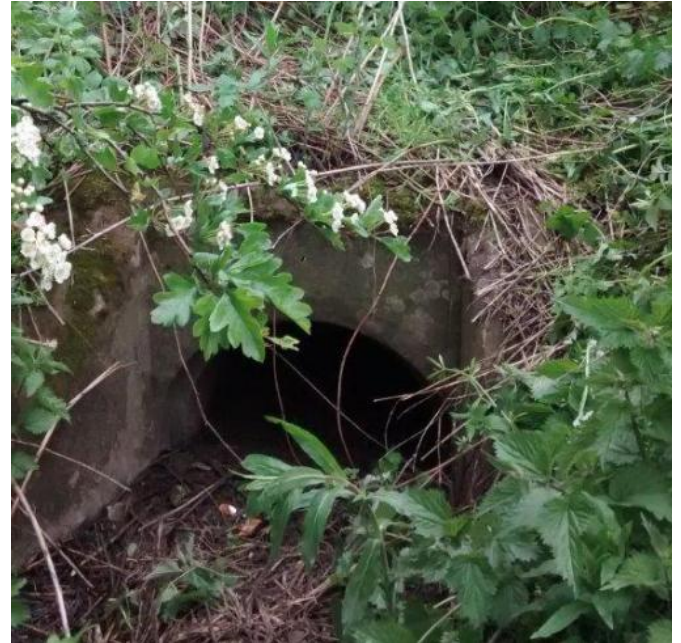
Figure 6-3 – Southern Tributary A1 Culvert (Inlet)
