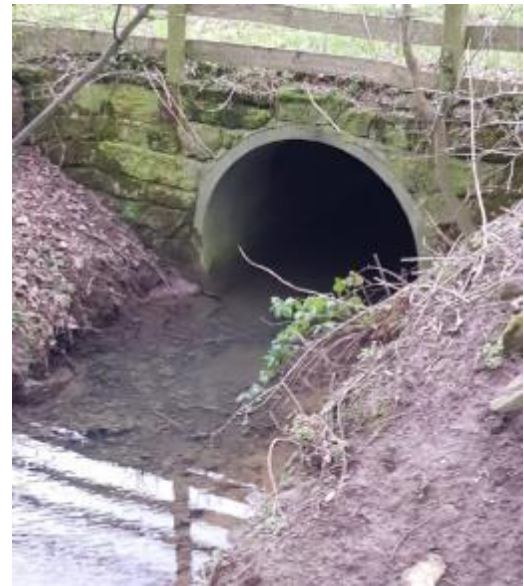
Figure 5-3 – White House Burn Field Access Culvert (Outlet)
