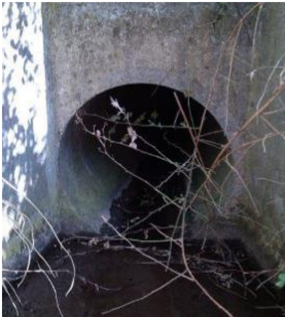
Figure 4-3 - Denwick Burn A1 Culvert Four Inlet
