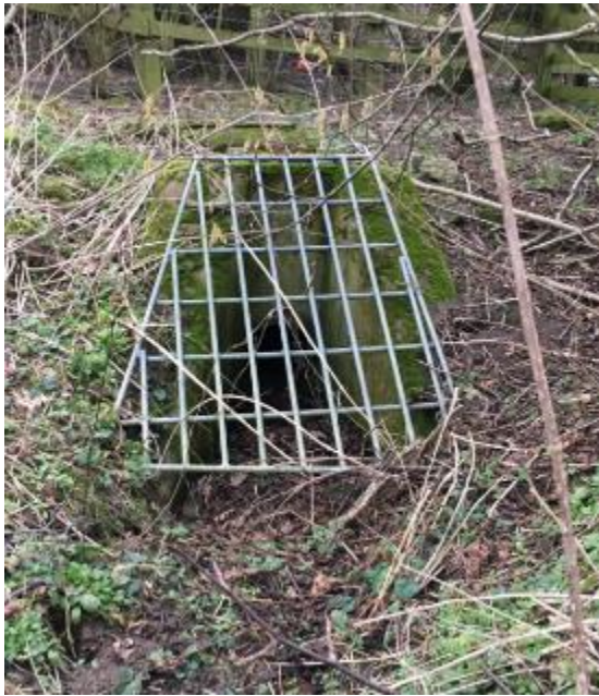
Figure 4-8 - Denwick Burn A1 Culvert Two Inlet
