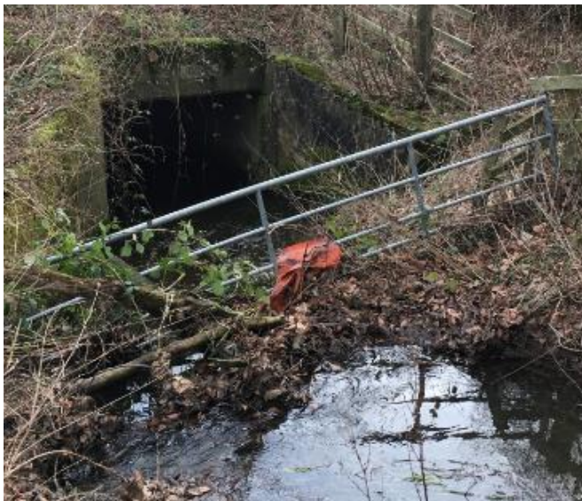
Figure 8-2 – Shipperton Burn A1 Culvert (Inlet)
