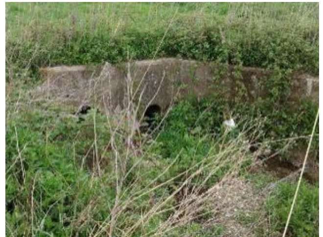
Figure 4-10 – Farm Access Culvert Two Outlet
