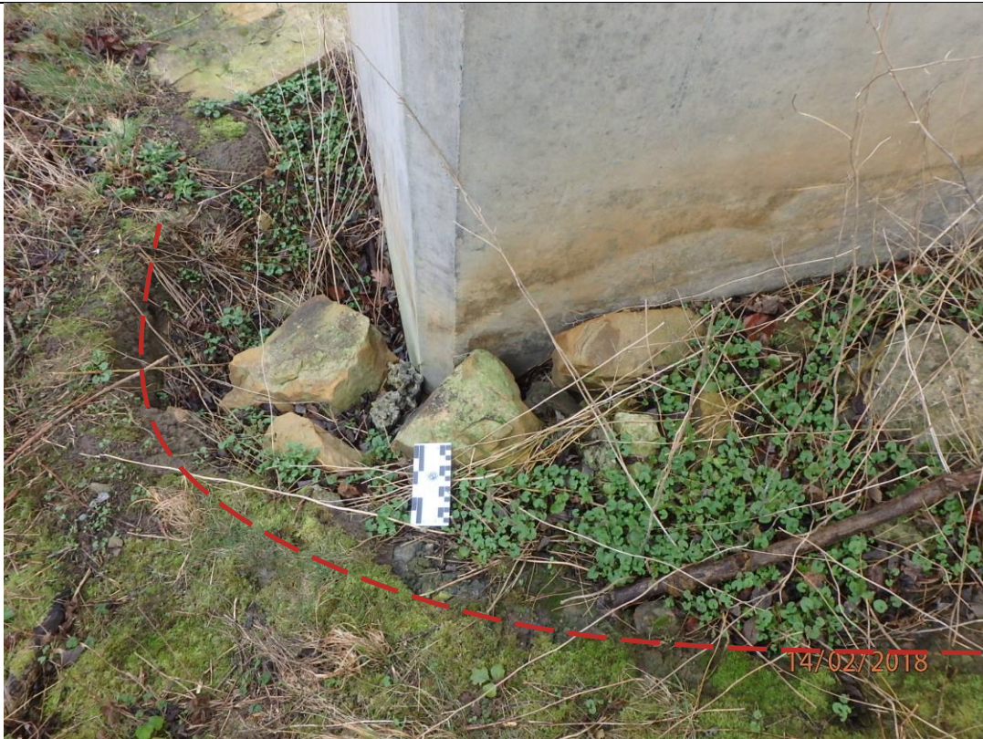
Photograph 6 – Apparent scour around the base and sides of the southern pier of the existing A1 bridge. Note the sandstone blocks which appear to have been intercepted by the structure. The upper divisions on the scale marker are centimetres.
