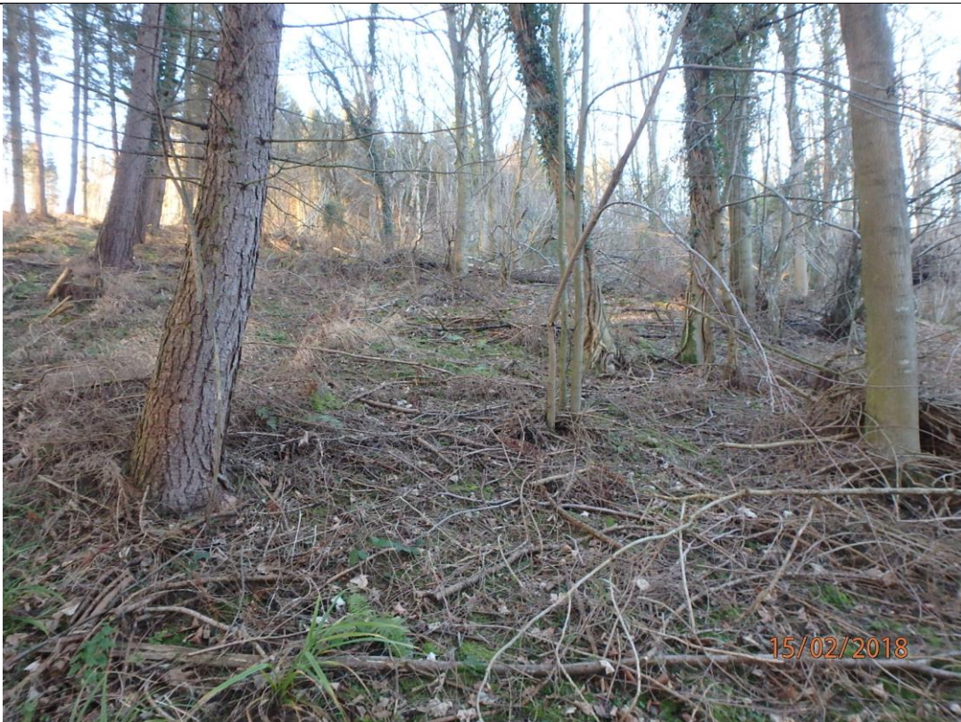
Photograph 19 – Proposed western extent of the zone of instability to the west of the existing A1 bridge northern abutment. Note the change in land use to coniferous forestry to the west.
