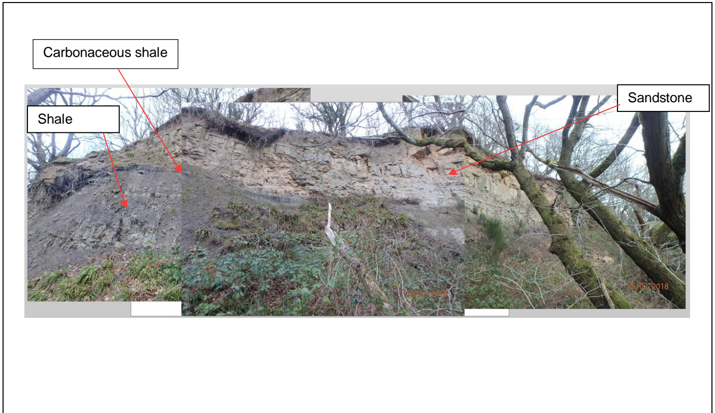
Photograph 16 – Bed rock geological succession observed to the east of the study area (photograph mosaic). This photograph demonstrates the change from the underlying shales to the overlying sandstones which thicken upwards. Photograph taken at NZ 17670 99895, 200m east of the existing bridge (location shown on Figure 5). Thought to represent an exposed failure plane.
