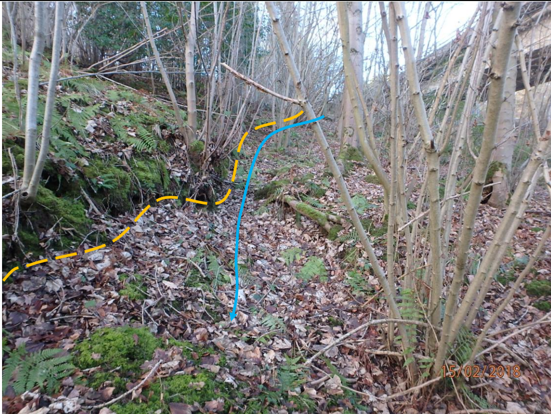
Photograph 20 – Example of the eastern lateral flank of the zone of instability to the west of the existing A1 bridge (yellow line). The lateral extent is marked by the location of a dry drainage channel (blue line).
