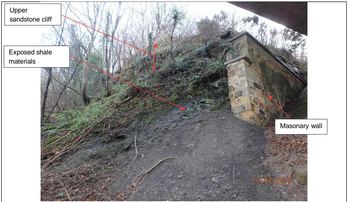
Photograph 1 – View south-east to the sandstone escarpment at the top of the slope.
