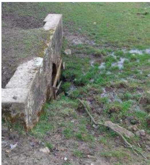
Figure 5-3 – Shieldhill Burn Downstream of Culvert
