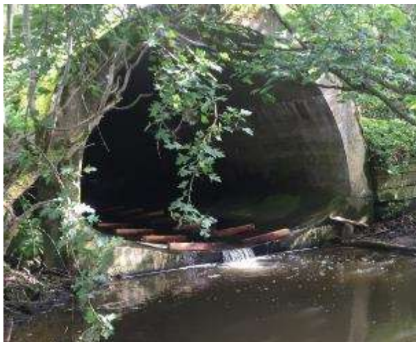
Figure 10-1 - Burgham Culvert, Outlet
