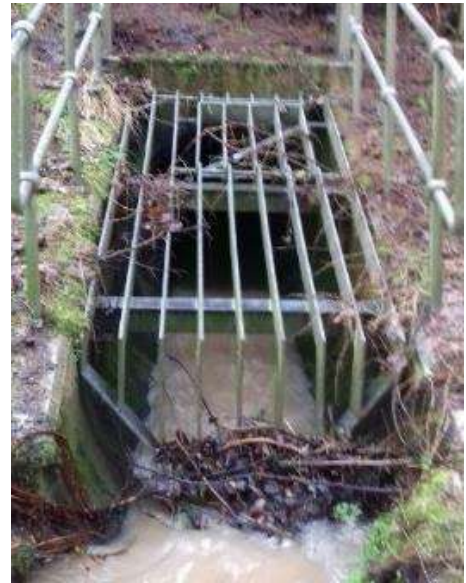
Figure 13-2 - Bradley Brook Culvert, Inlet
