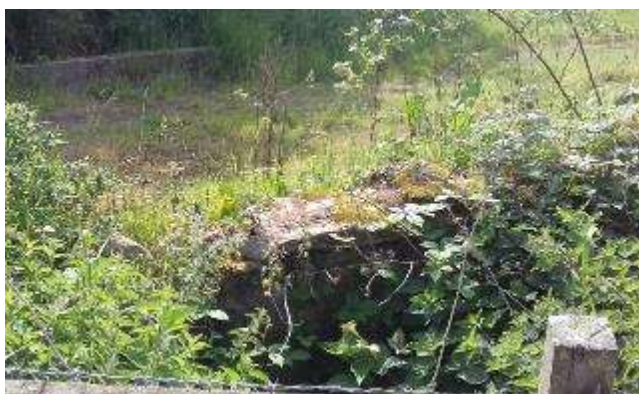
Figure 4-6 - Cotting Burn Crossing (Upstream)
