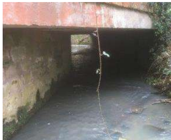
Figure 9-3 - Earsdon Burn Crossing (2)
