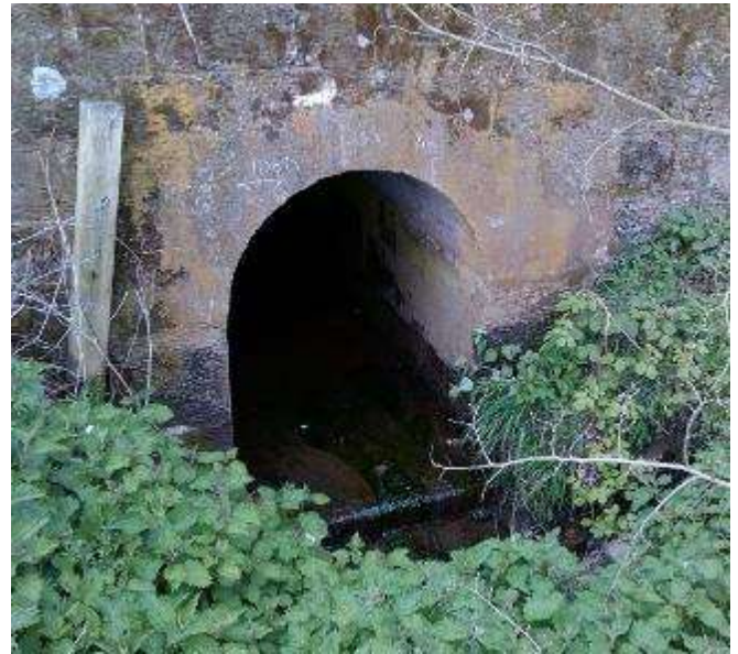
Figure 5-2 - Shieldhill Burn Culvert, Downstream
