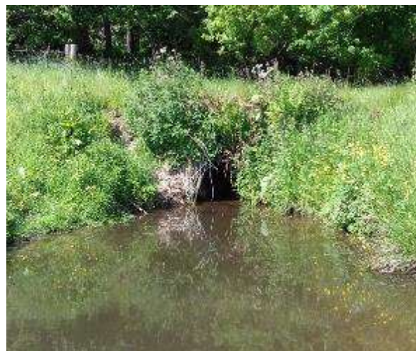
Figure 6-2 - Floodgate Burn Culvert Underneath Farm Access Track, Downstream
