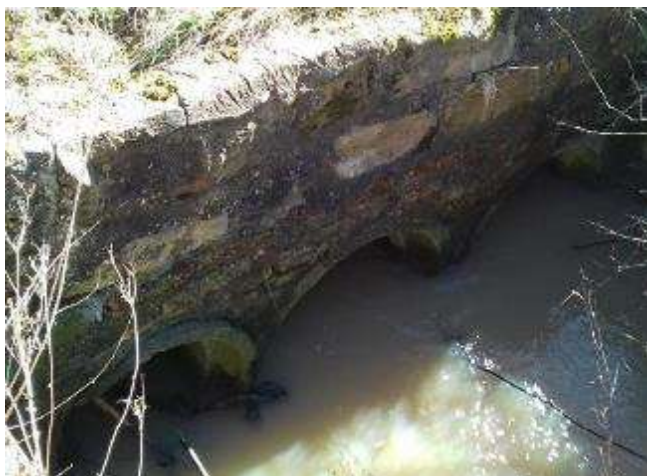
Figure 9-2 - Earsdon Burn Culvert (1)
