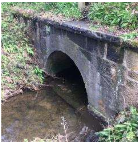
Figure 6-1 - Floodgate Burn Culvert Underneath the A1, Downstream
