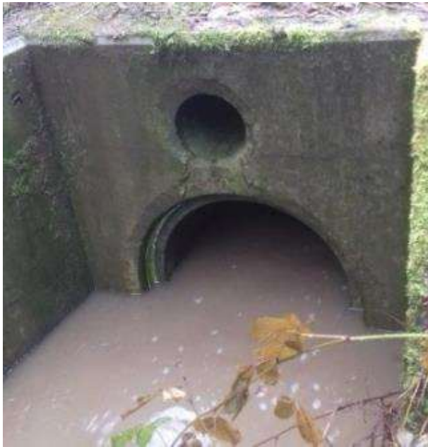
Figure 13-1 - Bradley Brook Culvert, Outlet
