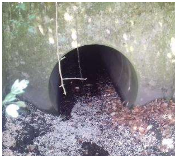
Figure 4-3 - Outlet of Cotting Burn Culvert (2)
