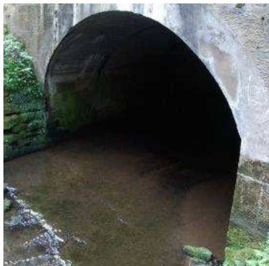
Figure 7-2 - River Lyne Culvert, Downstream
