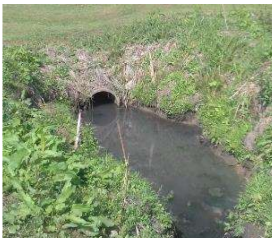
Figure 4-4 - Outlet of Cotting Burn Culvert (3)
