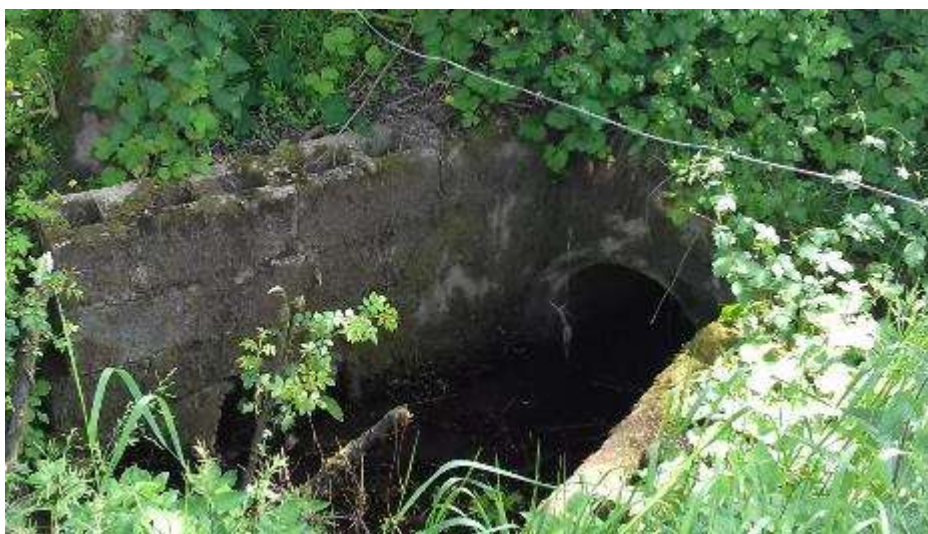
Figure 8-1 – Fenrother Burn Culvert, Upstream
