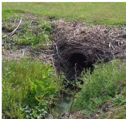
Figure 4-5 - Inlet of Cotting Burn Culvert (4)
