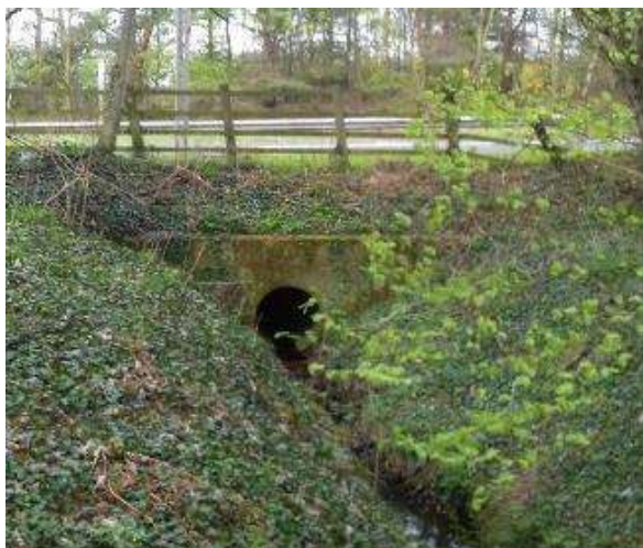
Figure 4-2 - Outlet of Cotting Burn culvert (1)
