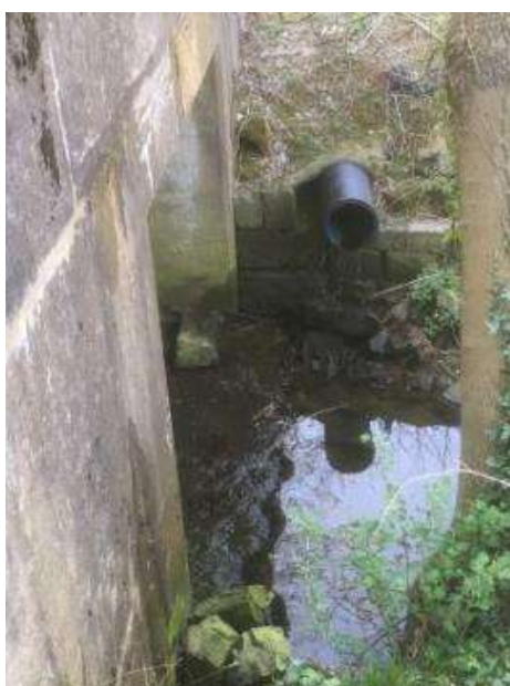
Figure 9-4 - Earsdon Burn Culvert (3)
