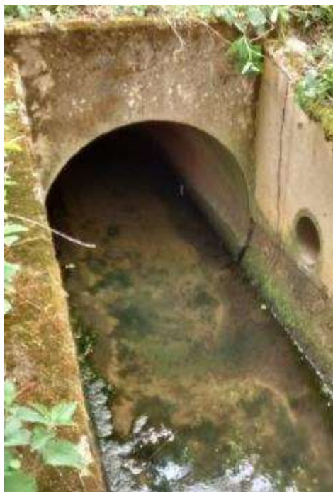
Figure 11-1 - Unnamed Tributary of Thirston Burn Culvert
