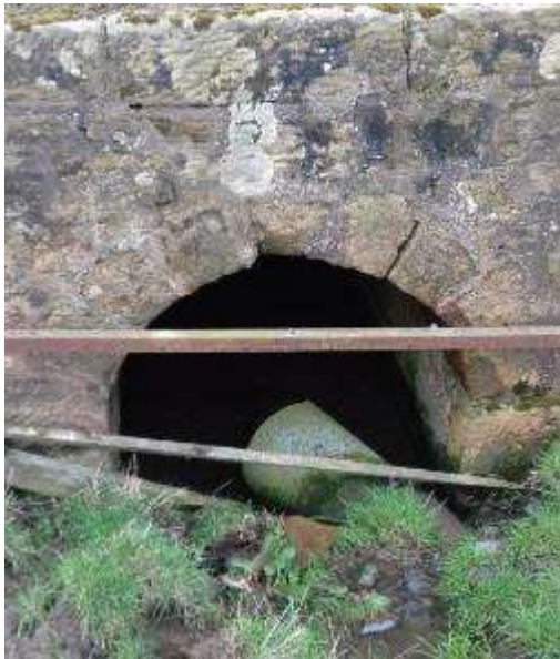
Figure 5-1 - Shieldhill Burn Culvert, Upstream
