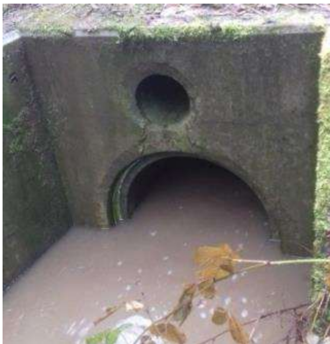
Figure 23 – Bradley Brook Culvert, Outlet
