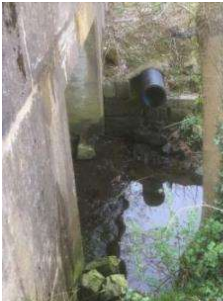
Figure 18 – Earsdon Burn Crossing (3)
