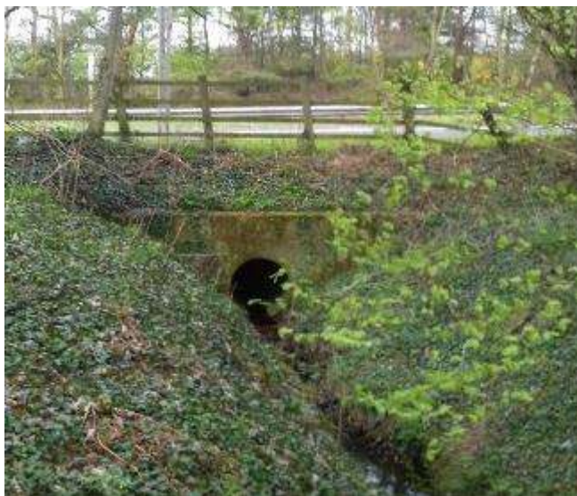
Figure 3 – Outlet of Cotting Burn Culvert (1)
