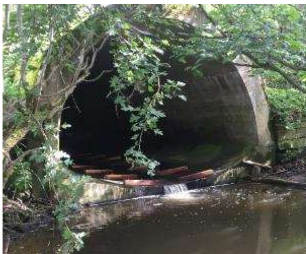
Figure 19 – Longdike Burn Culvert, Outlet
