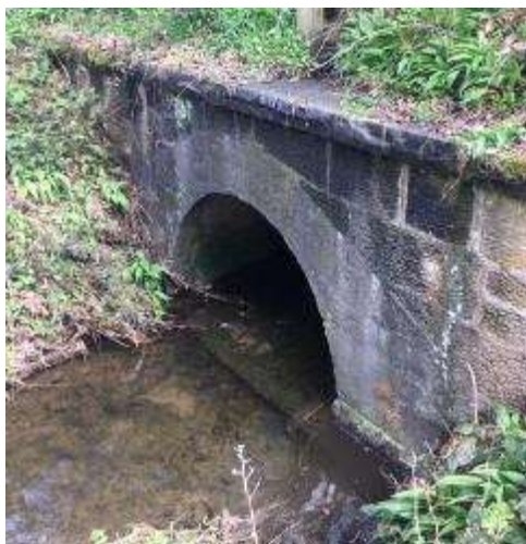
Figure 10 – Floodgate Burn Culvert Beneath the A1, Downstream
