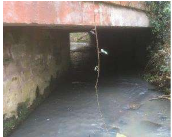
Figure 17 – Earsdon Burn Crossing (2)
