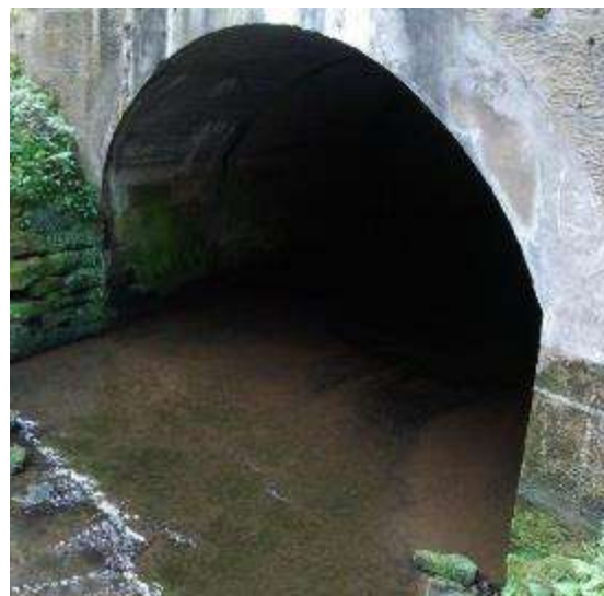
Figure 13 – River Lyne Culvert, Downstream
