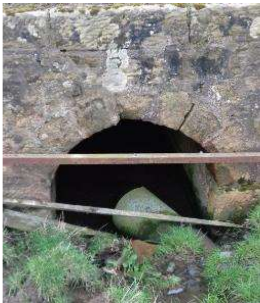
Figure 8 – Shieldhill Burn culvert, Upstream
