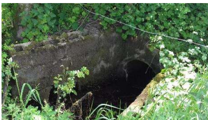
Figure 14 - Fenrother Burn Culvert, Upstream
