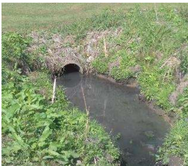
Figure 5 – Outlet of Cotting Burn Culvert (3)
