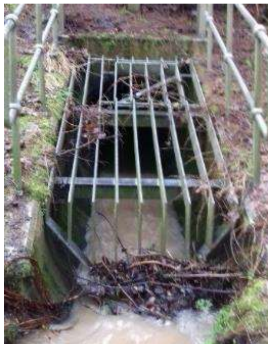
Figure 24 – Bradley Brook Culvert, Inlet
