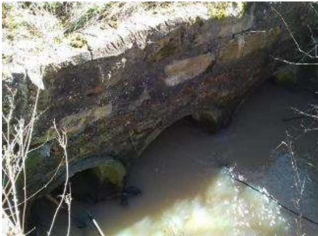
Figure 16 – Earsdon Burn Culvert (1)
