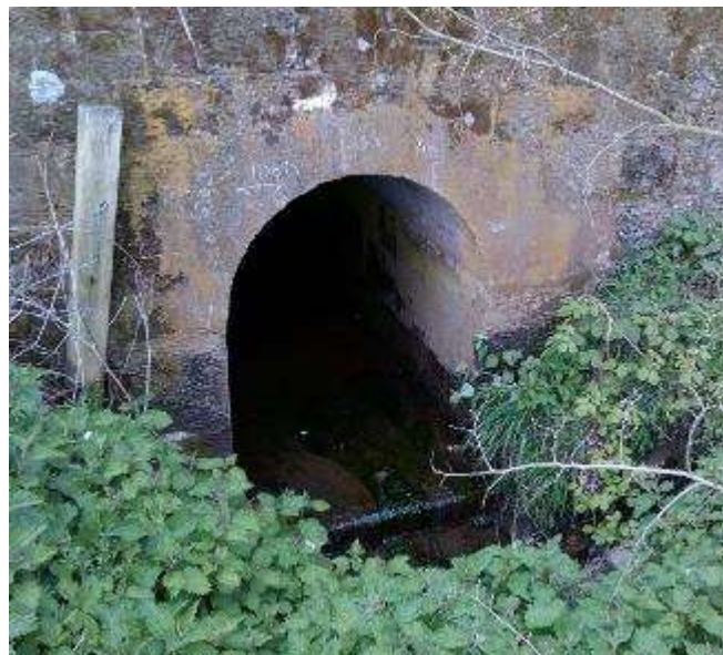
Figure 9 –Shieldhill Burn culvert, Downstream
