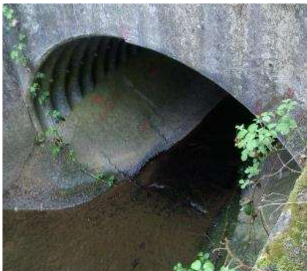
Figure 12 – River Lyne Culvert, Upstream
