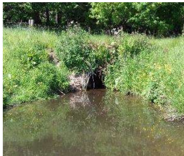
Figure 11 – Floodgate Burn Culvert Underneath Farm Access Track, Downstream
