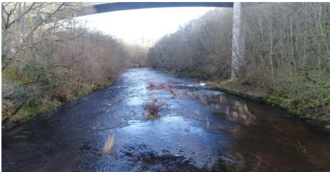
Figure 22 – River Coquet Bridge, Looking Downstream
