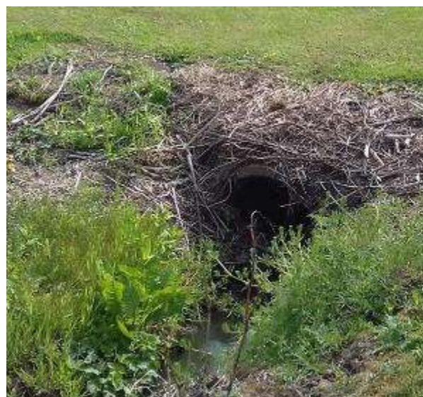
Figure 6 – Inlet of Cotting Burn Culvert (4)
