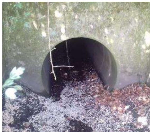
Figure 4 – Outlet of Cotting Burn Culvert (2)
