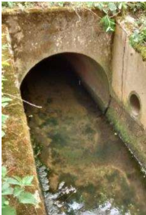
Figure 21 – Unnamed Tributary of Thirston Burn culvert
