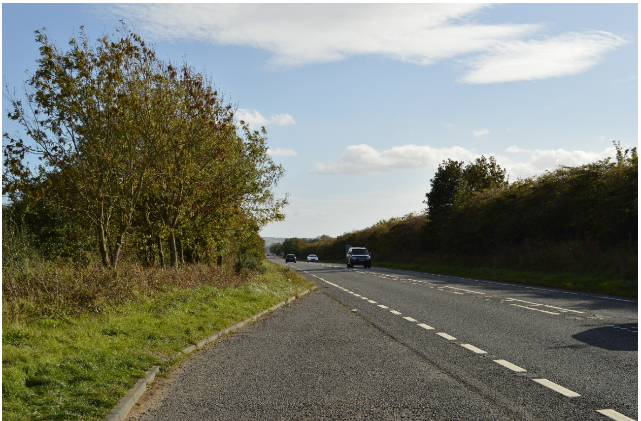
Figure 7.7 - View from Layby Looking to the South Along the A1
