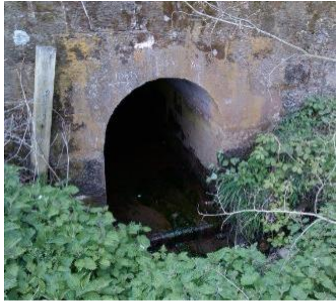
Image 10-9 - Shieldhill Burn Culvert, Downstream
