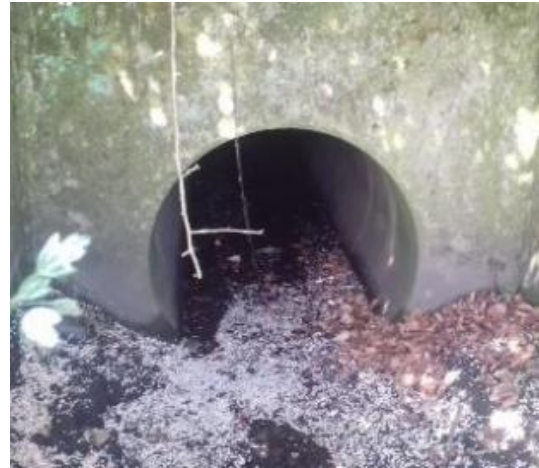
Image 10-3 - Outlet of Cotting Burn Culvert (2)
