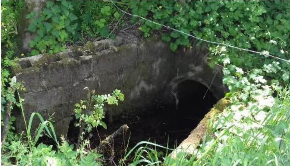
Image 10-17 - Fenrother Burn Culvert, Upstream
