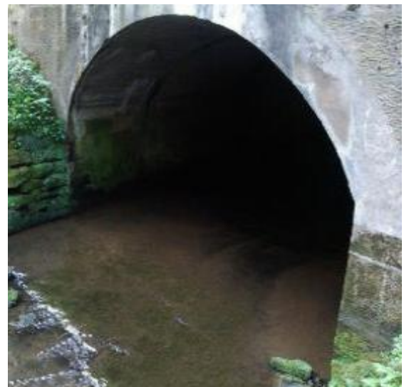
Image 10-15 - River Lyne Culvert, Downstream
