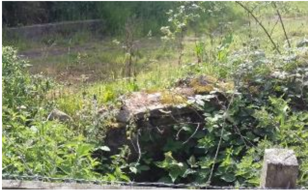
Image 10-6 - Cotting Burn Crossing (Upstream)
