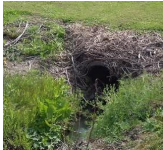
Image 10-5 - Inlet of Cotting Burn Culvert (4)
