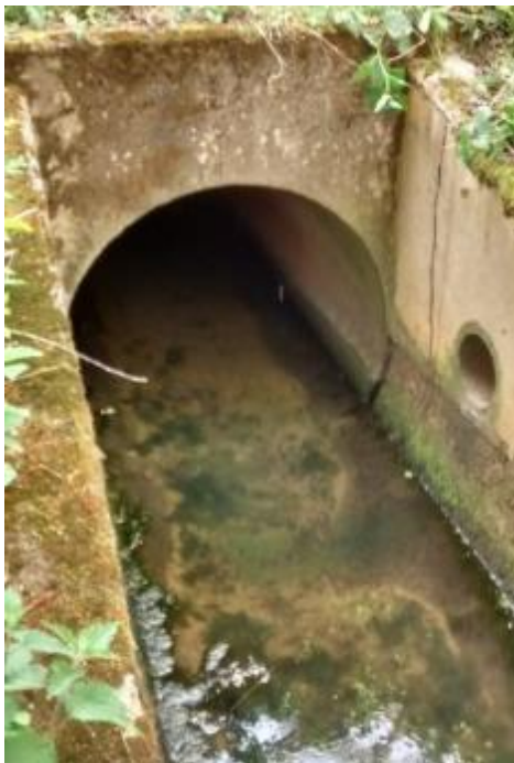
Image 10-27 - Unnamed Tributary of Thirston Burn Culvert
