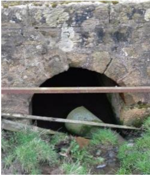
Image 10-8 - Shieldhill Burn Culvert, Upstream
