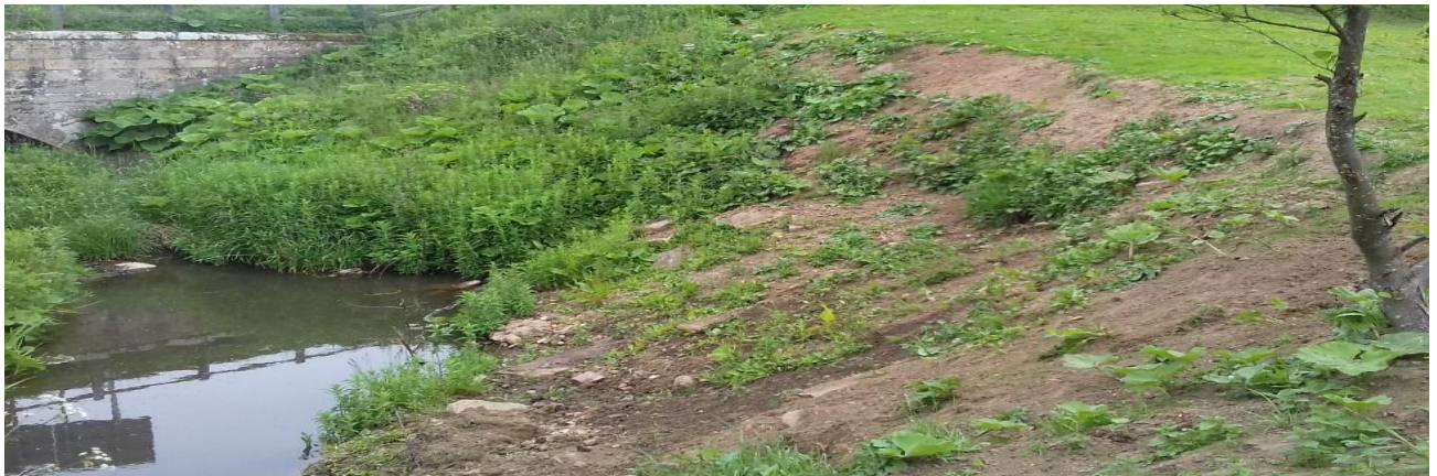
Image 10-25 – Evidence of Erosion along Longdike Burn
