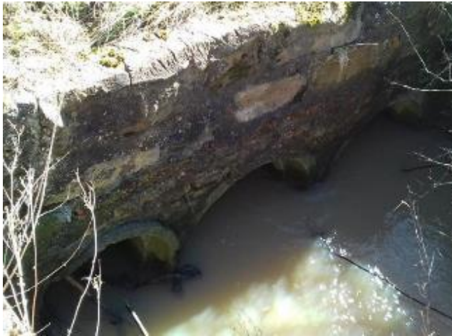
Image 10-19 - Earsdon Burn Culvert (1)
