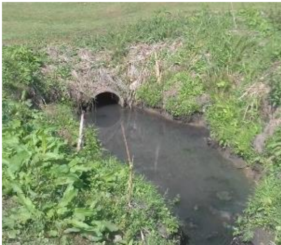
Image 10-4 - Outlet of Cotting Burn Culvert (3)
