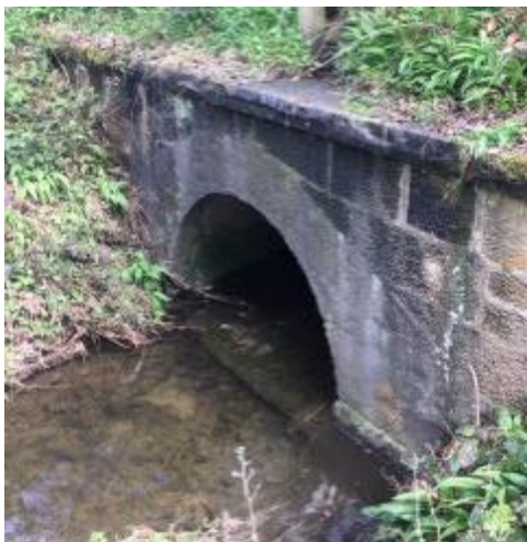
Image 10-11 - Floodgate Burn Culvert Underneath the A1, Downstream
