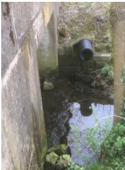
Image 10-21 - Earsdon Burn Culvert (3)
