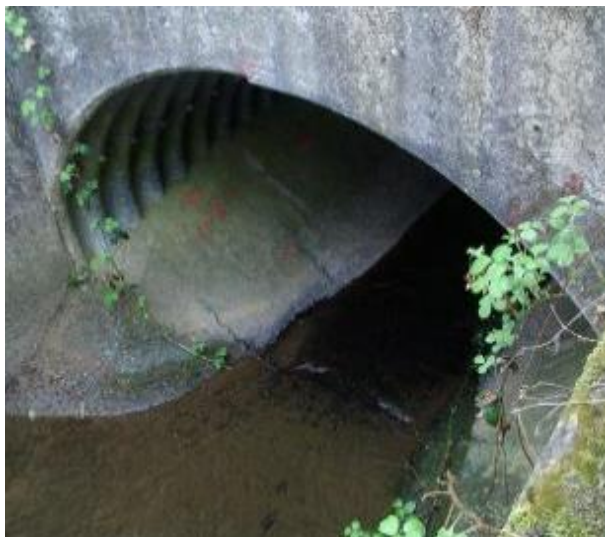
Image 10-14 - River Lyne Culvert, Upstream
