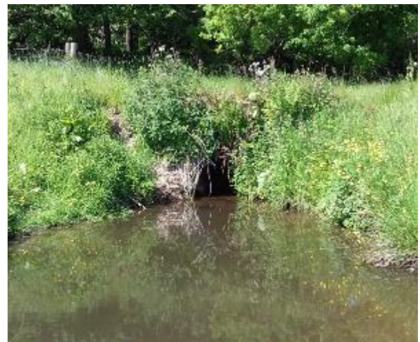
Image 10-12 - Floodgate Burn Culvert Underneath Farm access Track, Downstream
