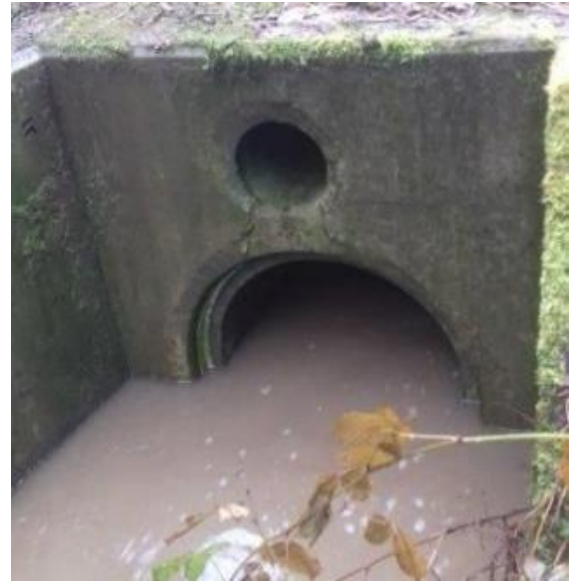
Image 10-32 - Bradley Brook Culvert, Outlet
