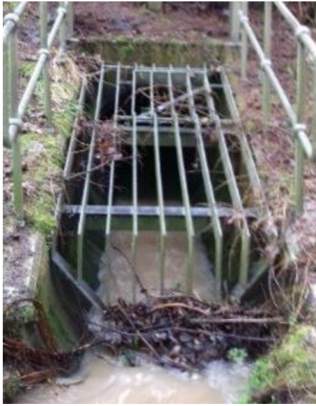
Image 10-31 - Bradley Brook Culvert, Inlet
