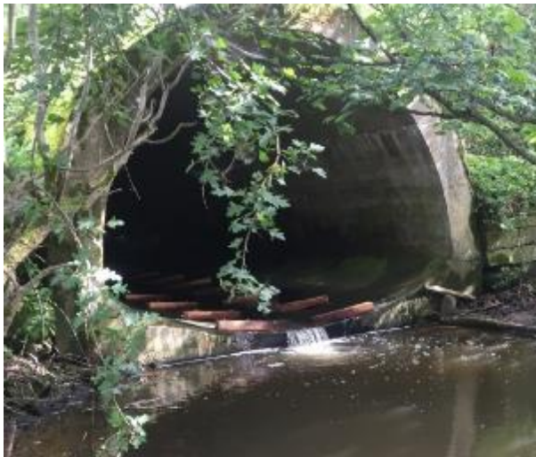
Image 10-23 - Burgham Culvert, Outlet
