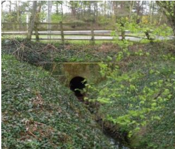
Image 10-2 - Outlet of Cotting Burn Culvert (1)
