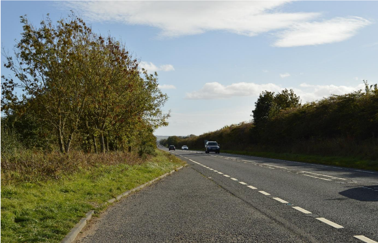
Figure 5-2 - View from the layby looking to the south along the A1
