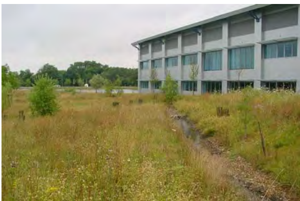
The use of ditches and wildflower meadows softens the impact of hi-tech office buildings at Granta Park.
