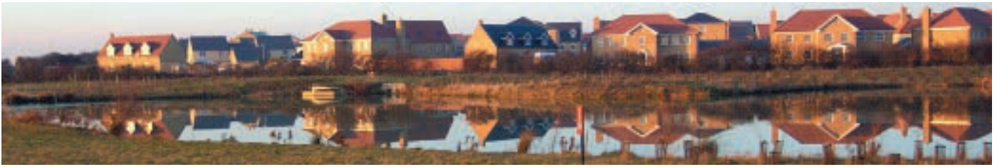
New housing at Cambourne by Caxton Bridleway 5
