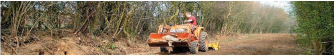
Byway improvements at Gypsy Lane Dullingham
