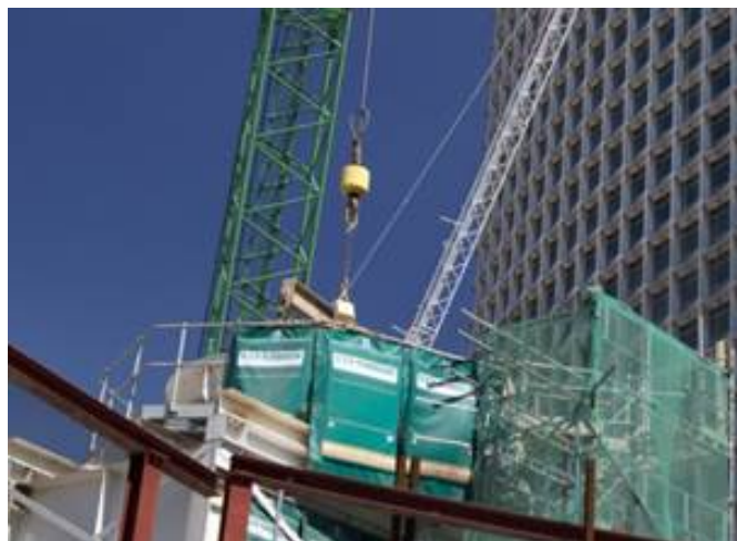
Figure 13.2 Localised screening for construction works - example 2
