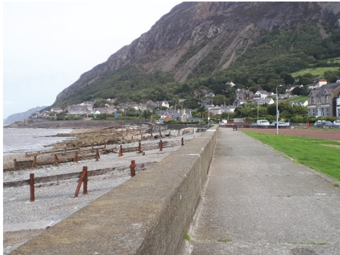
Plate 2- View Eastwards along Beach at Junction 15
