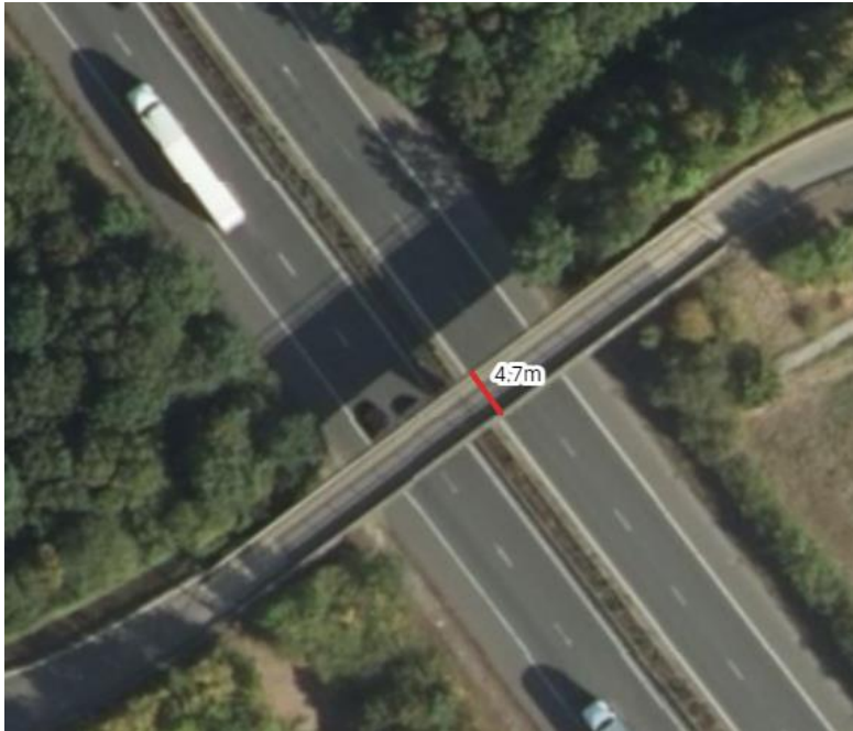
Figure 1 – M11 bridge (Cantelupe Farm)
