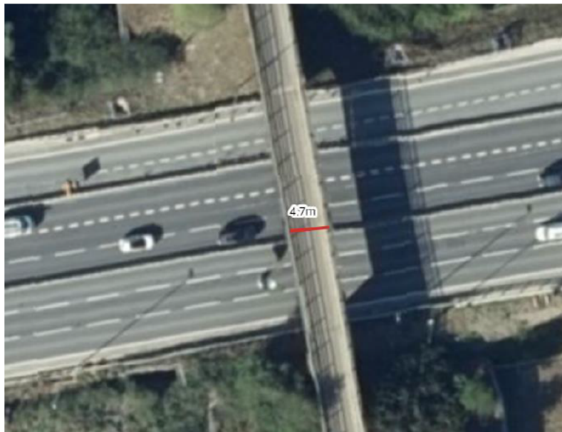
Figure 2 – A14 Bridge between Histon and Girton (Park Farm)
