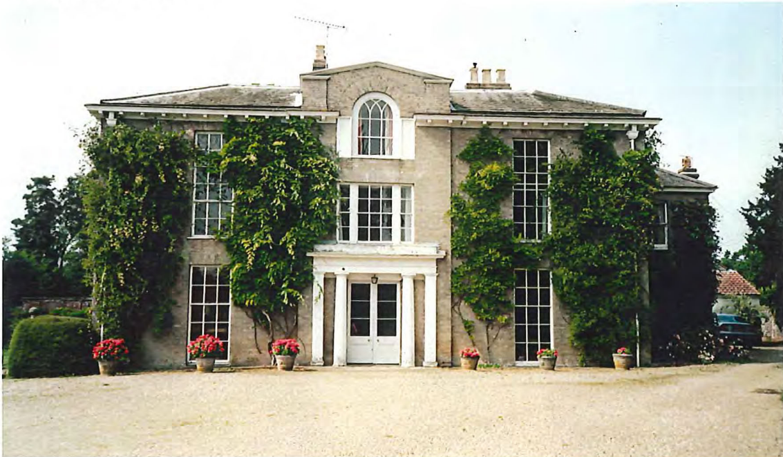
East elevation of Berry Hall
