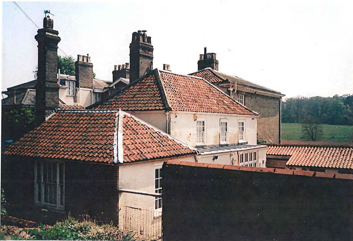
Berry Hall service range seen from the north west with the log store and garden shed to the right
