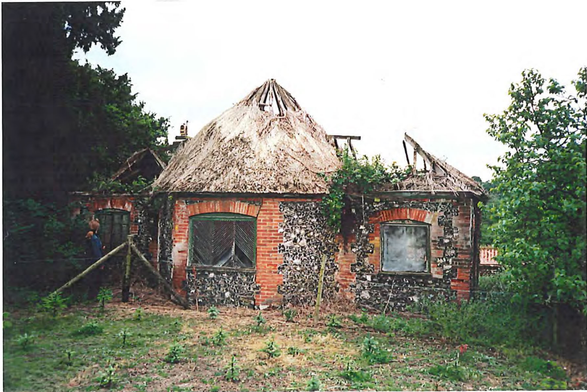
The Old Dairy seen from the north
