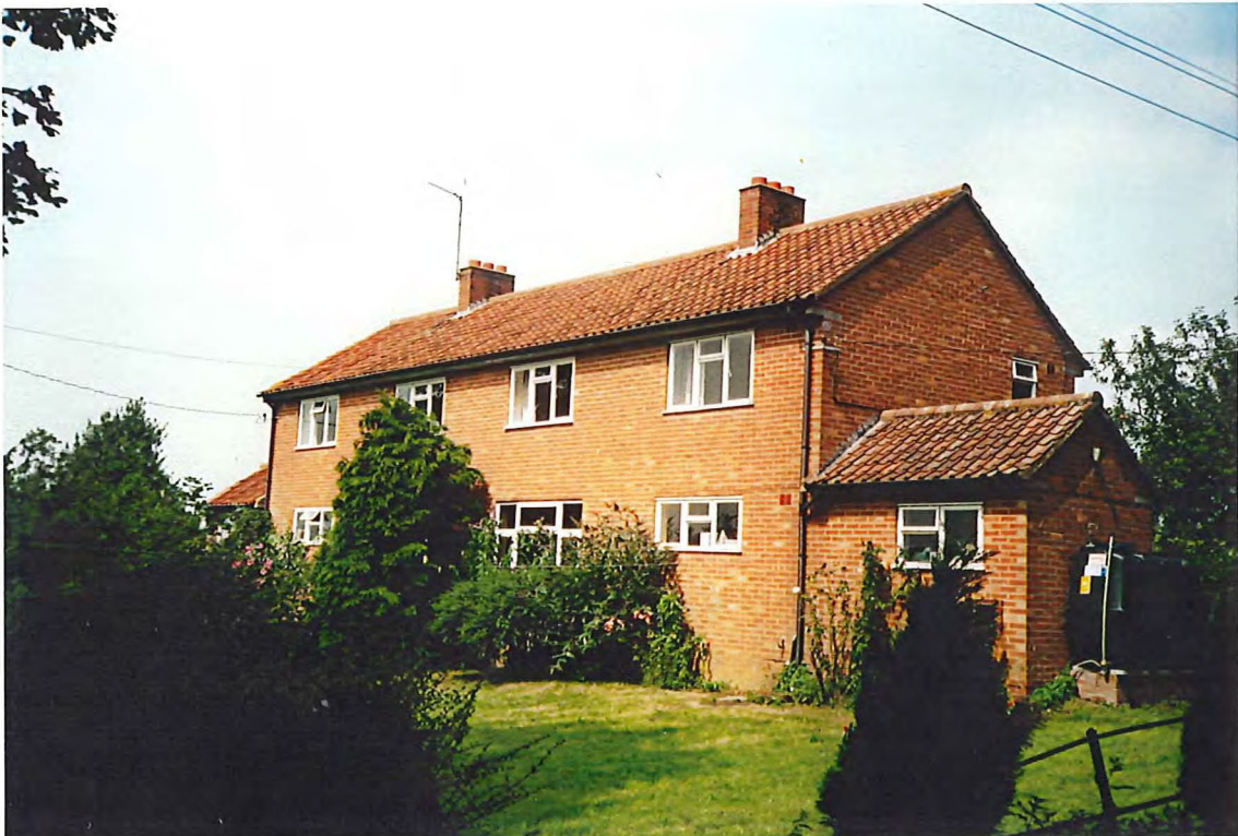
The semi-detached cottages seen from the south east
