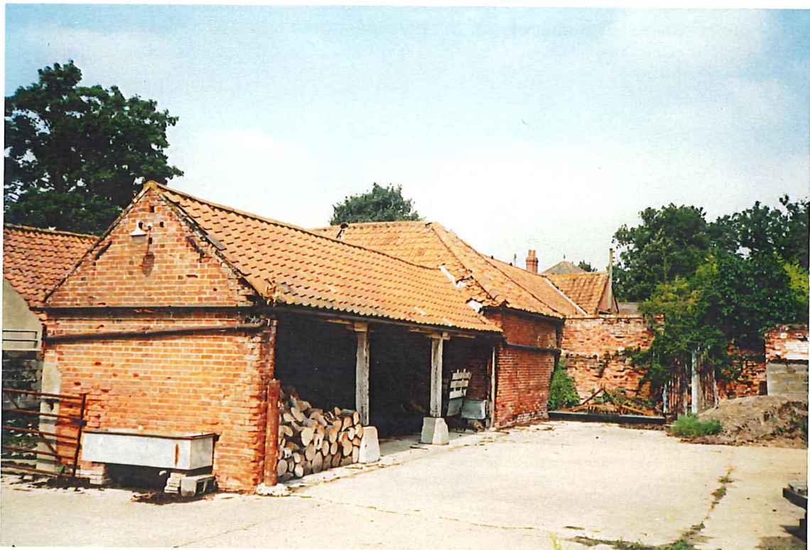
Range E seen from the south east
