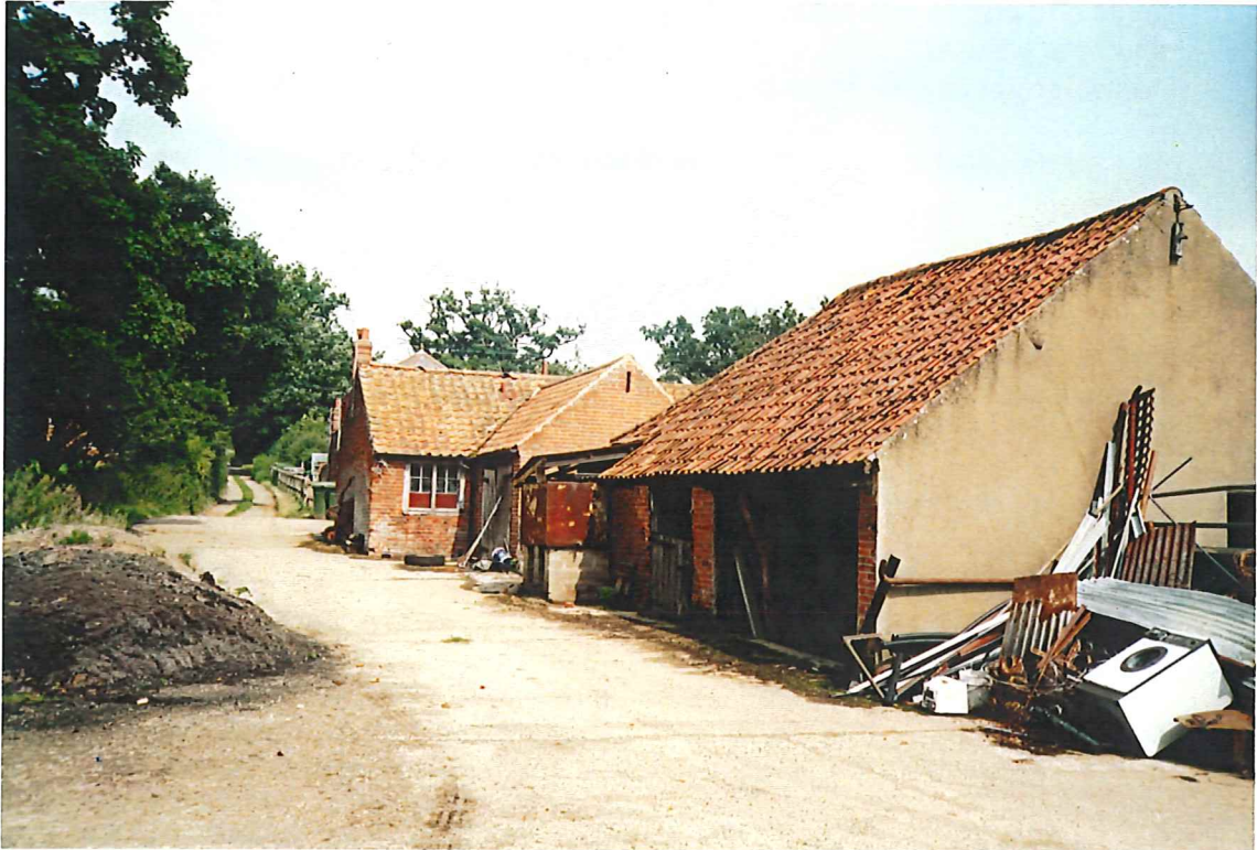
Range D seen from the south west with range A and B in the background
