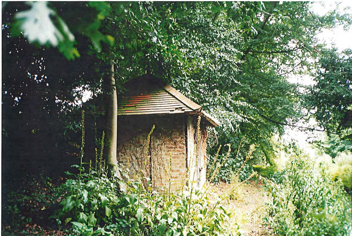
The Pump House seen from the west
