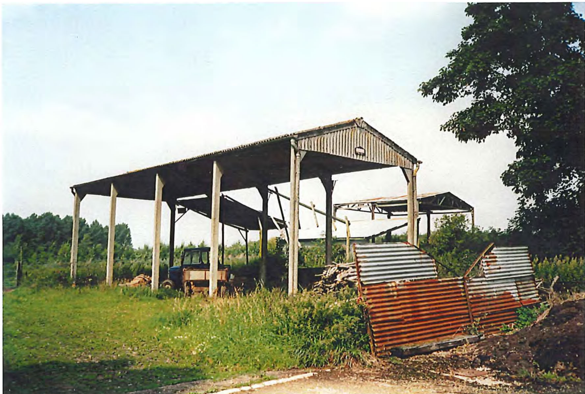
The Dutch Barns seen from the south east
