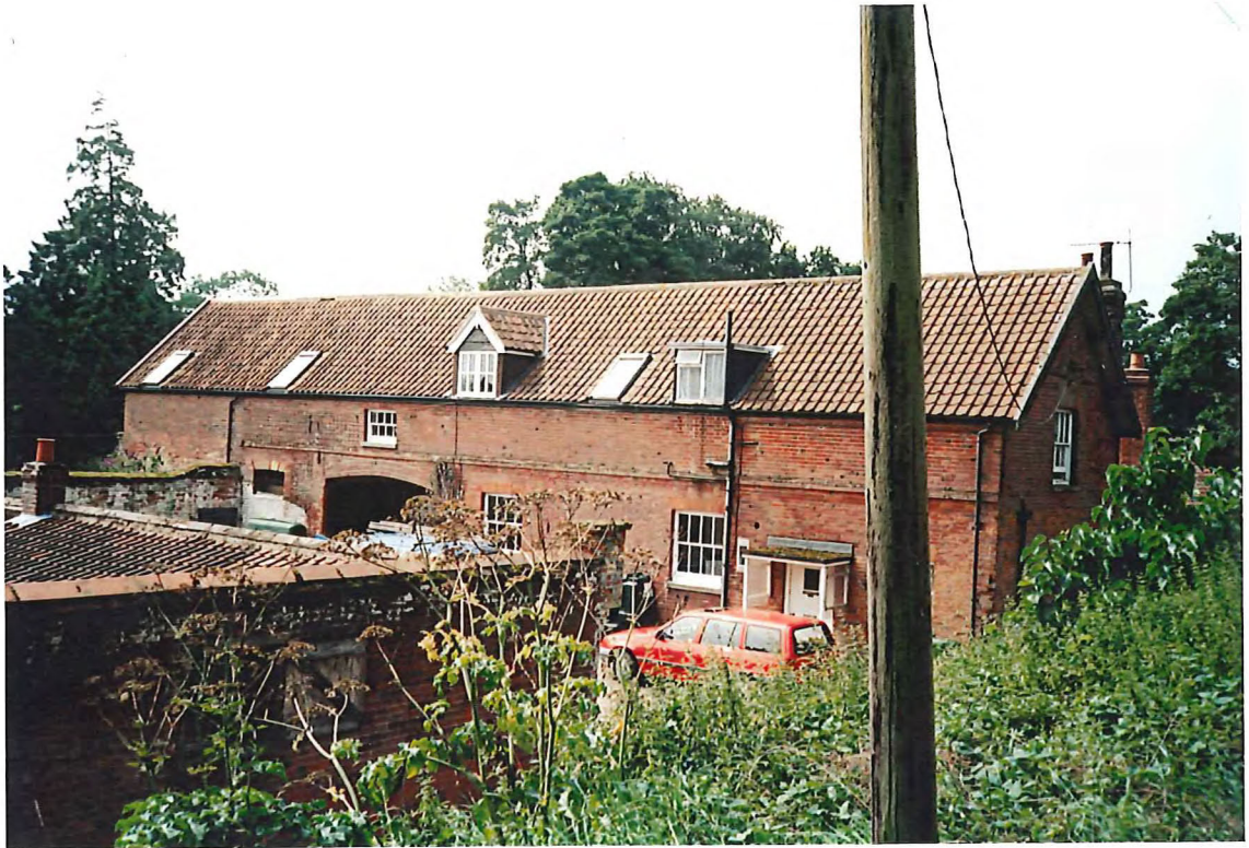
The east elevation Stables with Rosemary Cottage to the right seen from the north east
