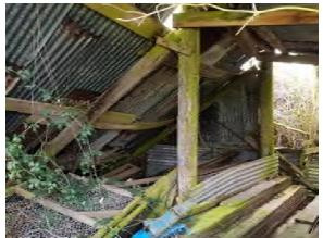
Photo 2. Collapsing wood storage shelter.
