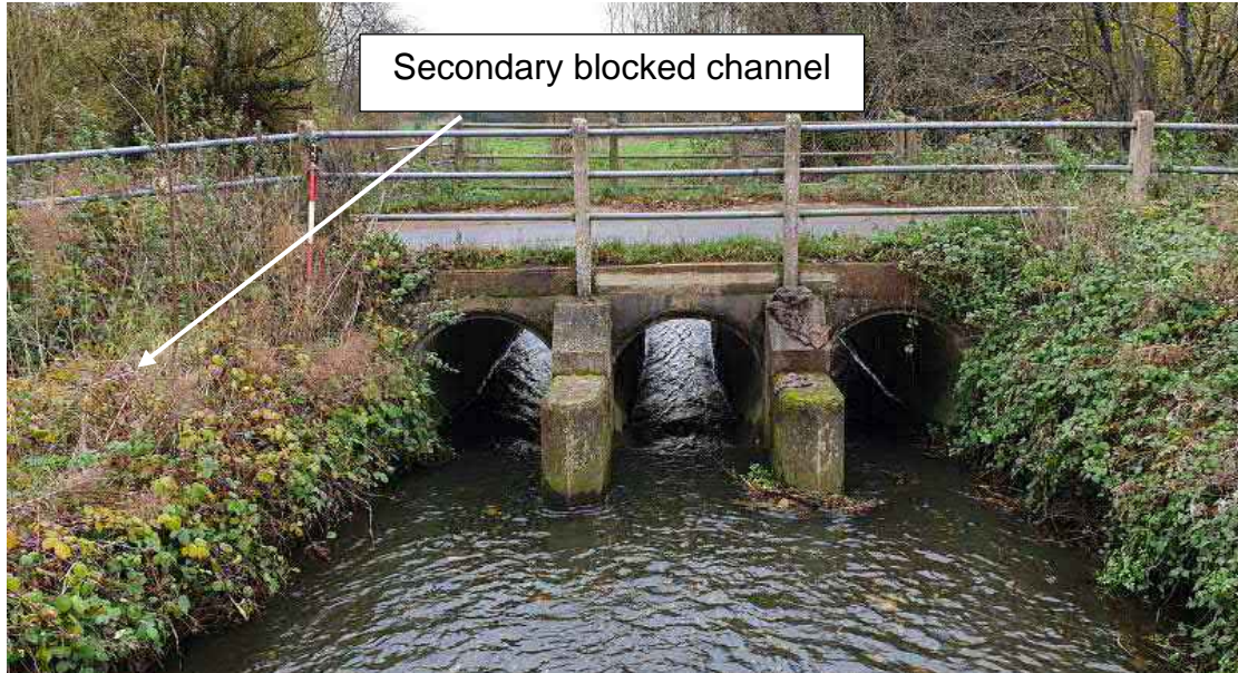
Figure 3-5 Three main culverts at Berry Lane Bridge
