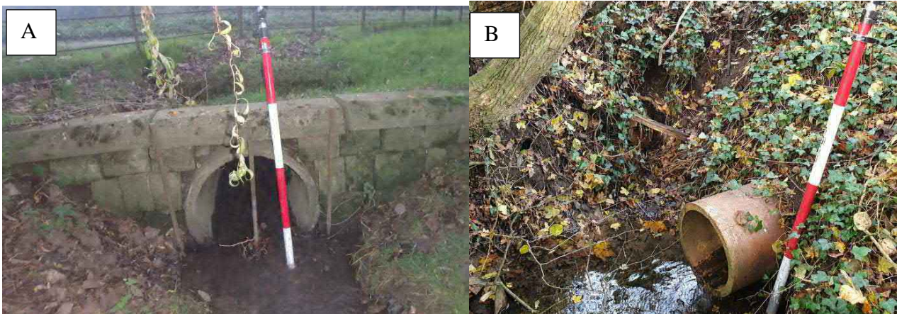
Figure 5-5 (A) Inlet and (B) outflow of the culvert under Low Road
