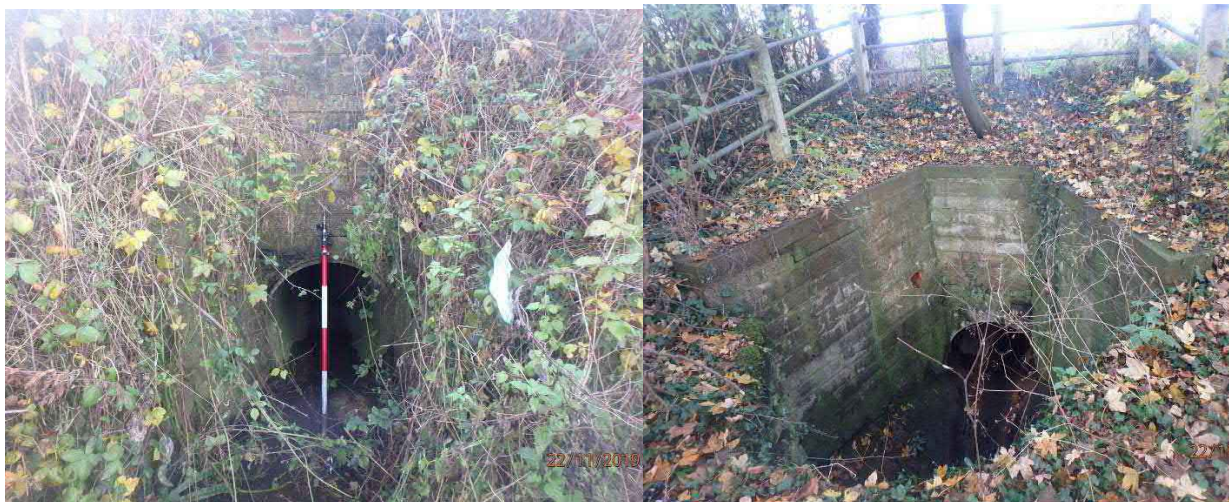
Figure 6-5 (A) Inlet to the culvert under the A47 and (B) open section between The Street and the A47
