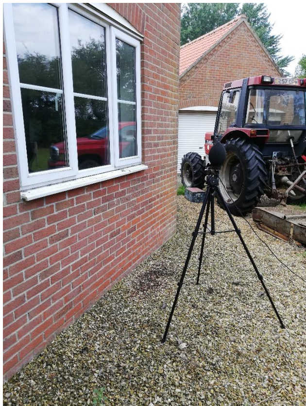
Figure 11.3.11: ST2 (façade measurement, from the south)
