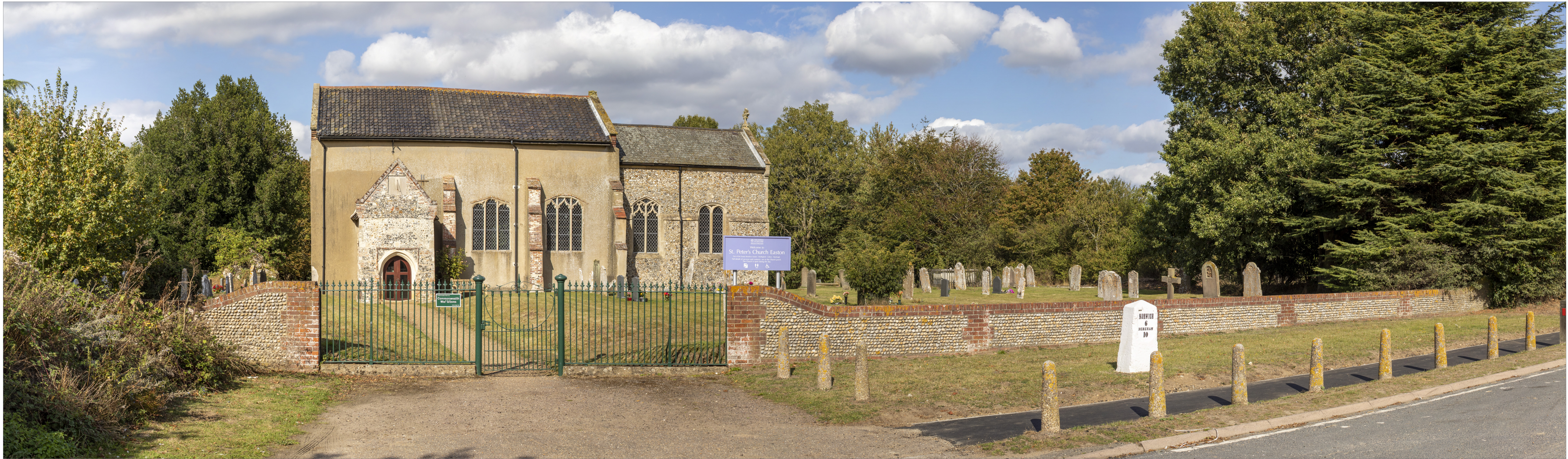
A47 North Tuddenham To Easton - Photomontages Figure 7.6.8B - Viewpoint 6: Existing View (Summer)
