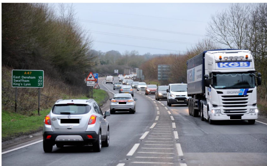
Caption: A view of the existing A47 between North Tuddenham and Easton
