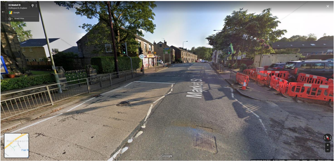
Figure 2.1 Existing pedestrian crossing on Market Street, Hollingworth which could be improved.
