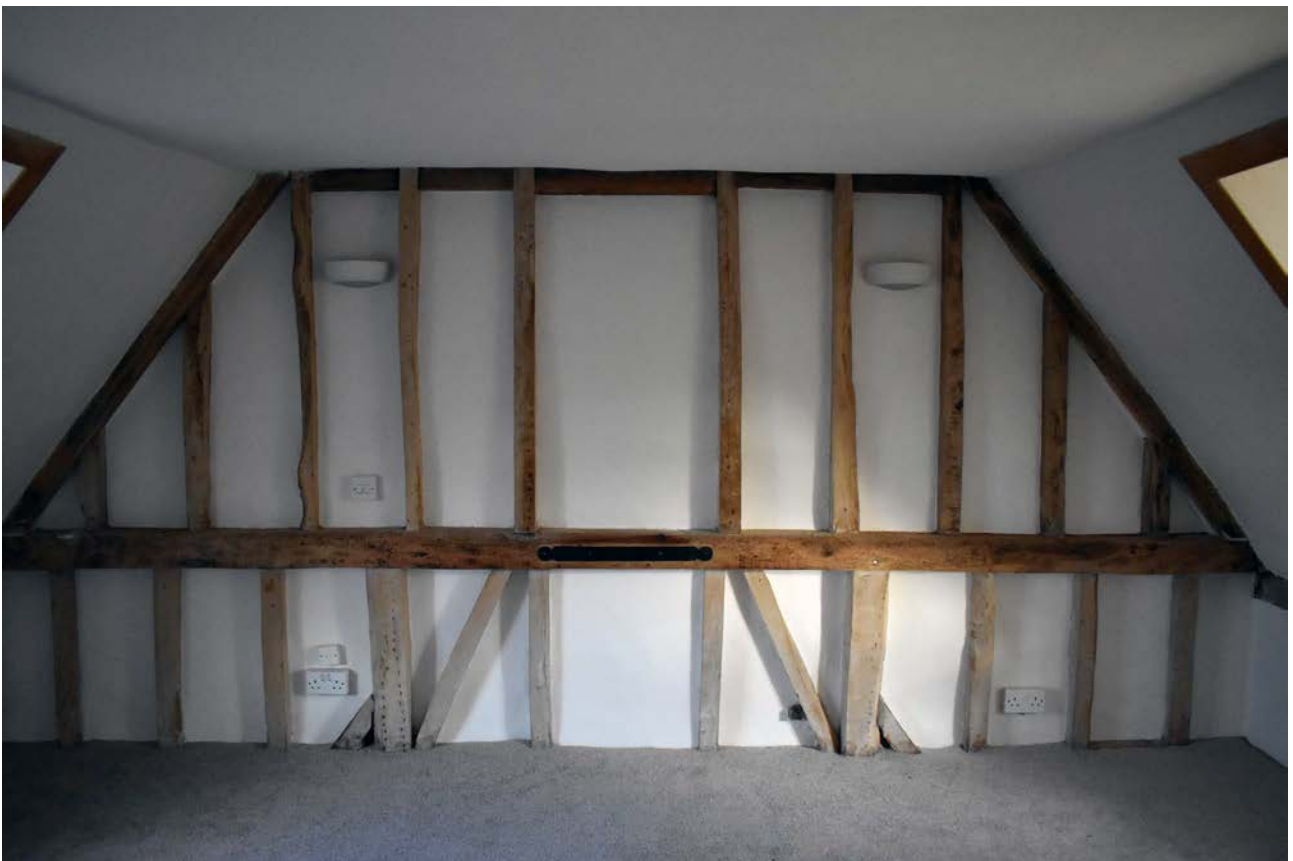
Plate 89: First floor, principal bedroom, east wall
