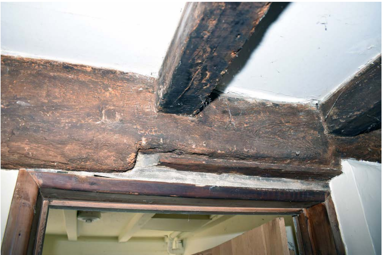
Plate 17: Principal joist in the hallway above the kitchen doorway
