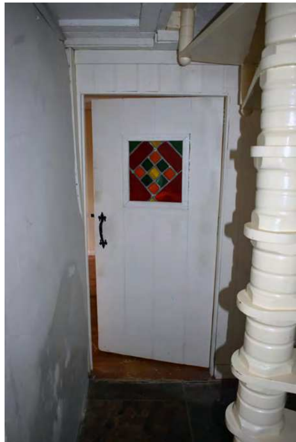
Plate 40: Ground floor, central bay, entrance to the north bay
