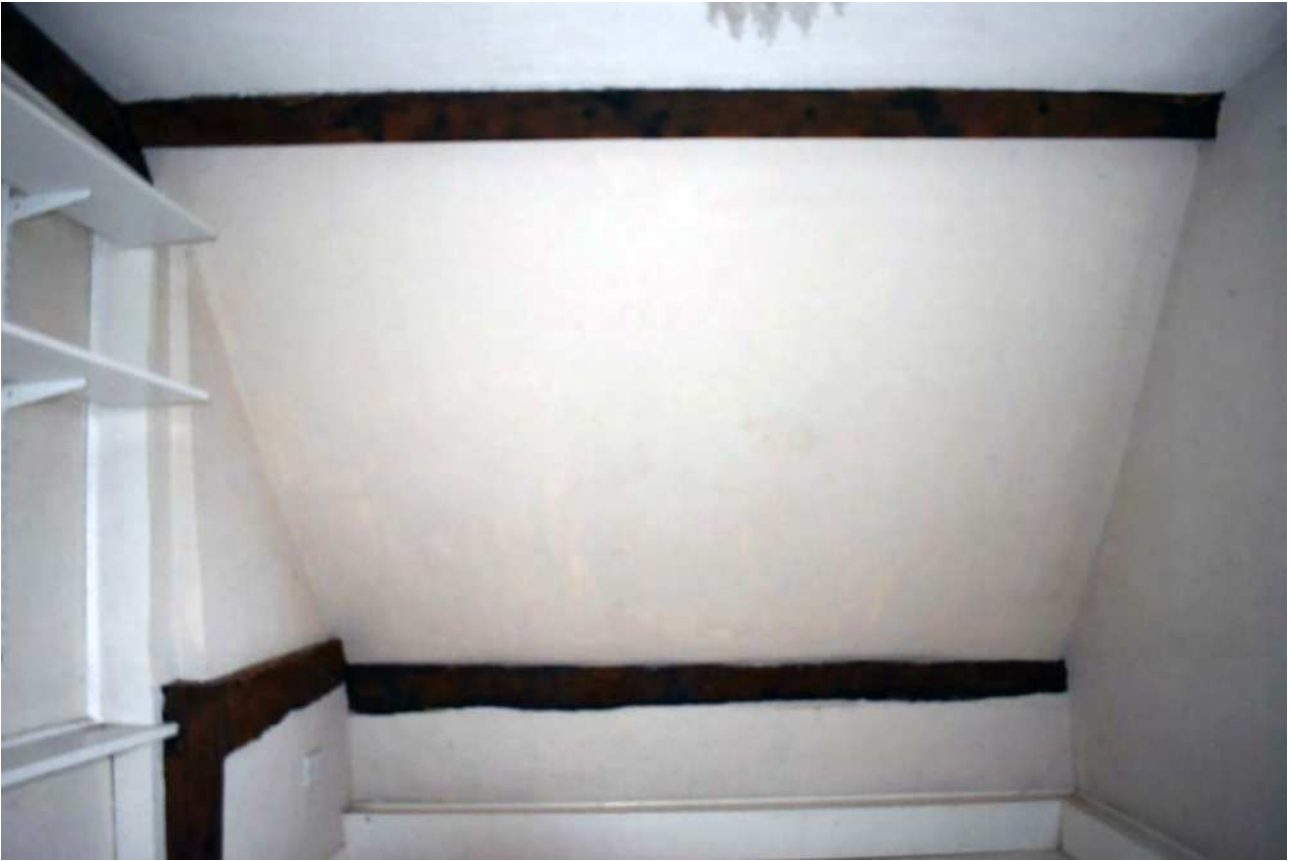
Plate 66: First floor, north bay, west wall
