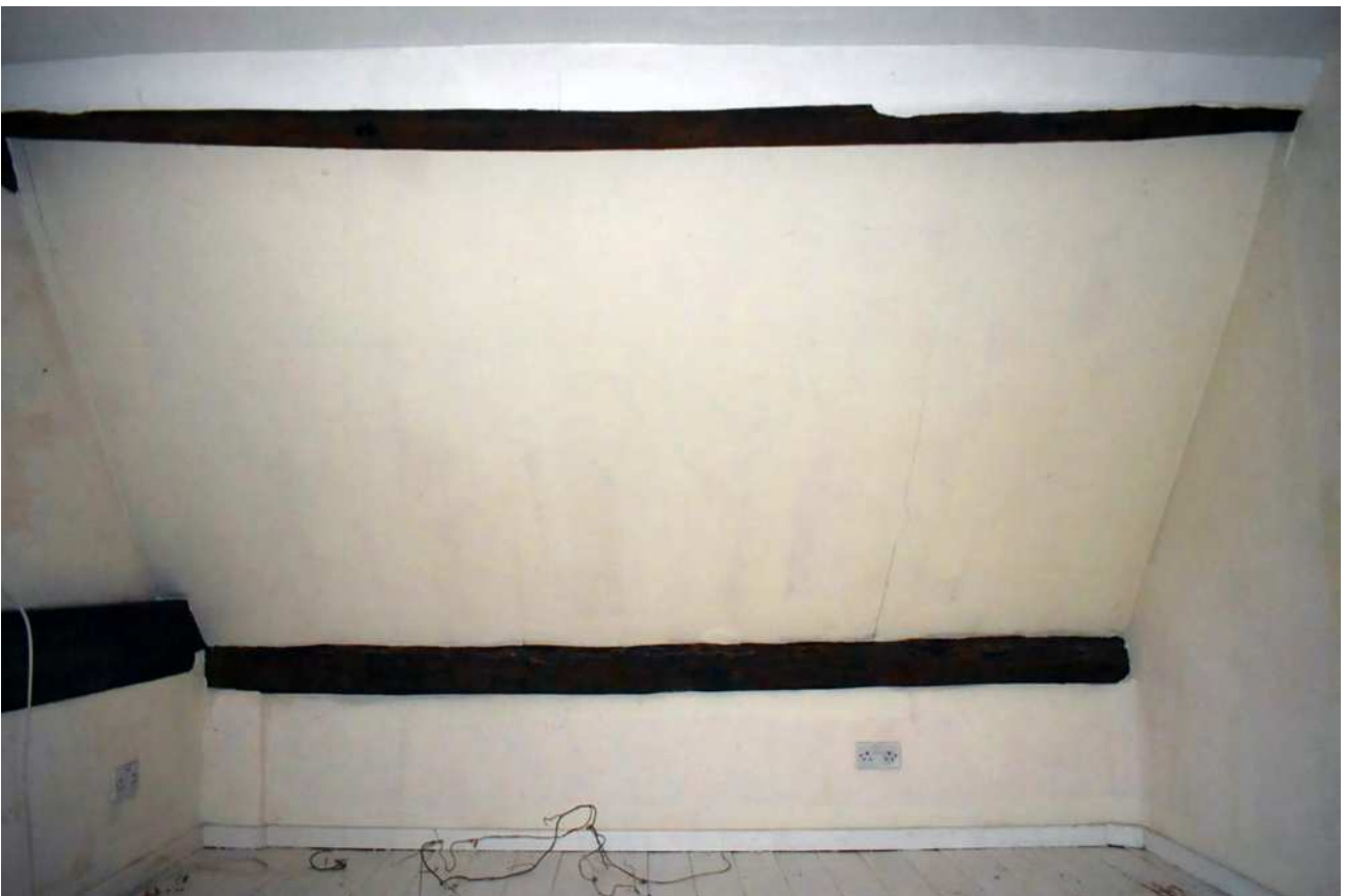
Plate 63: First floor, south bay, west wall
