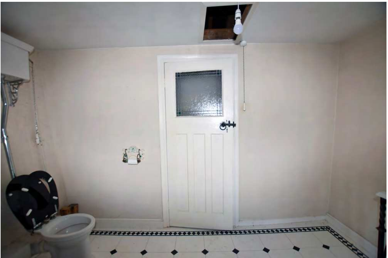
Plate 59: First floor, central bay, bathroom, east wall
