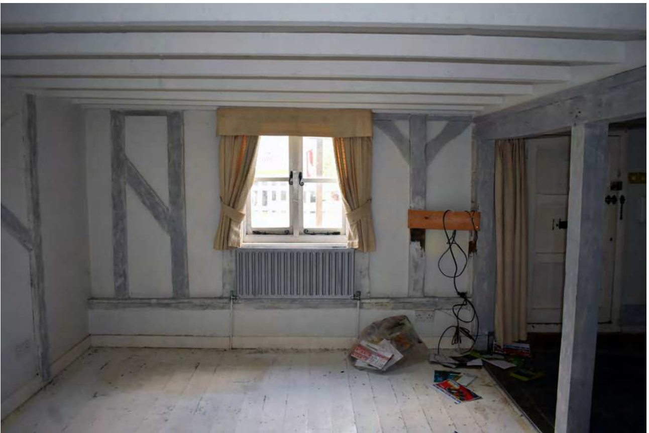
Plate 34: Ground floor, south bay, west wall
