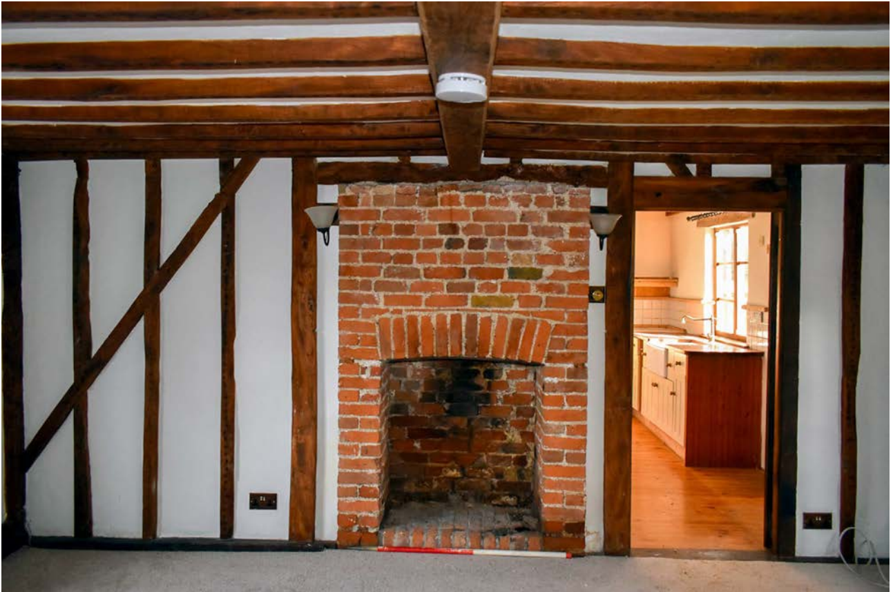
Plate 68: Ground floor, living room, east wall with chimney
