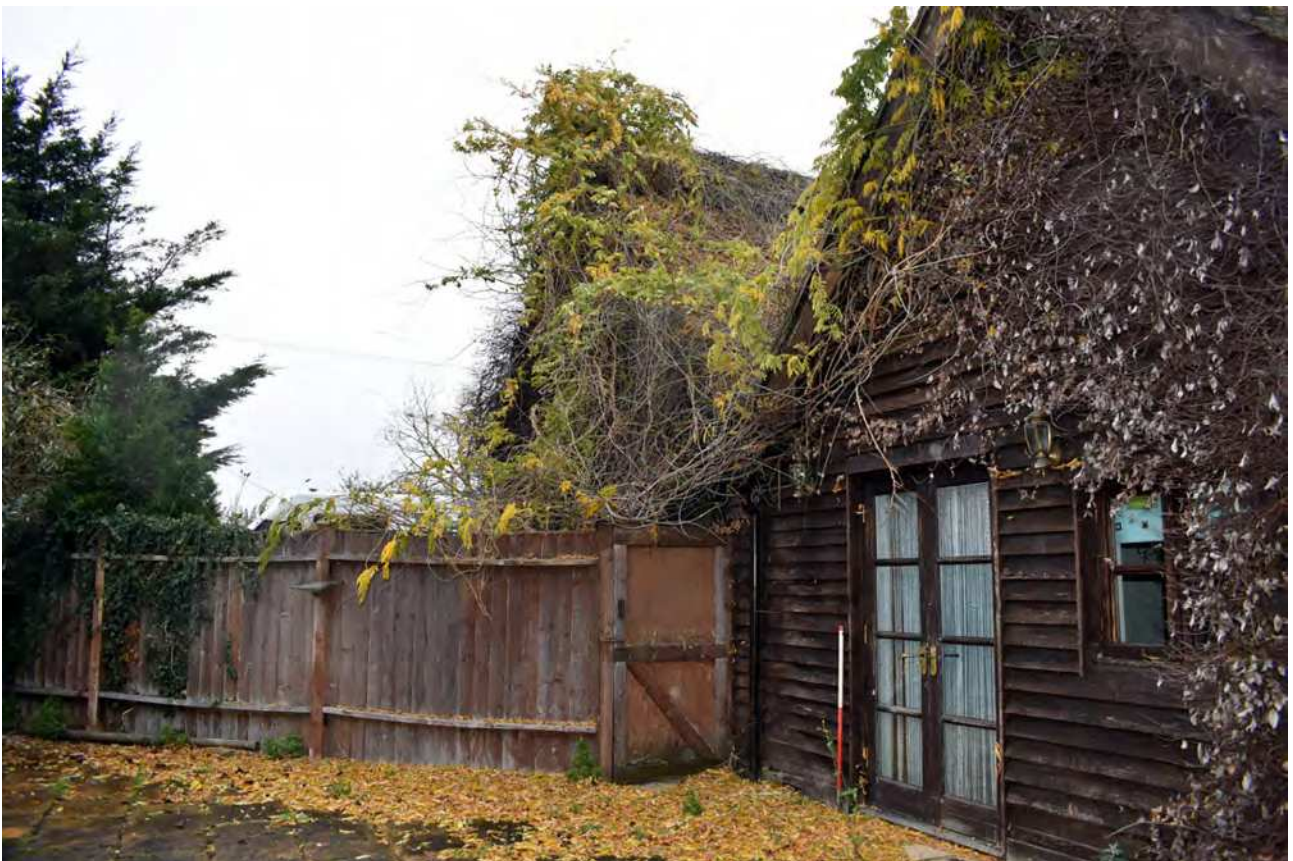
Plate 14: South elevation, fence between the cottage and the extension
