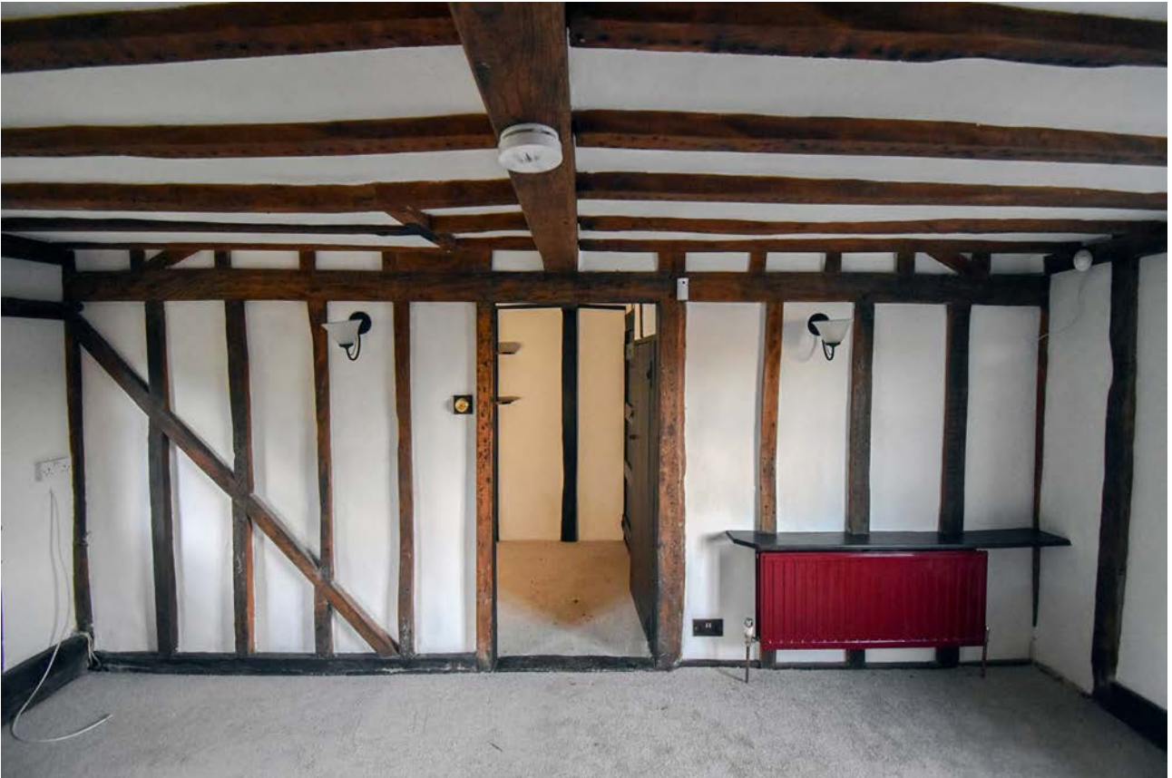
Plate 72: Ground floor, living room, west wall
