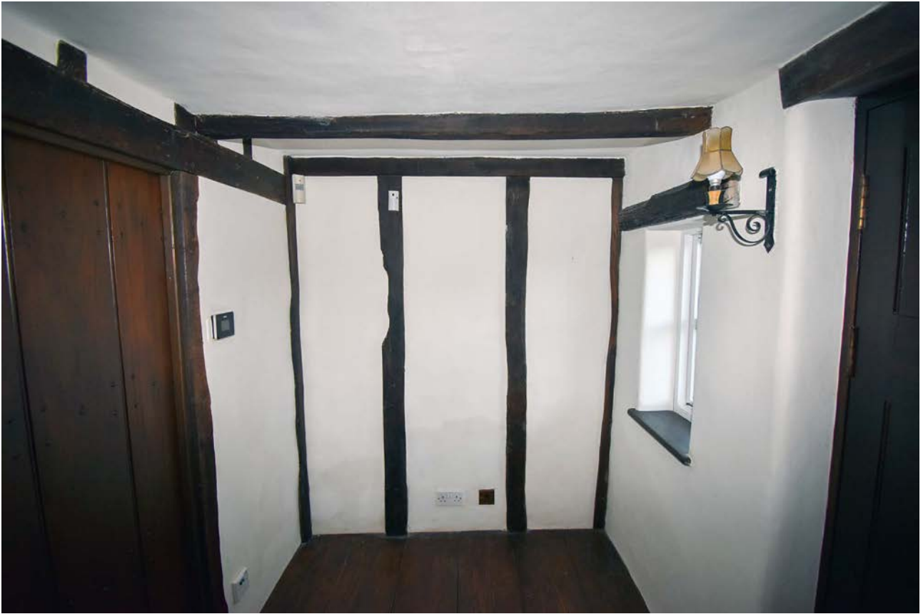
Plate 58: Ground floor, entrance hall, west wall
