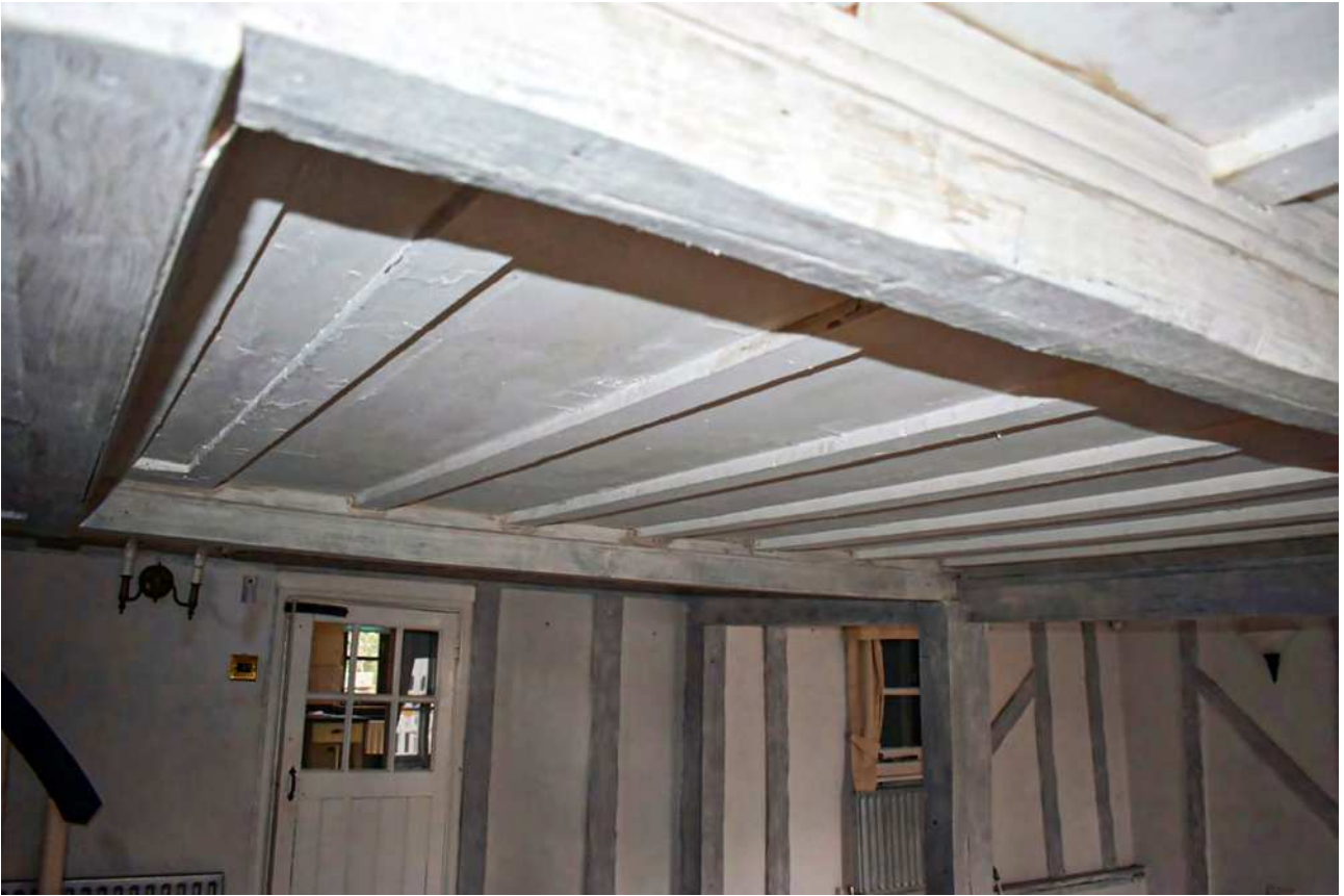
Plate 41: Ground floor, central bay, ceiling beams
