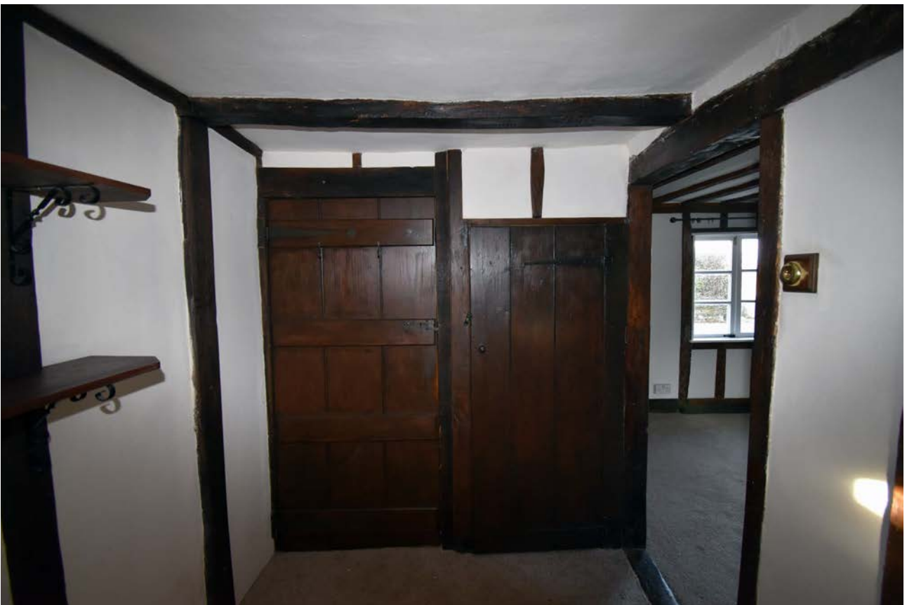
Plate 65: Ground floor, lobby, north wall
