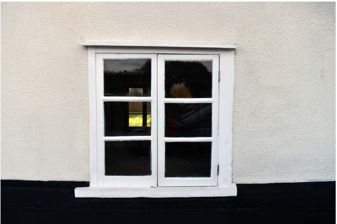
Plate 38: North elevation, window with casement with two two-pane lights
