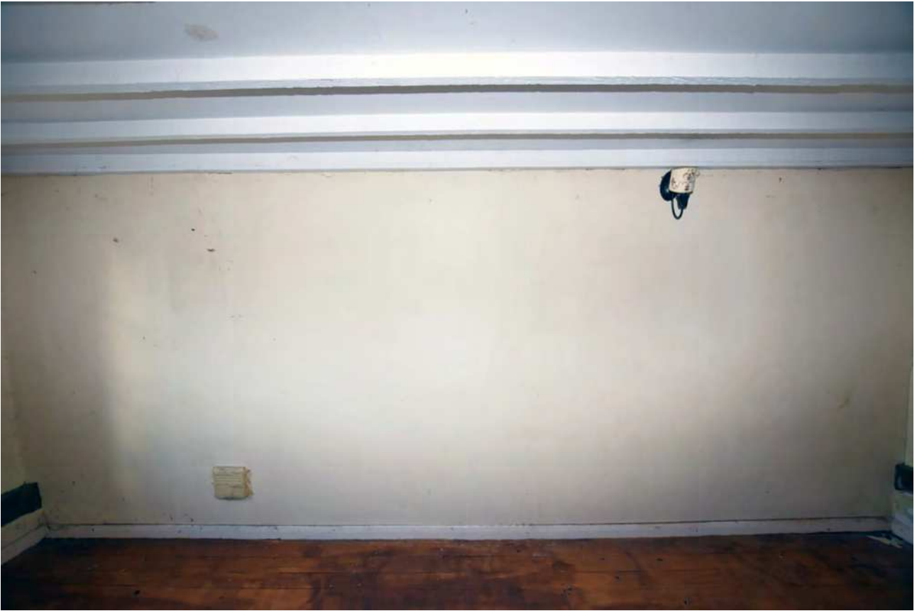
Plate 48: Ground floor, north bay, north wall
