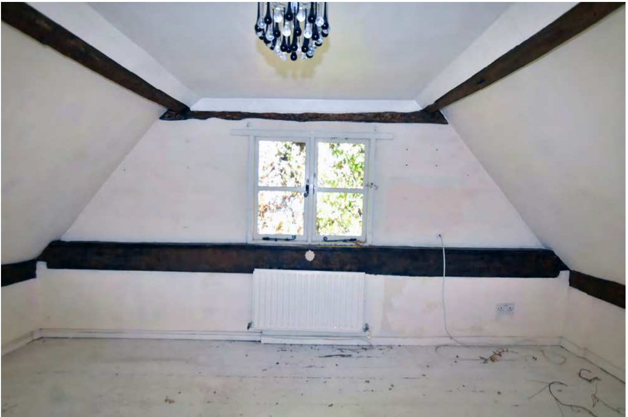
Plate 64: First floor, south bay, south wall
