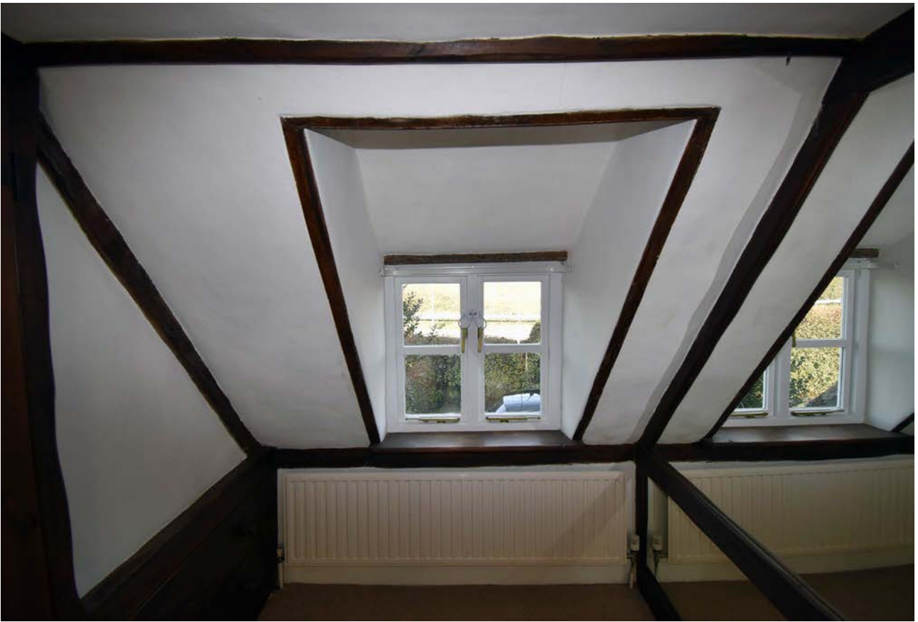
Plate 94: First floor, wardrobe, north wall
