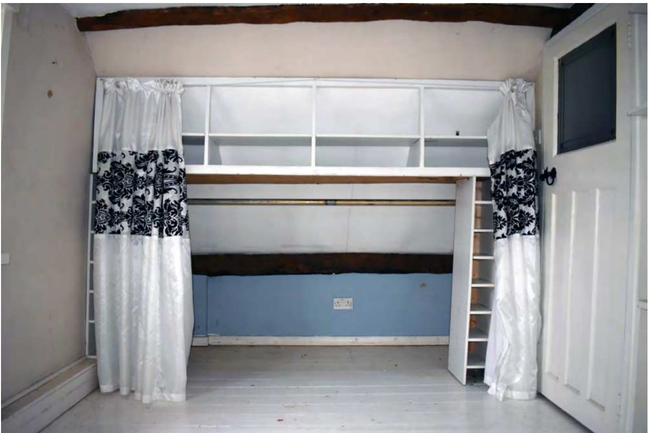
Plate 65: First floor, north bay, east wall
