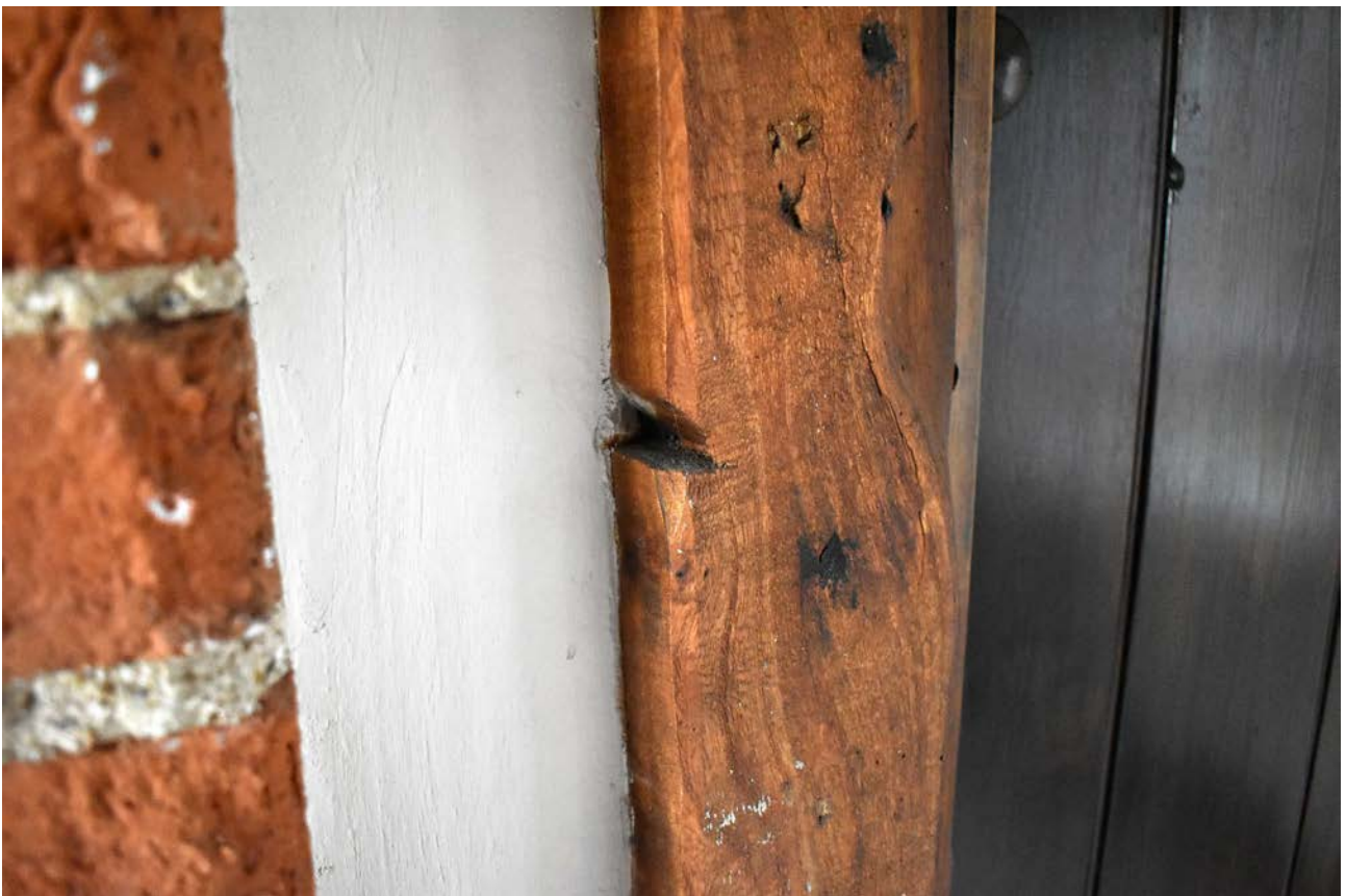
Plate 69: Ground floor, living room, east wall, hole for the fireplace casing
