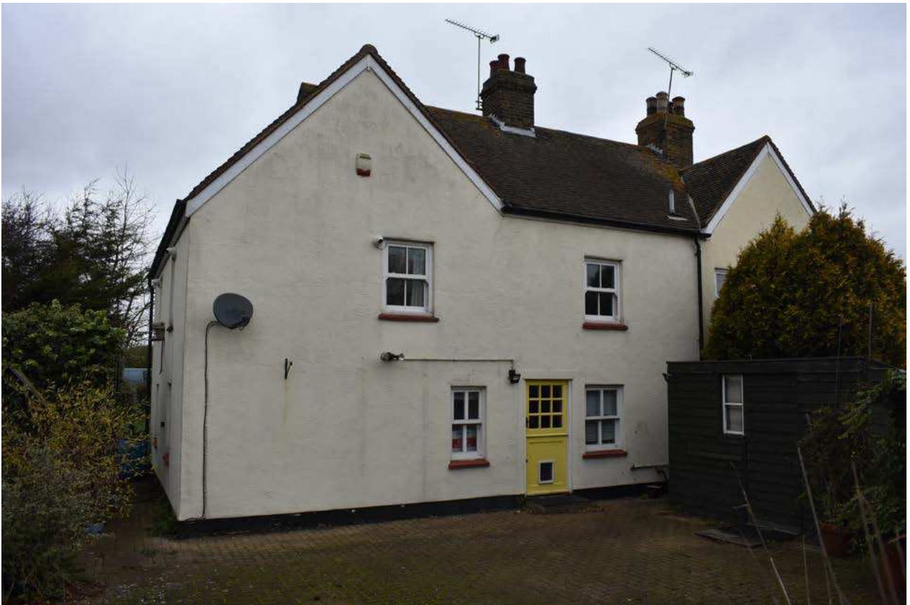
Plate 4: The south elevation of No. 2 Grays Corner Cottages
