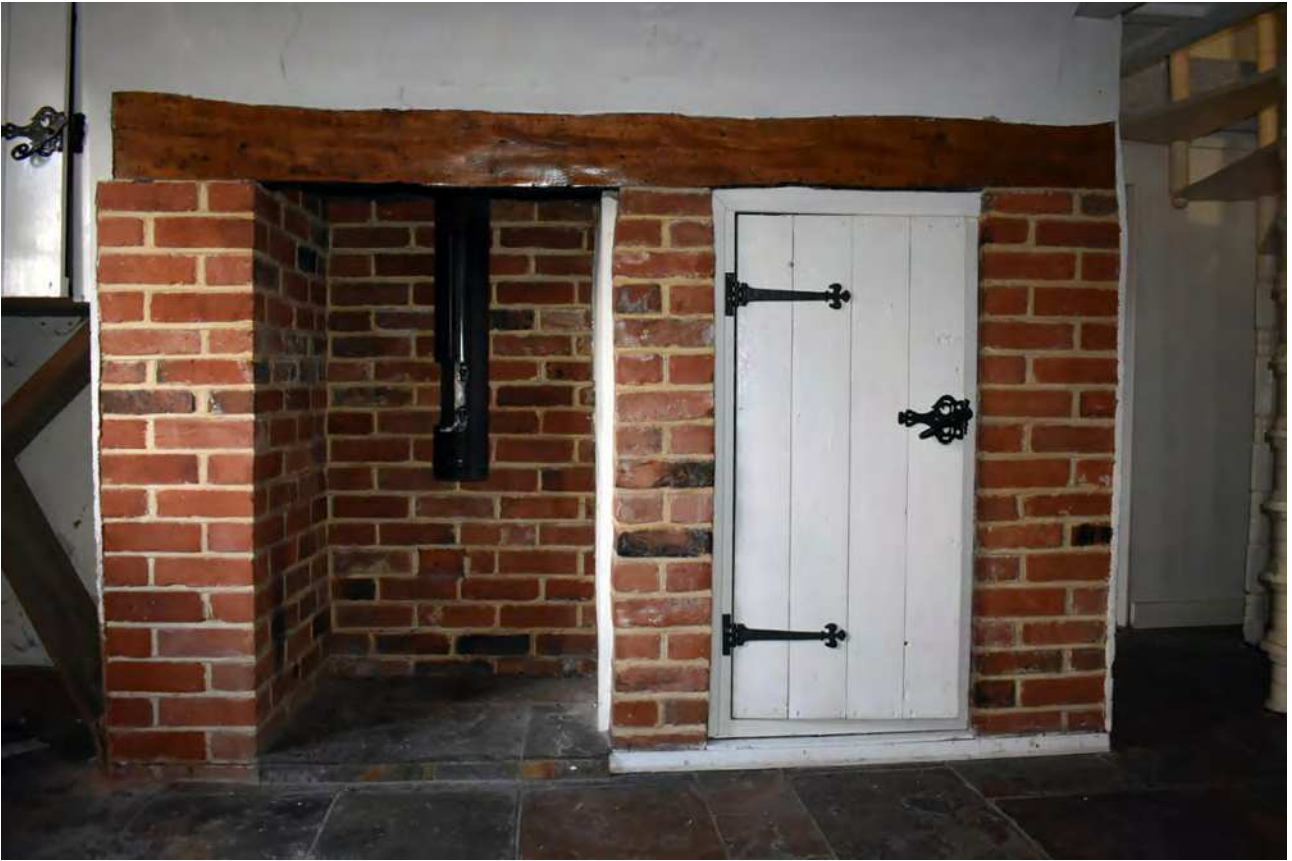
Plate 37: Ground floor, central bay, north wall, the chimney
