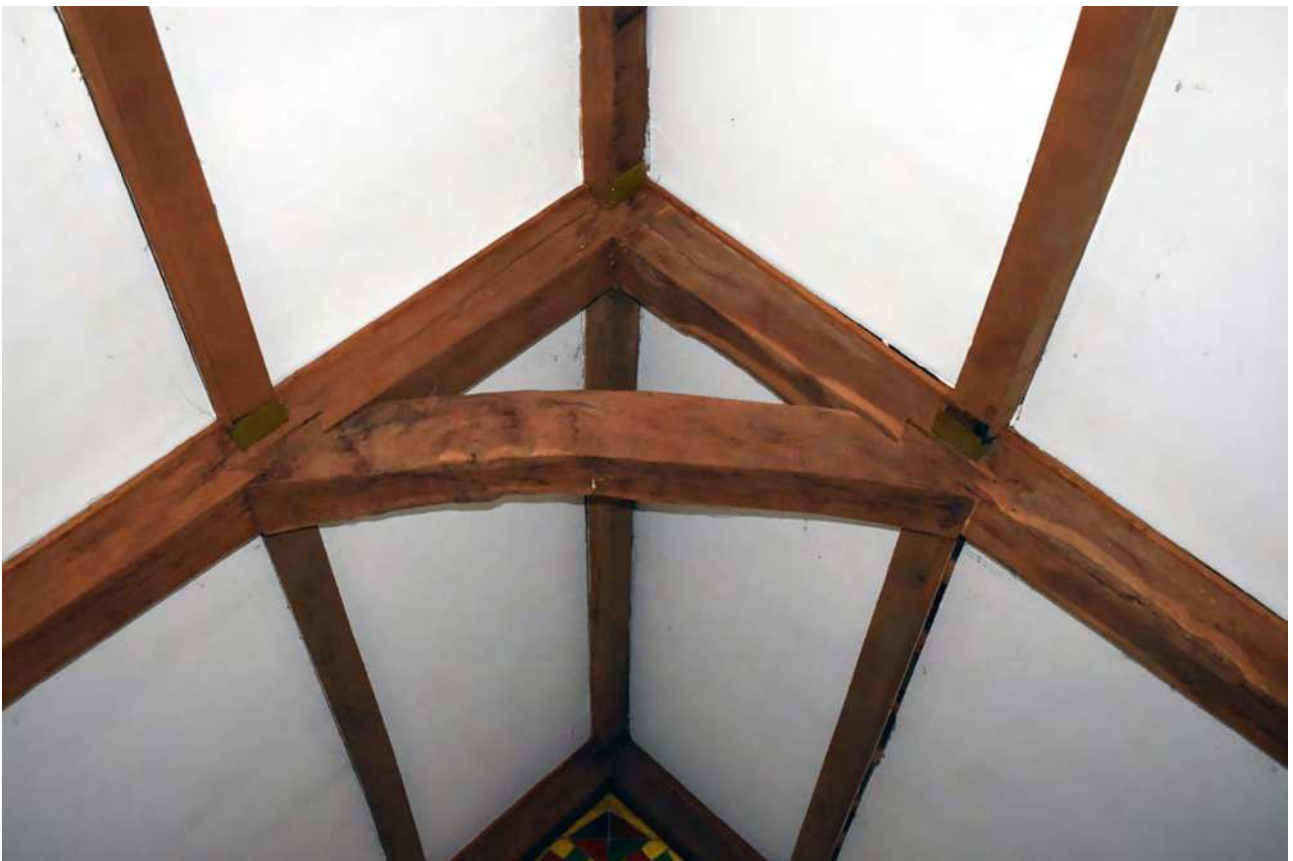
Plate 77: Extension, join between principal rafter collar and purlin
