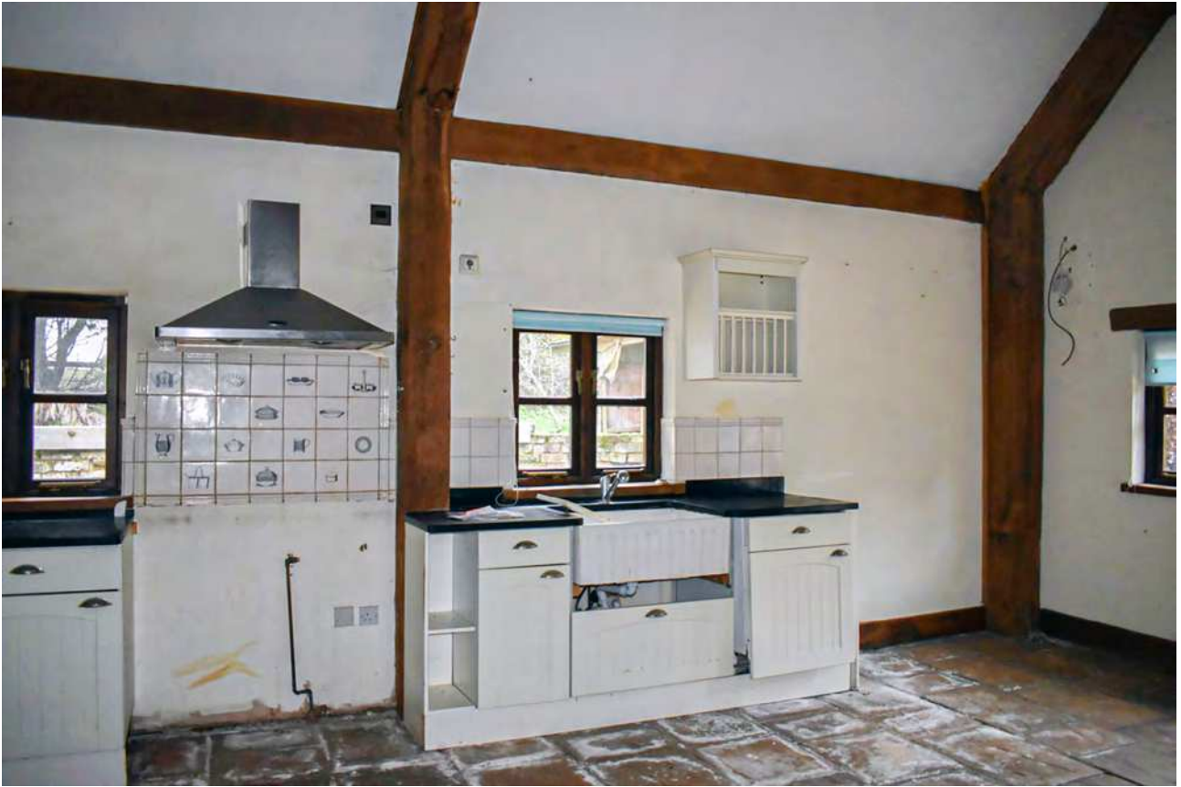
Plate 83: Extension, south bay, south part of the west wall
