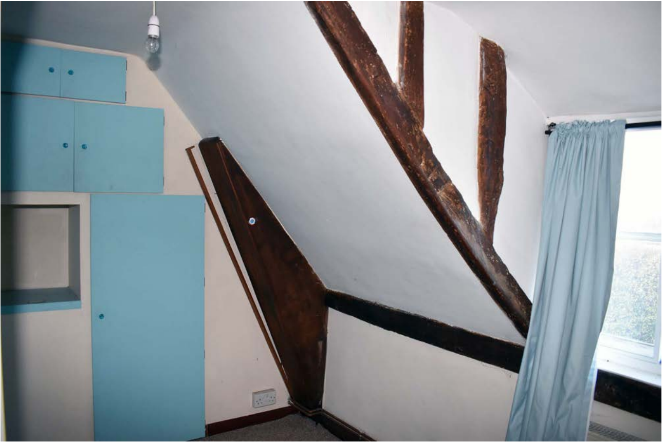
Plate 27: The north-west bedroom of The Thatches looking north-west
