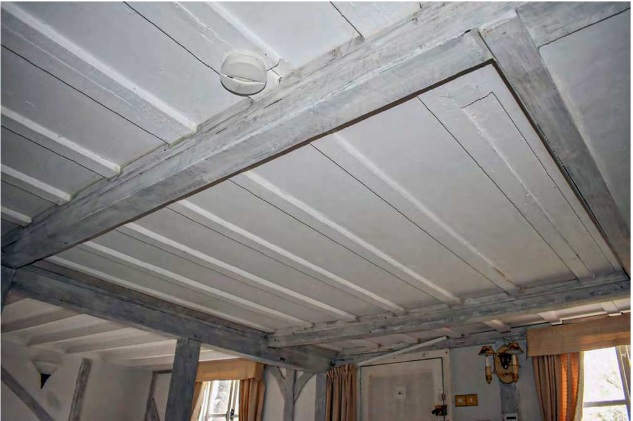
Plate 42: Ground floor, central bay, ceiling beams
