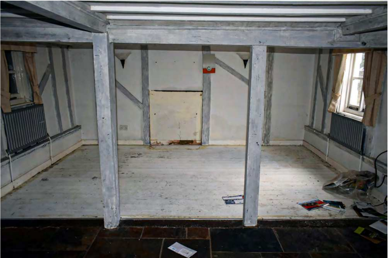
Plate 43: Ground floor, central bay, ceiling beams
