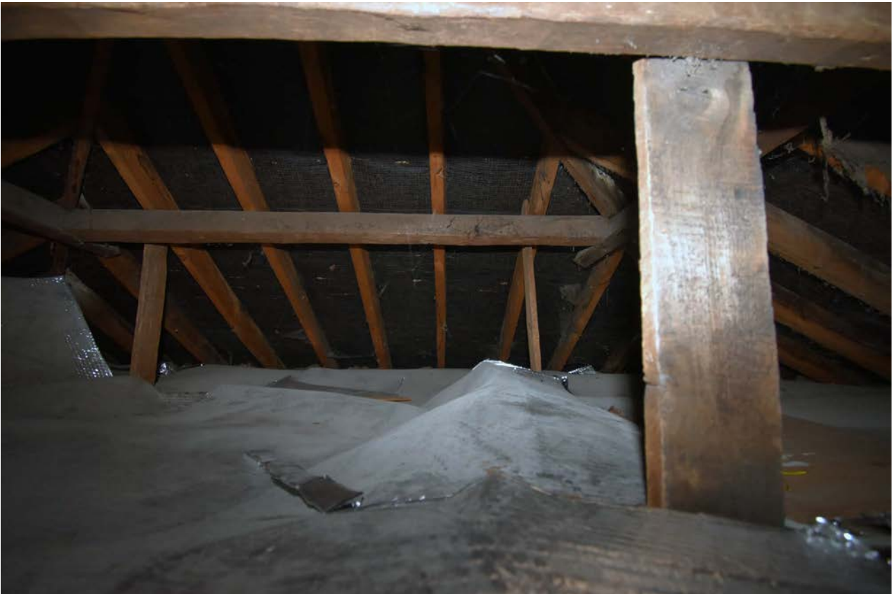
Plate 81: Roof of extension, north part
