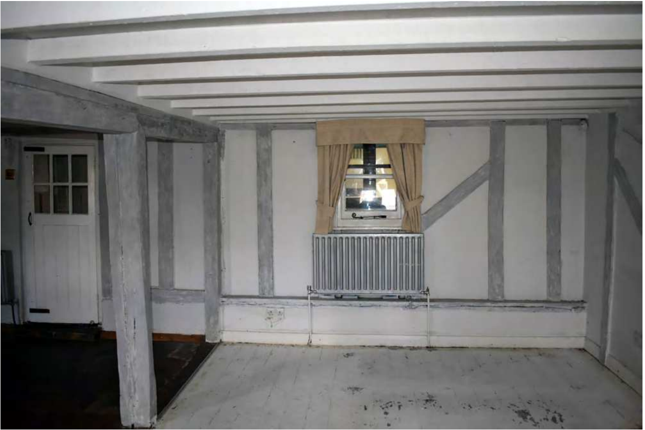
Plate 33: Ground floor, south bay, east wall
