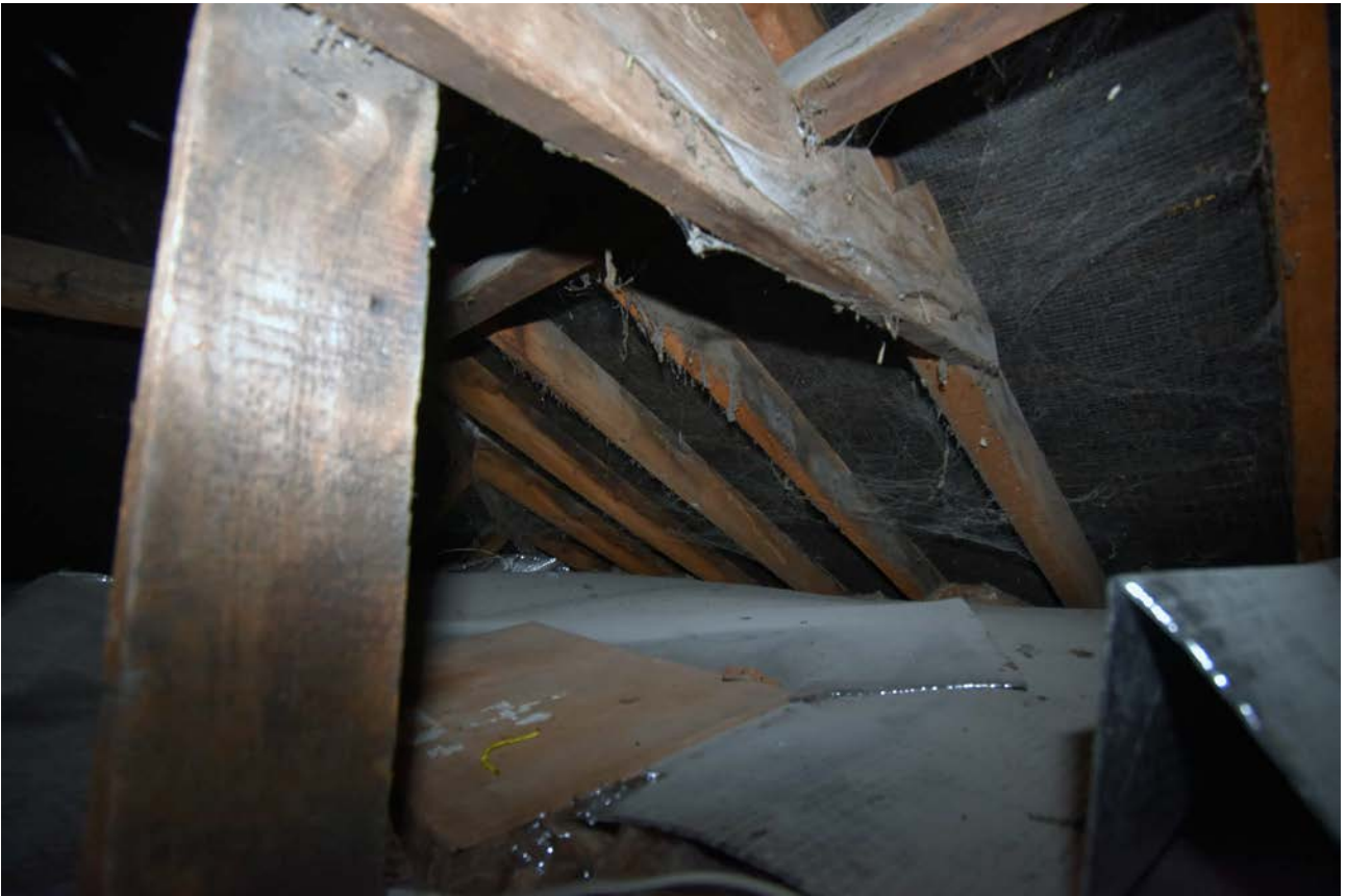
Plate 83: Roof of extension, south- east corner
