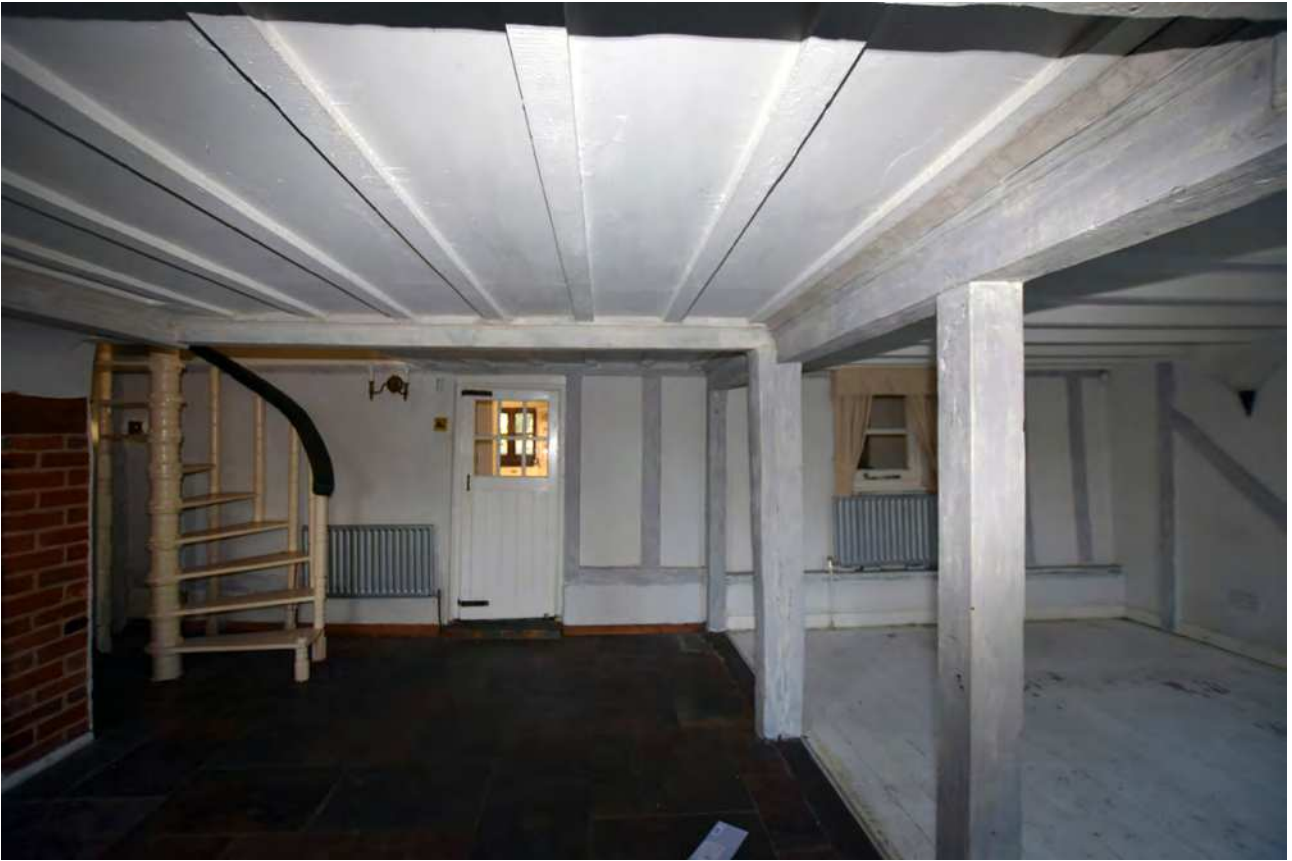
Plate 35: Ground floor, central and south bay, east wall
