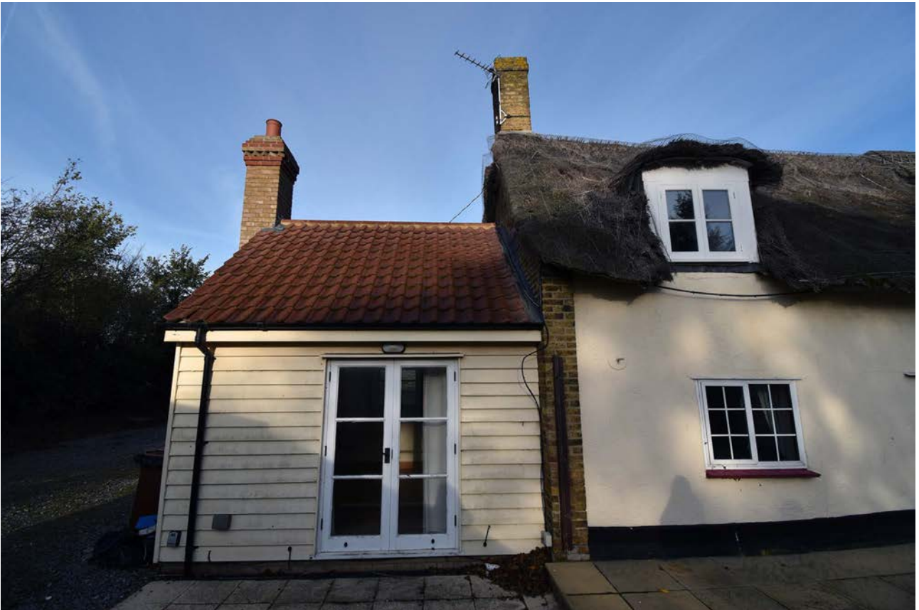
Plate 6: The south elevation of the extension to The Thatches
