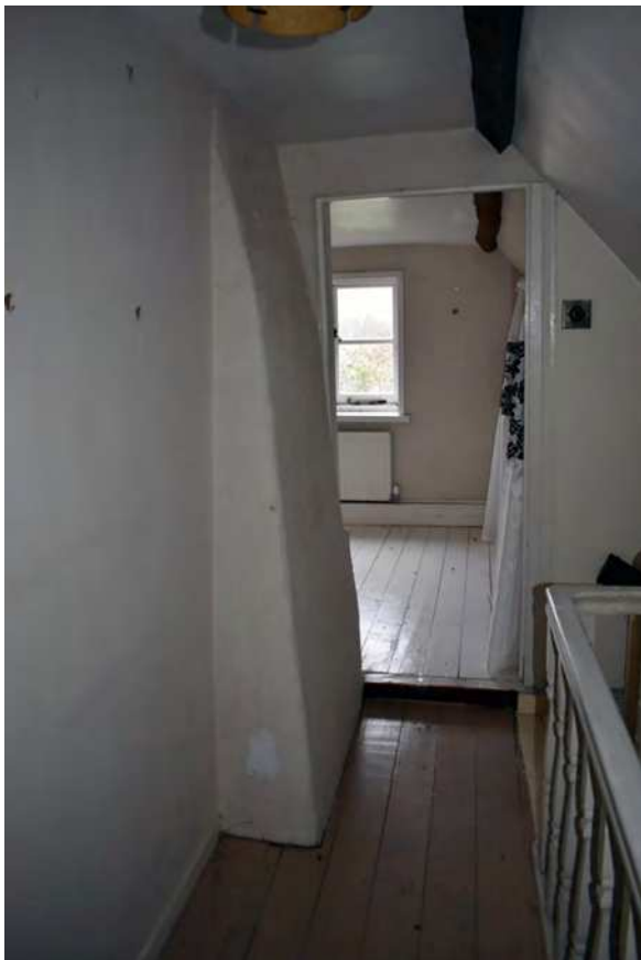
Plate 53: First floor, central bay, view to the north bay
