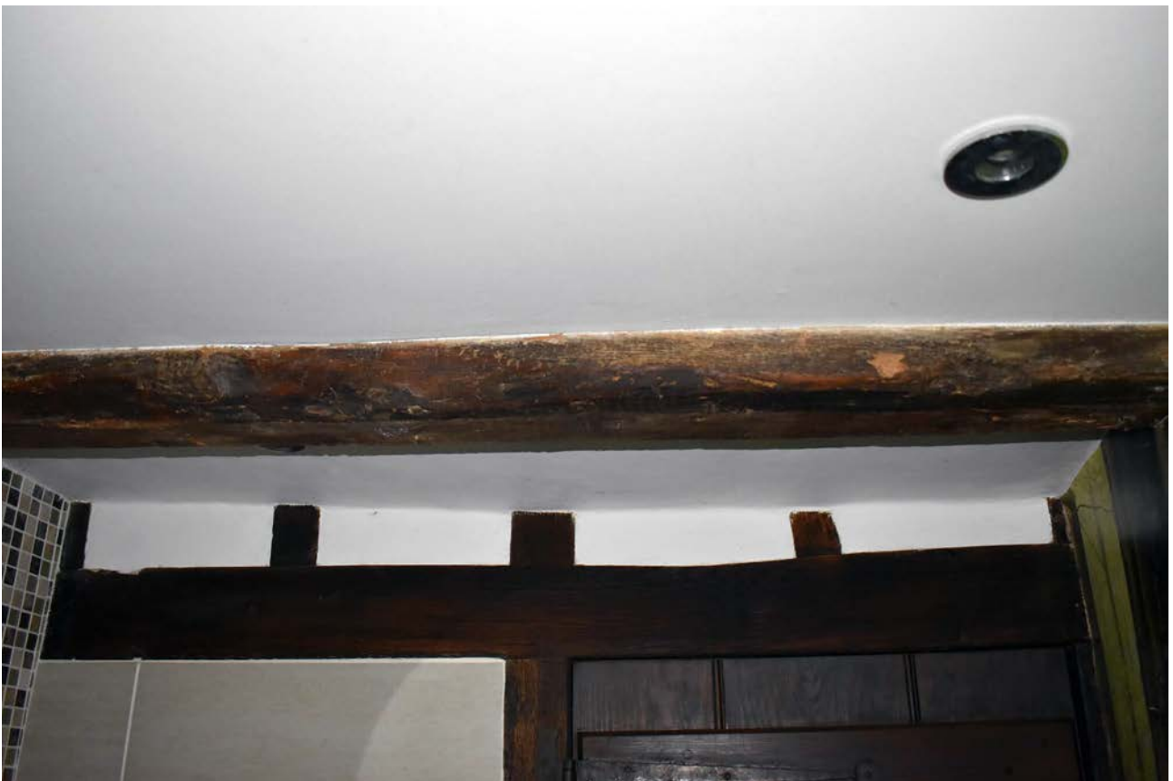
Plate 63: Ground floor, bathroom, ceiling, principal joist
