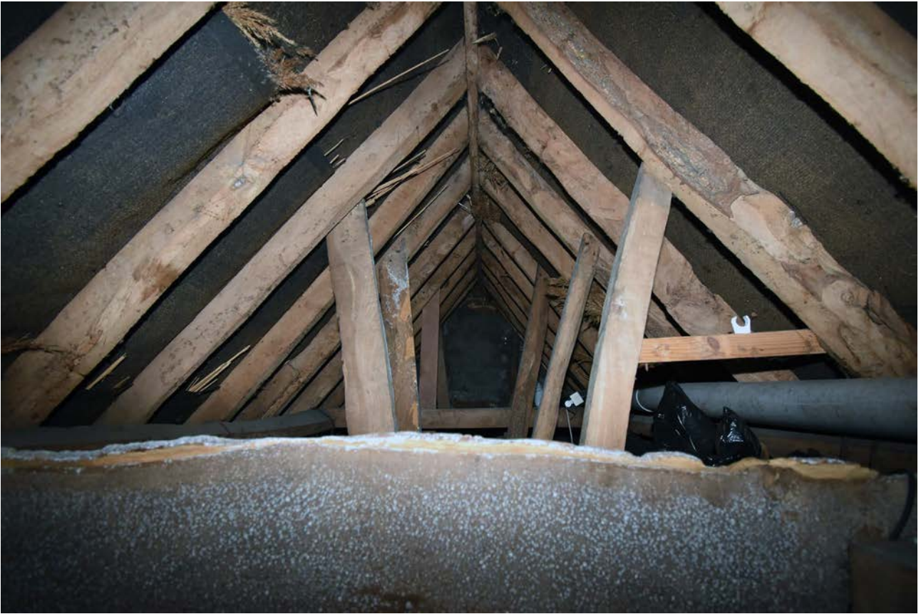
Plate 98: Roof, east part
