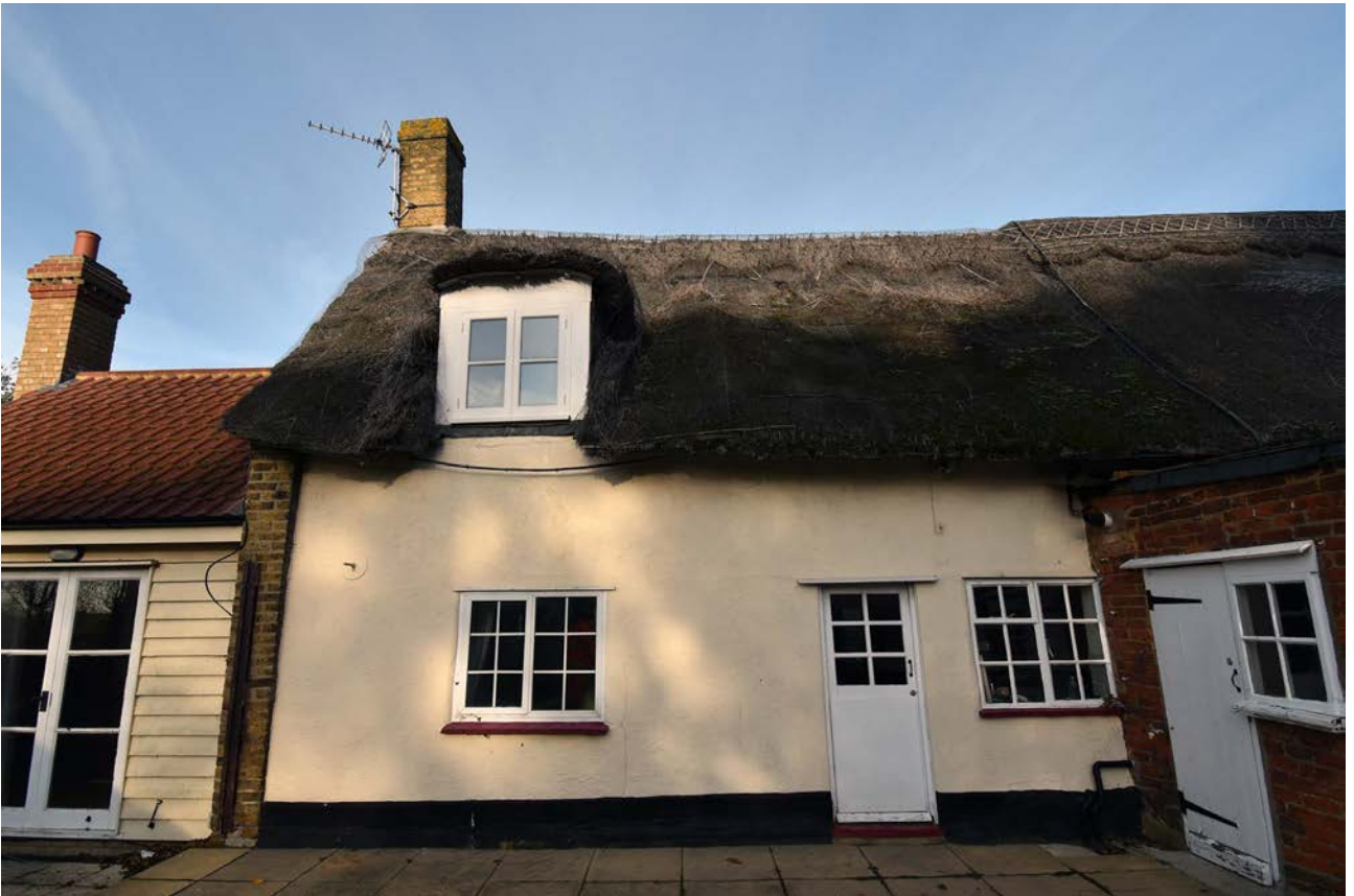
Plate 4: The south elevation of The Thatches
