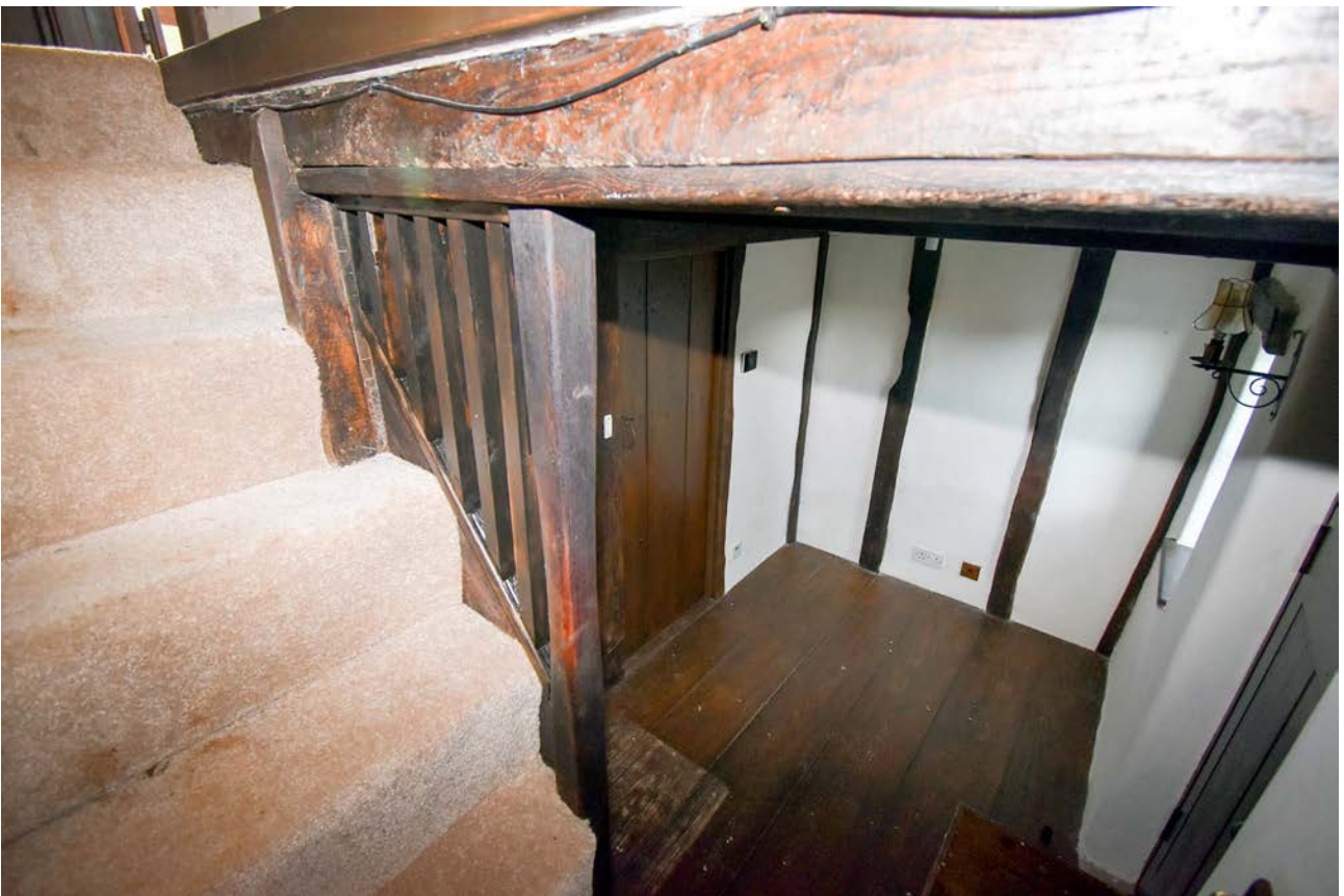
Plate 87: Staircase, view for entrance hall
