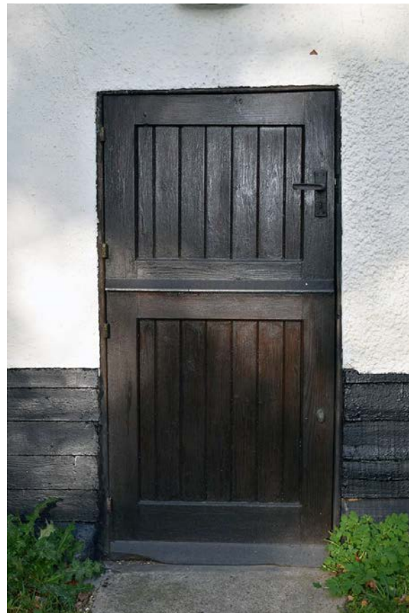
Plate 47: Extension, south elevation, stable-style wooden door
