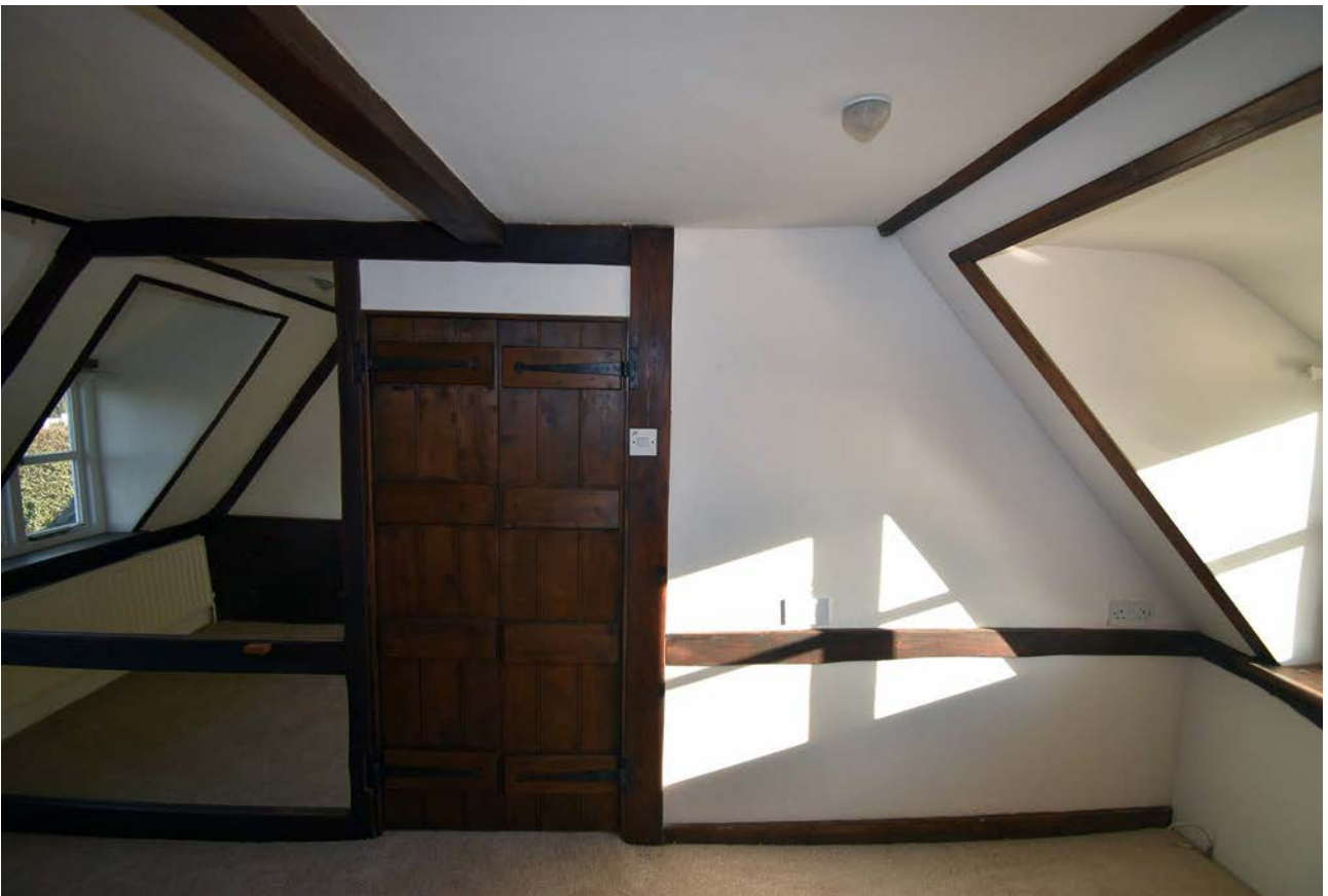
Plate 95: First floor, wardrobe, east wall
