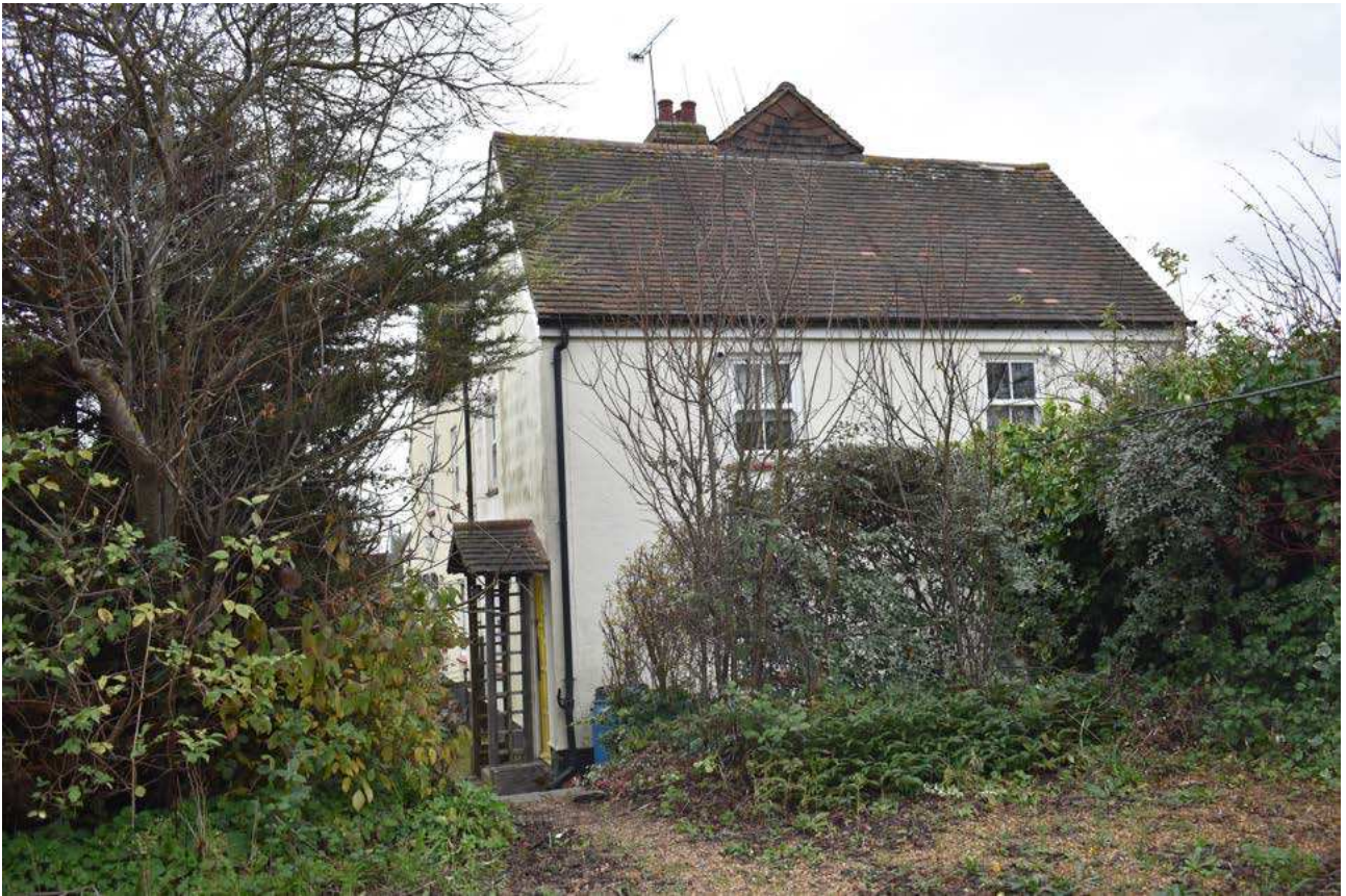
Plate 3: The west elevation of No. 2 Grays Corner Cottages
