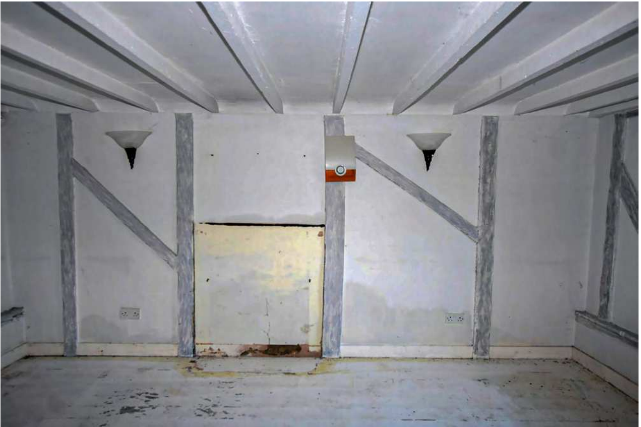
Plate 32: Ground floor, south bay, south wall
