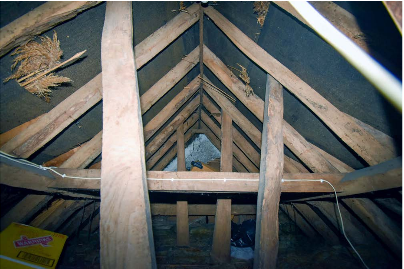
Plate 99: Roof, west part
