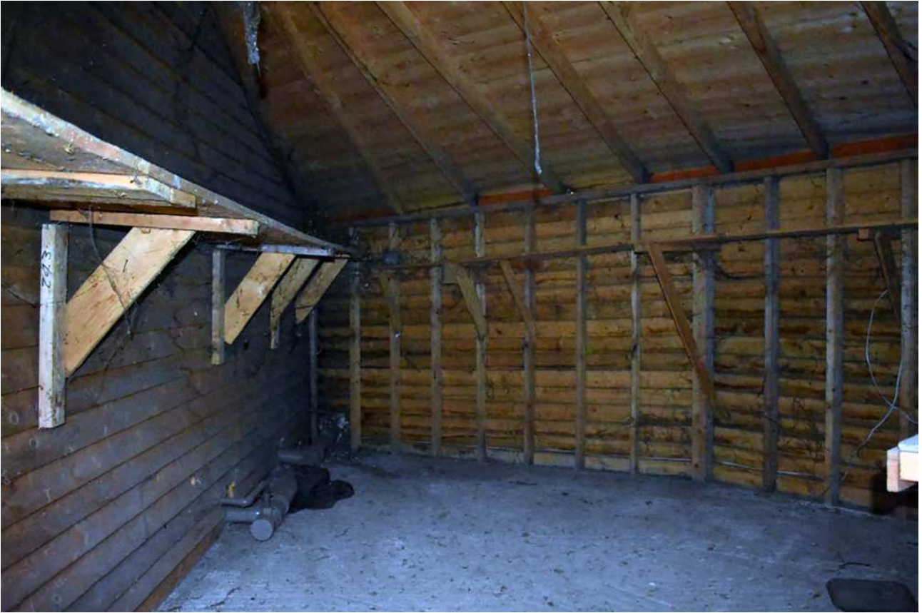
Plate 21: Linking structure, interior
