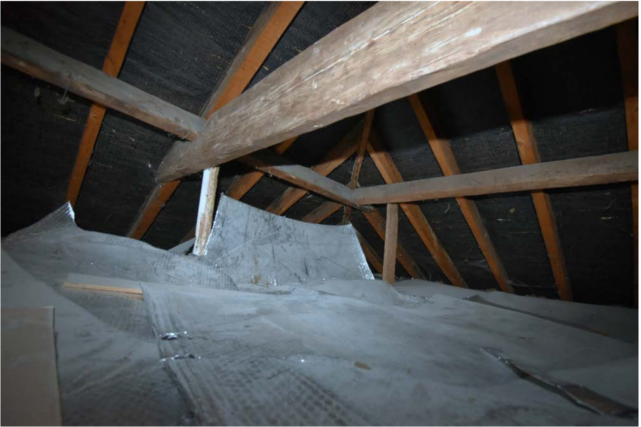
Plate 82: Roof of extension, north- east corner
