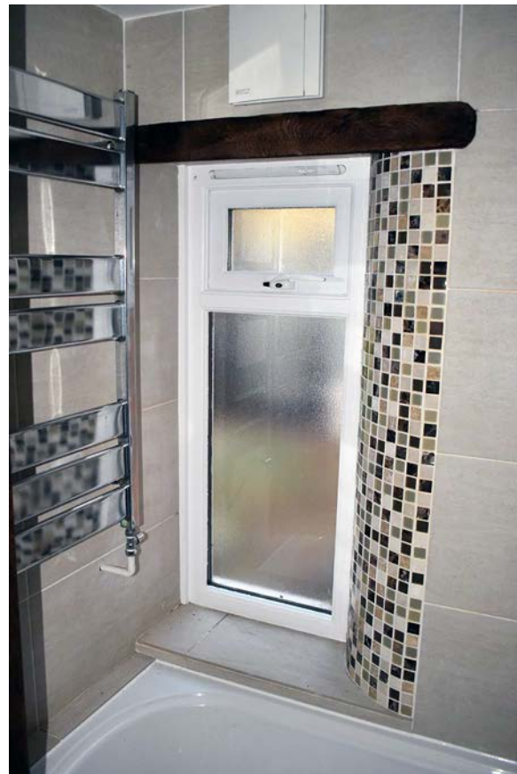
Plate 61: Ground floor, bathroom, south wall, small window featuring an upper awning light
