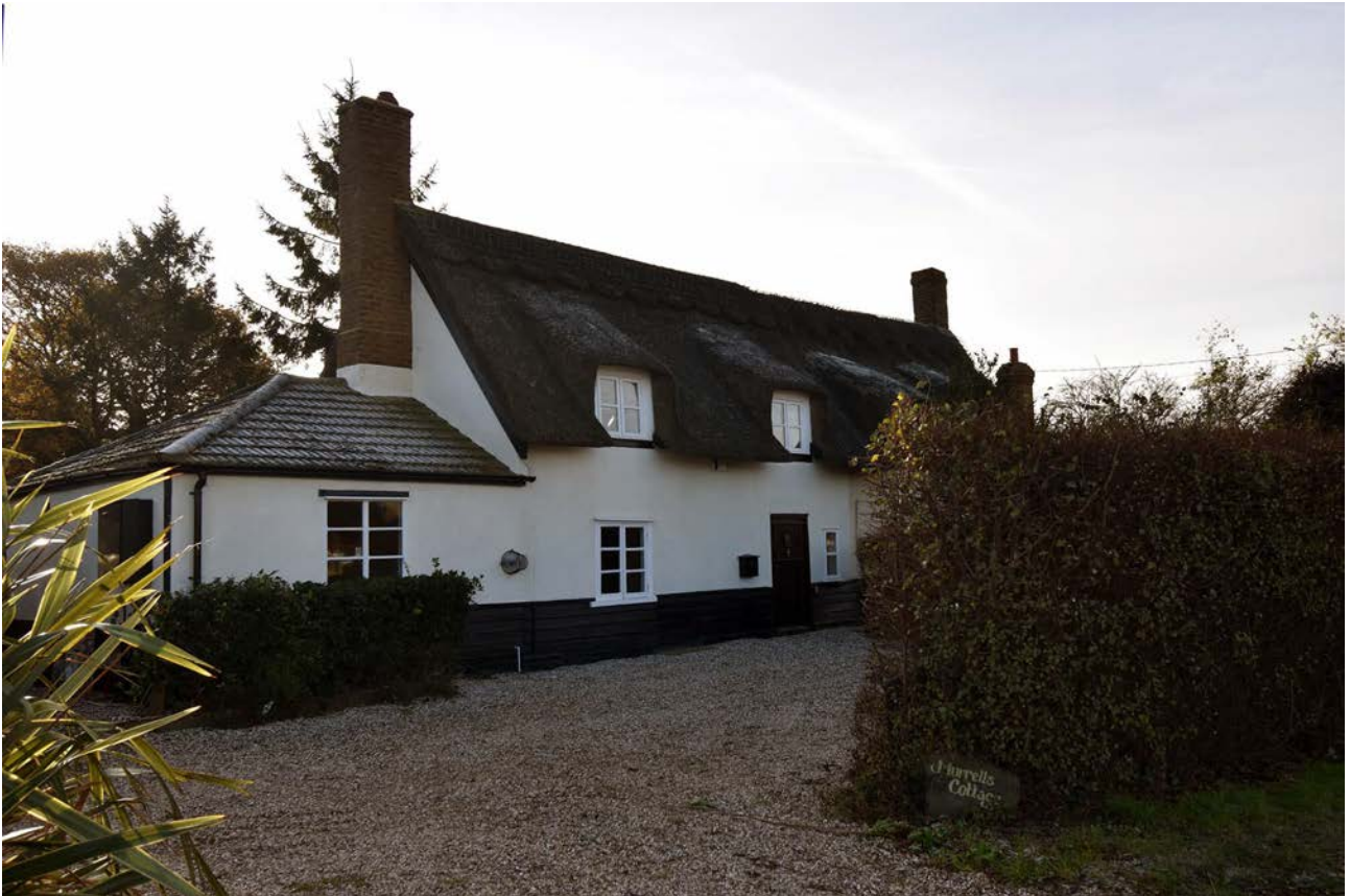
Plate 37: North elevation, front façade
