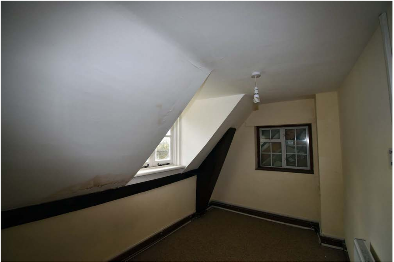
Plate 29: The south-west bedroom of The Thatches looking south-west
