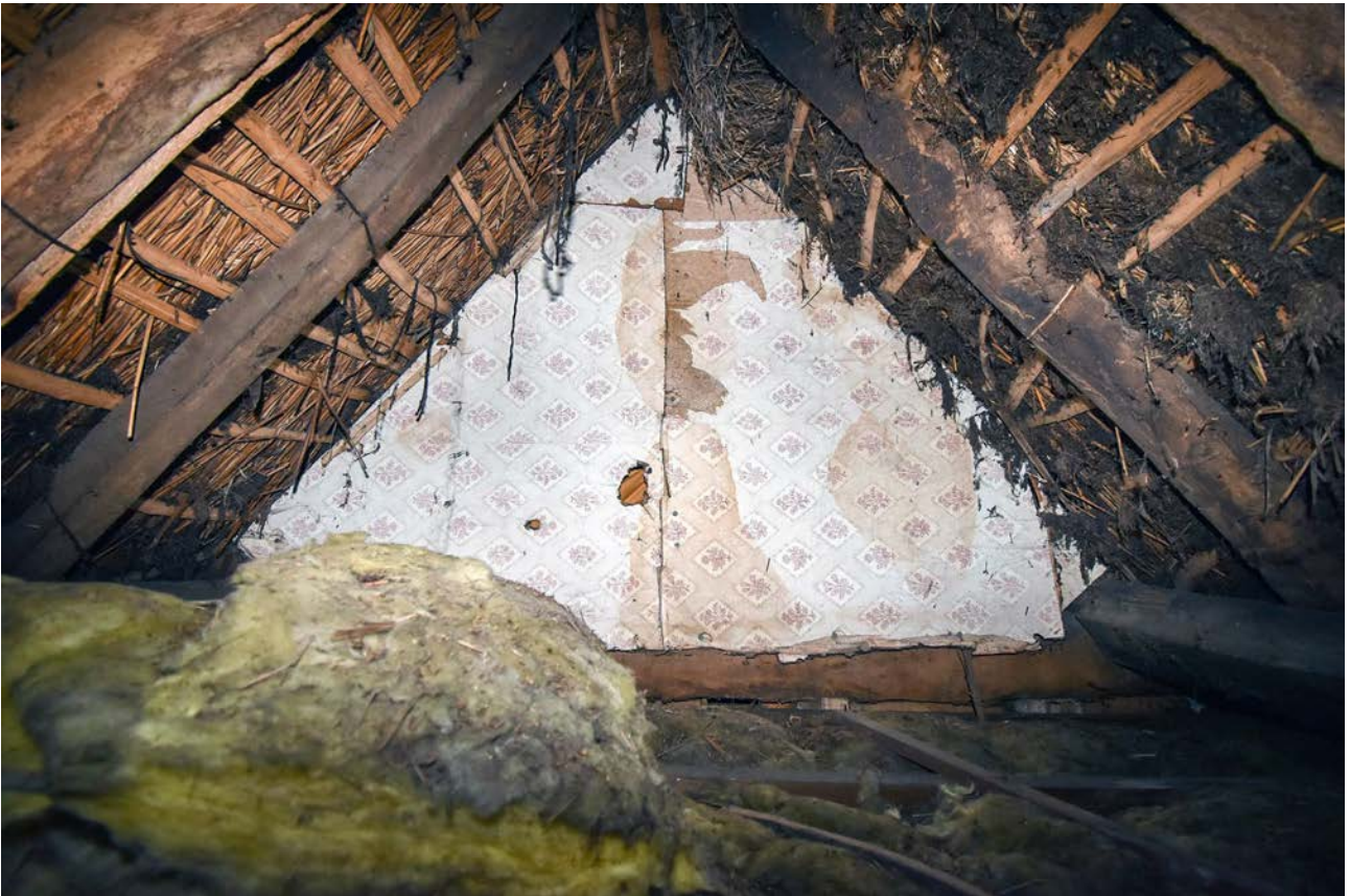
Plate 32: The attic of The Thatches looking east
