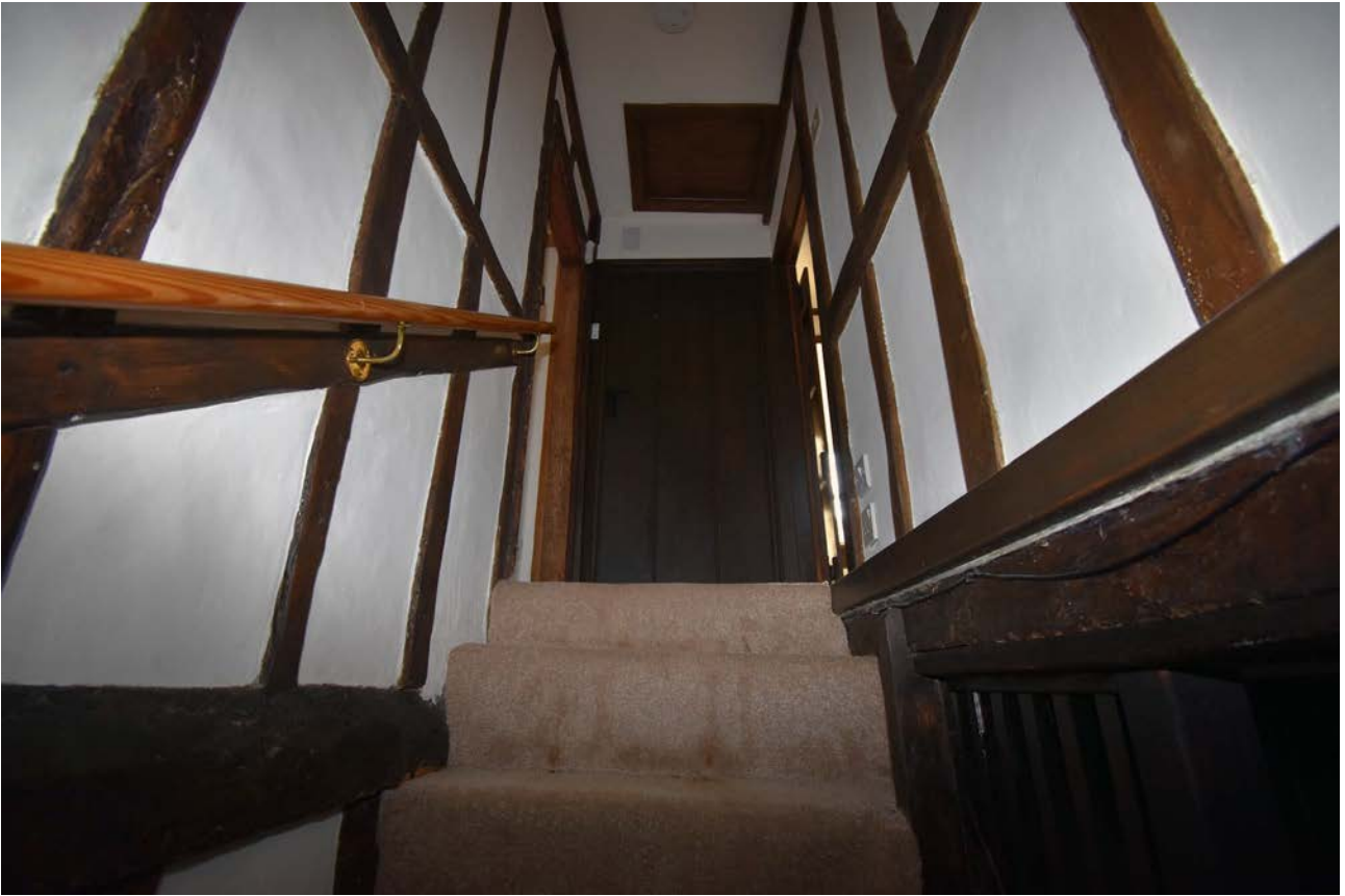
Plate 86: Staircase, view for landing
