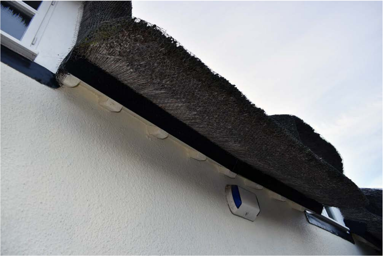
Plate 100: Roof, north elevation, rafter feet
