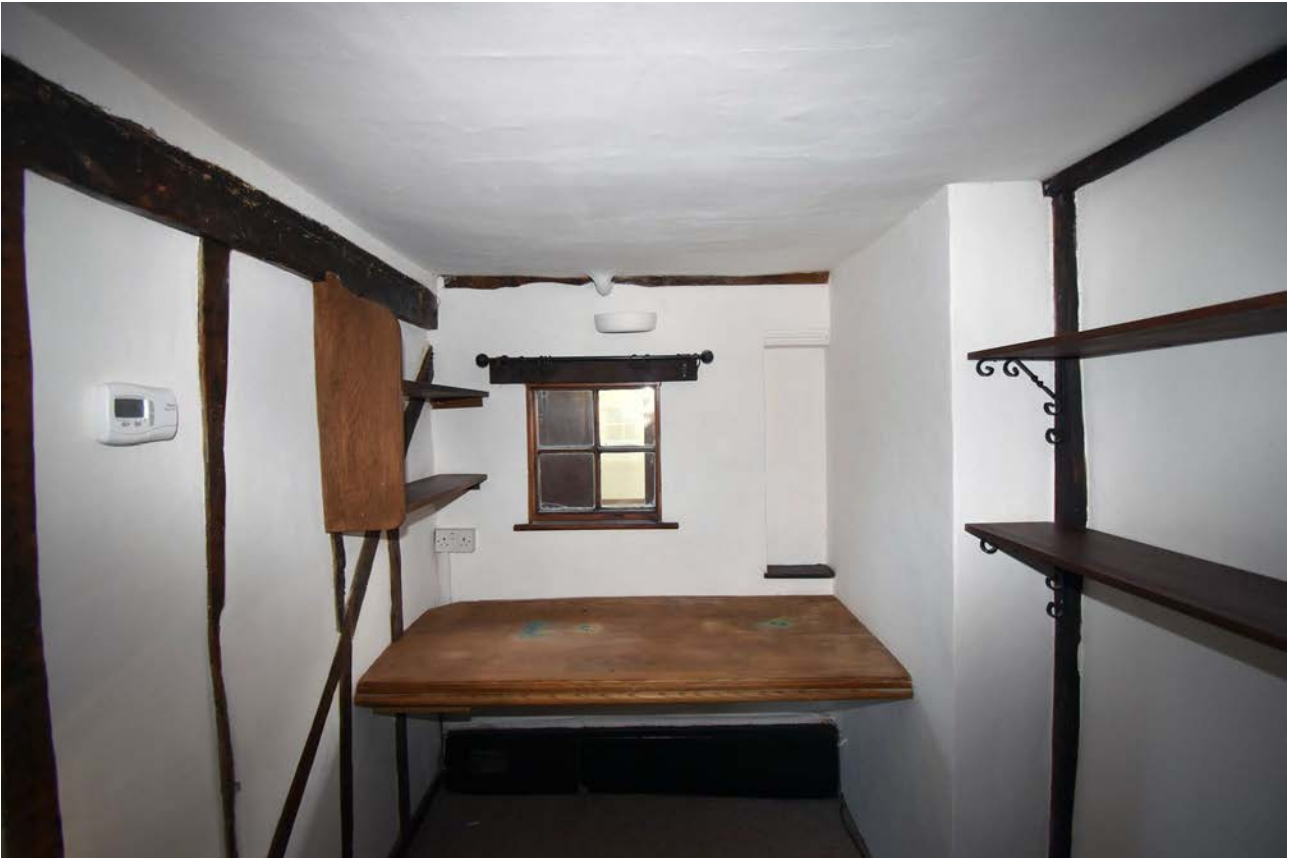
Plate 64: Ground floor, lobby, south wall
