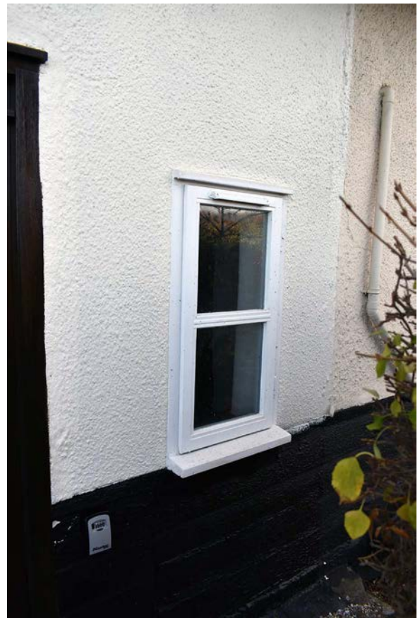
Plate 41: North elevation, small two-light window
