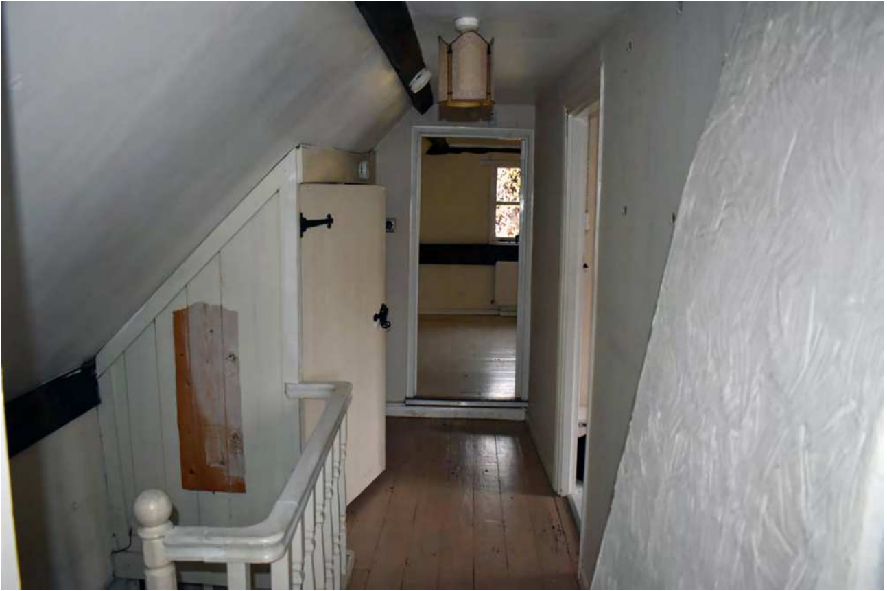
Plate 52: First floor, central bay, view to the south bay
