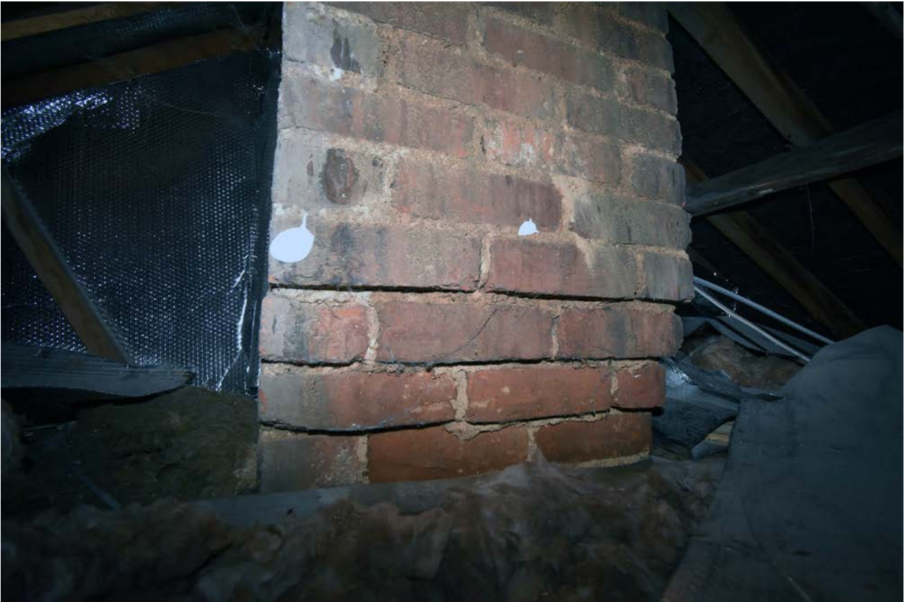
Plate 84: Roof of extension, west part with chimney
