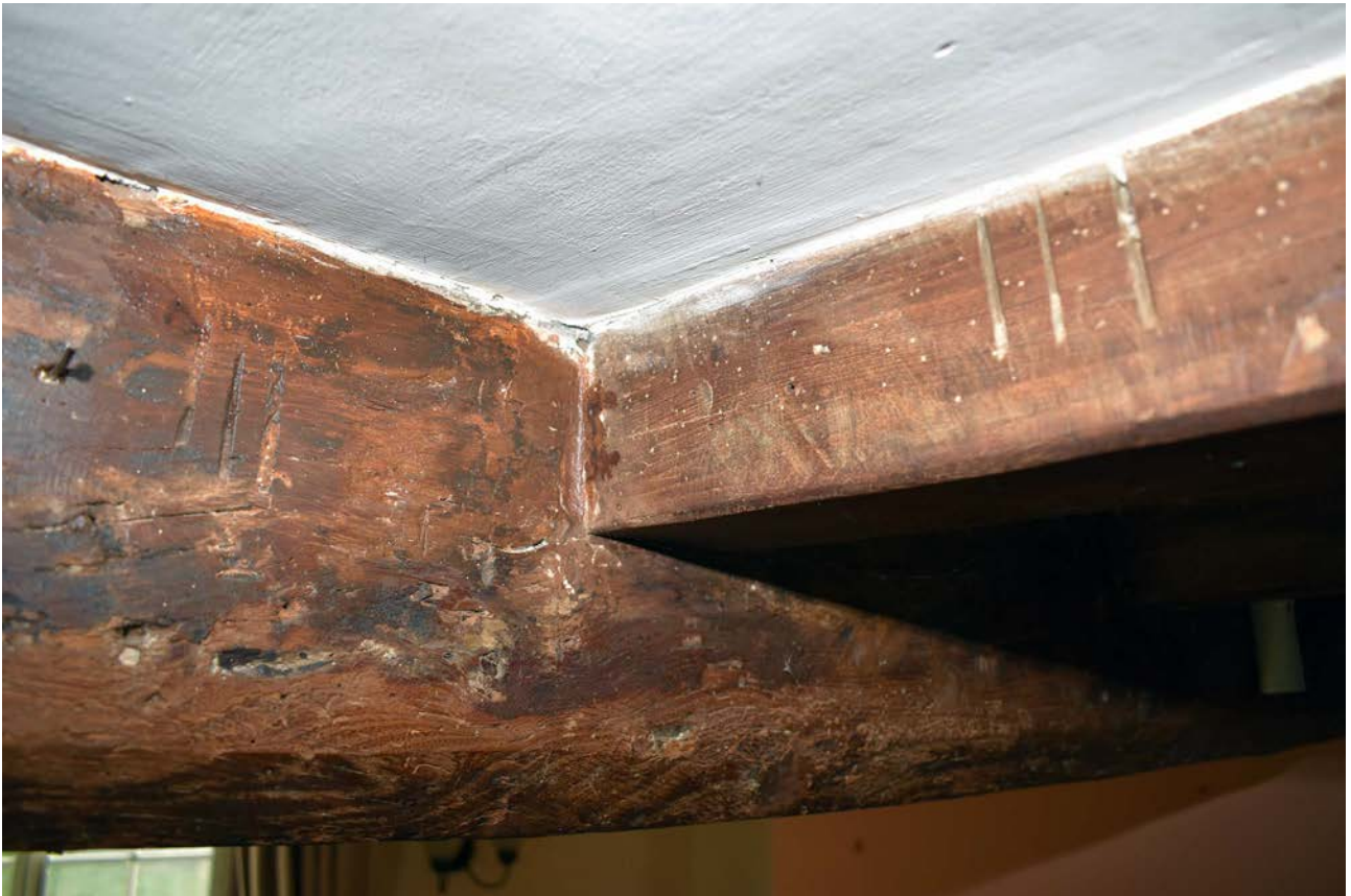
Plate 10: Pair of carpenters' marks on the ceiling of the central reception room
