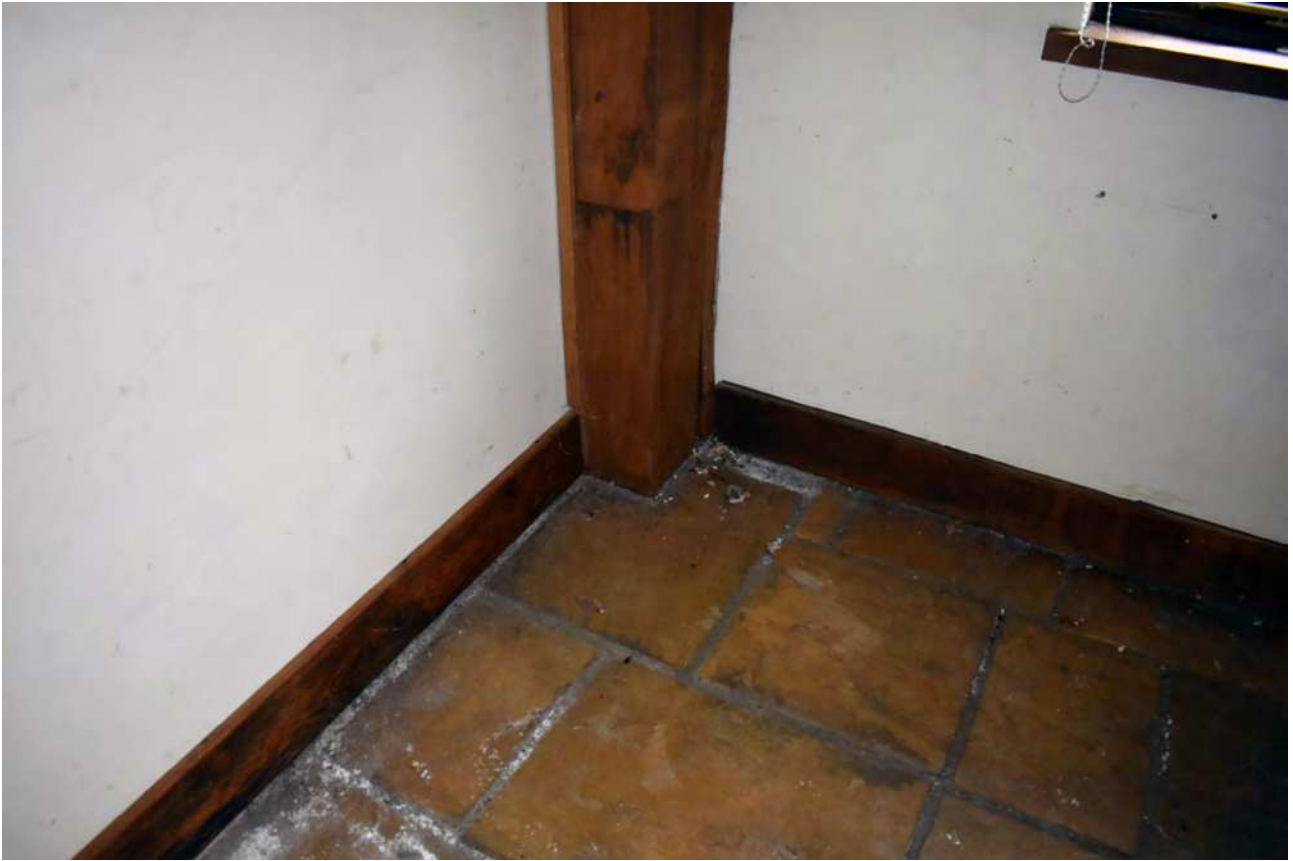
Plate 81: Extension, central bay, floor
