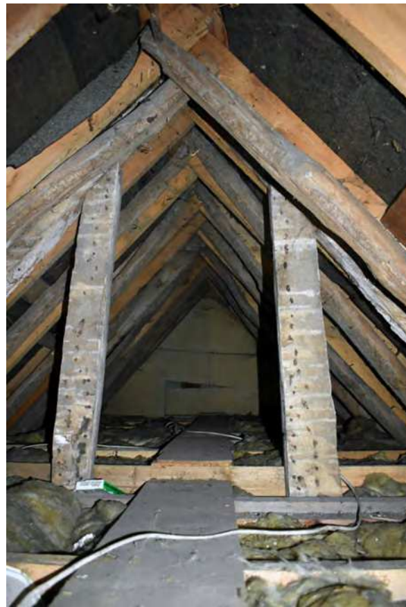
Plate 69: Roof, view to the south
