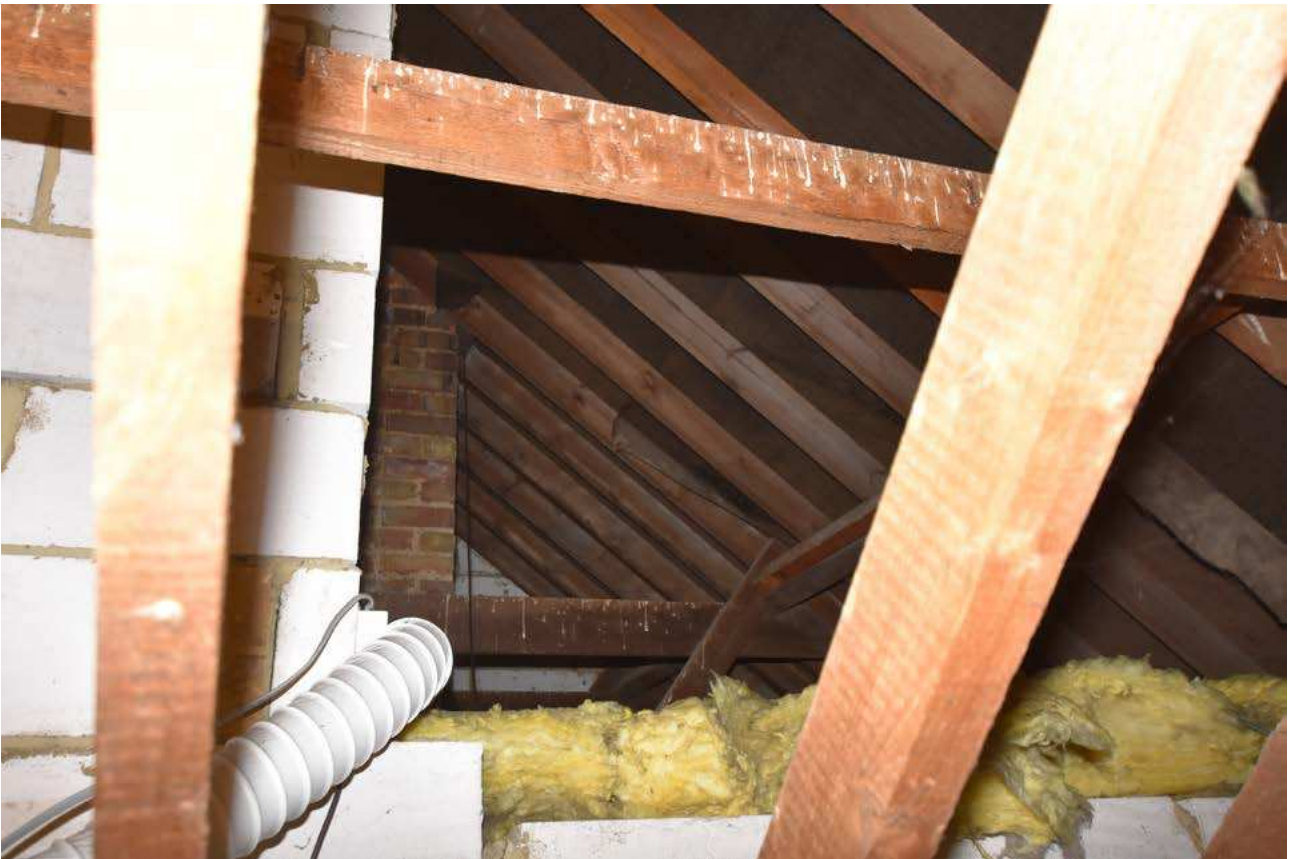
Plate 20: The attic looking south-east into the older roof space
