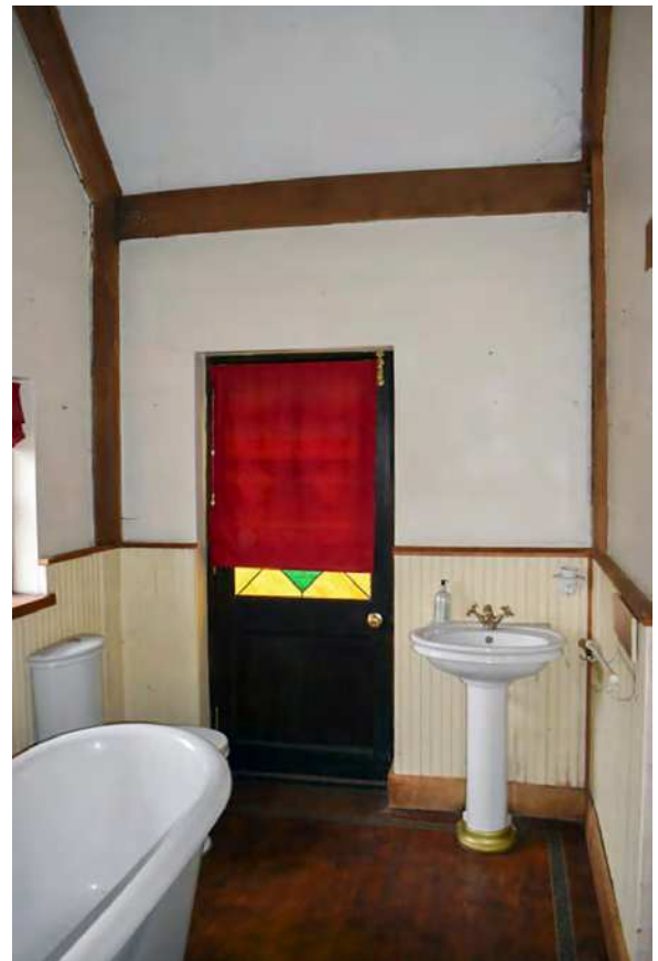
Plate 90: Extension, north bay, east wall
