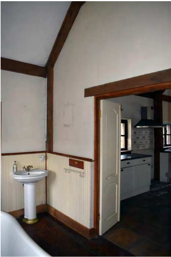
Plate 91: Extension, north bay, south- east corner
