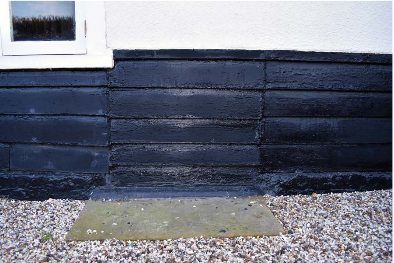
Plate 39: North elevation, trace of the earlier door
