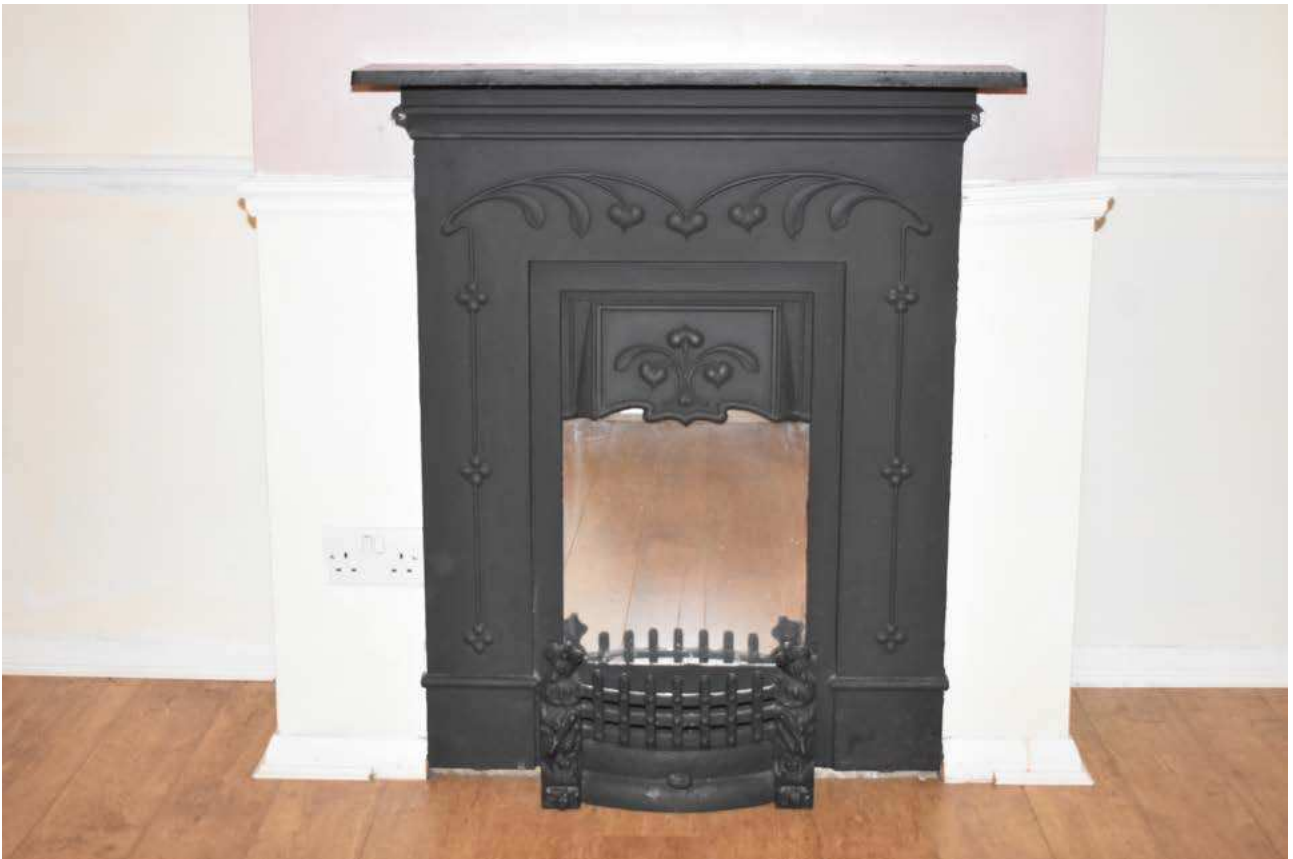
Plate 18: The fire surround and grate in the principal bedroom
