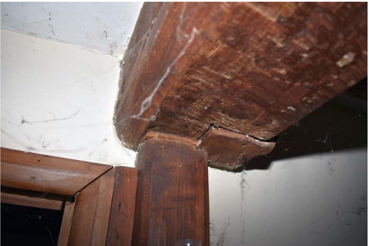
Plate 12: Truncated post in central reception room
