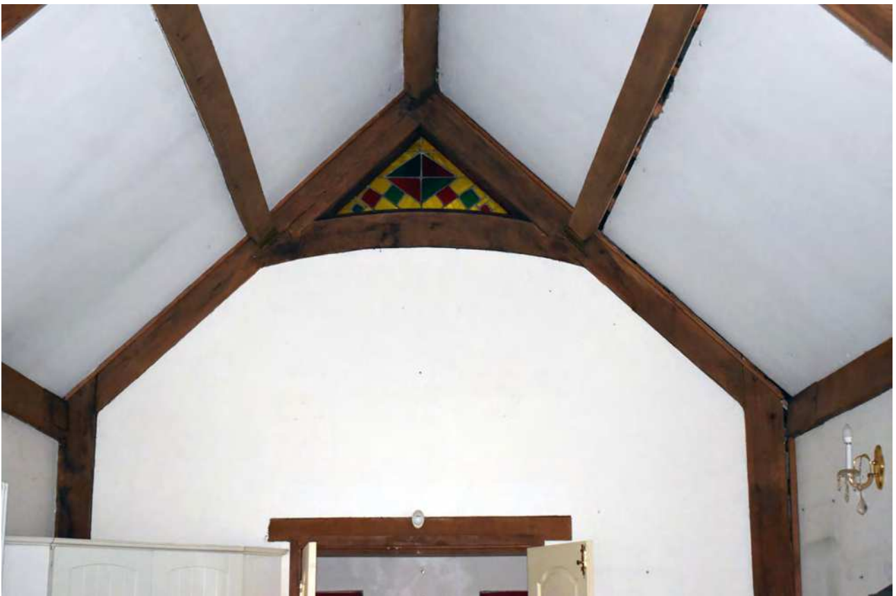
Plate 75: Extension, central bay, north wall
