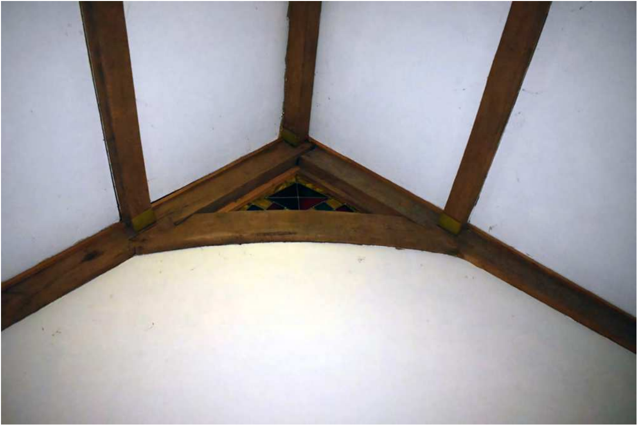
Plate 94: Extension, north bay, south wall, apex
