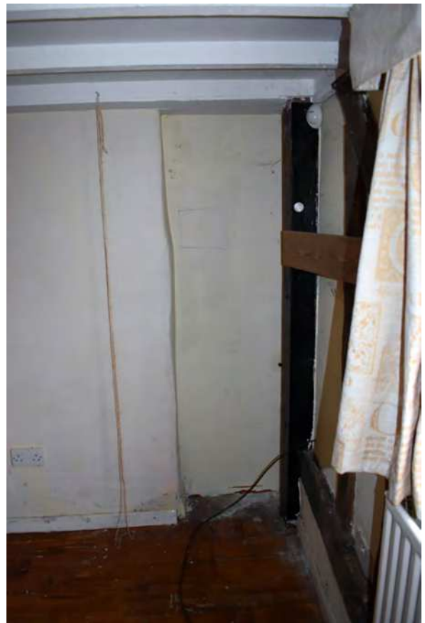
Plate 47: Ground floor, north bay, west part of the south wall
