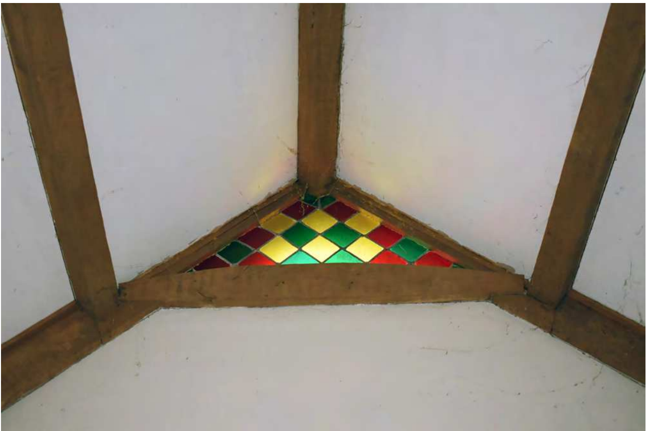
Plate 93: Extension, north bay, north wall, apex
