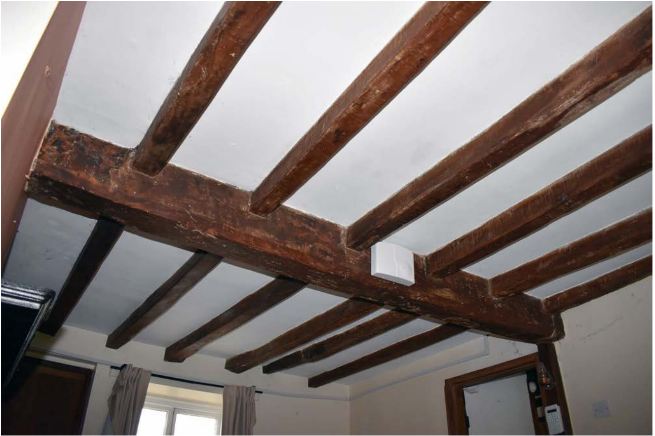
Plate 9: The ceiling of the central reception room looking north-east
