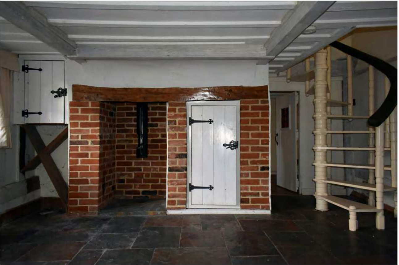
Plate 39: Ground floor, central bay, north wall
