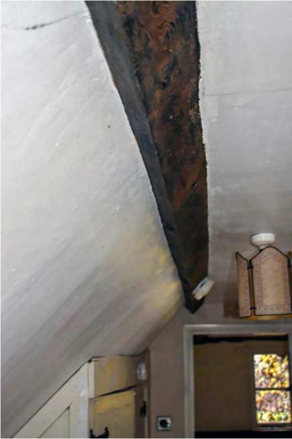
Plate 55: First floor, central bay, east purlin, view to the south
