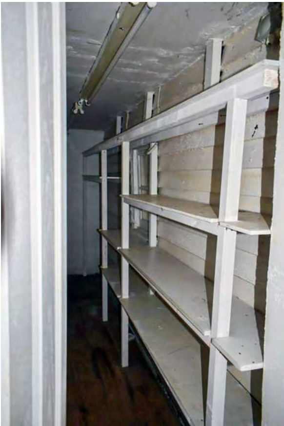
Plate 73: Passage between cottage and extension, south part
