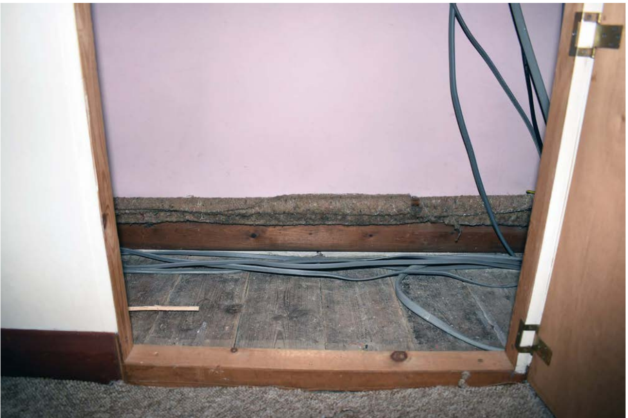
Plate 28: Floorboards in the north-west bedroom of The Thatches
