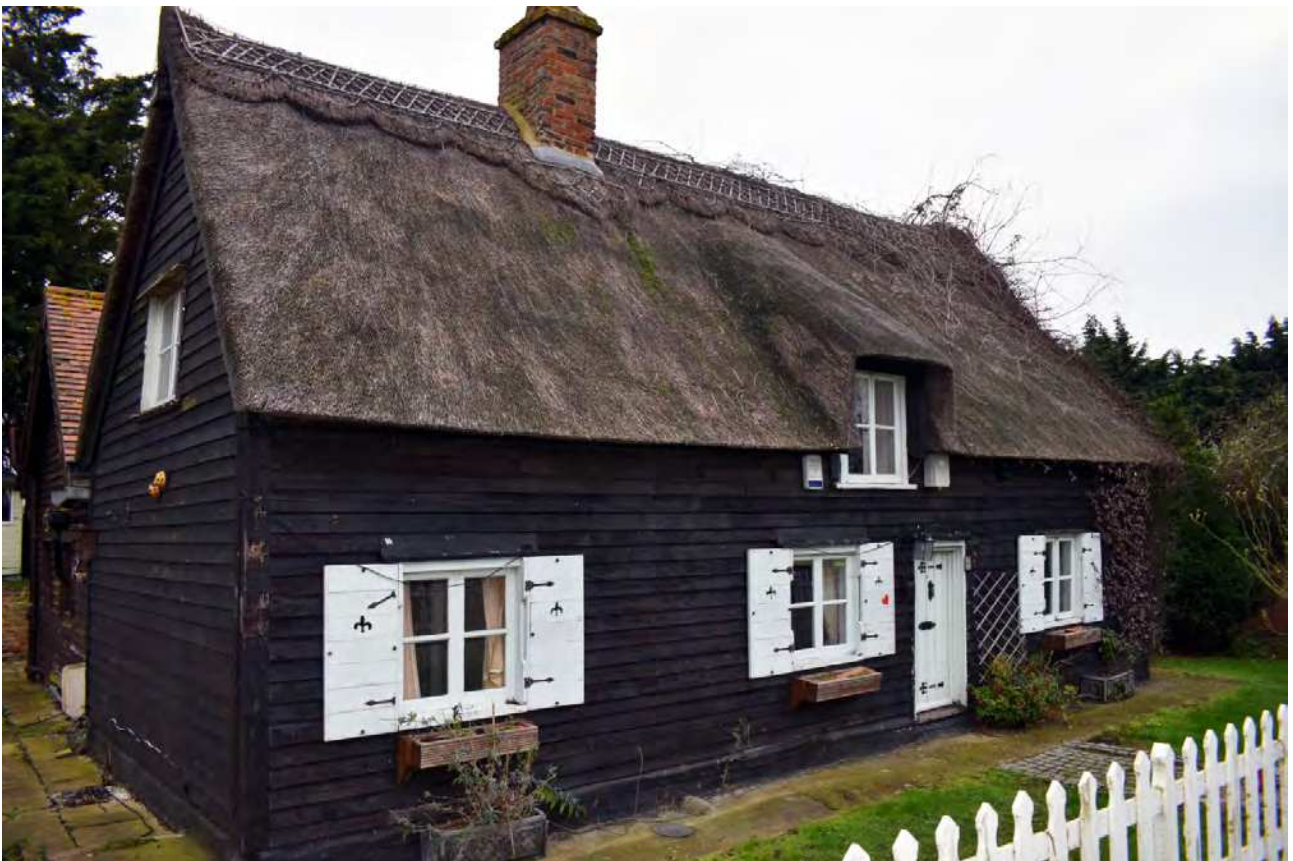
Plate 2: West elevation from north- west corner
