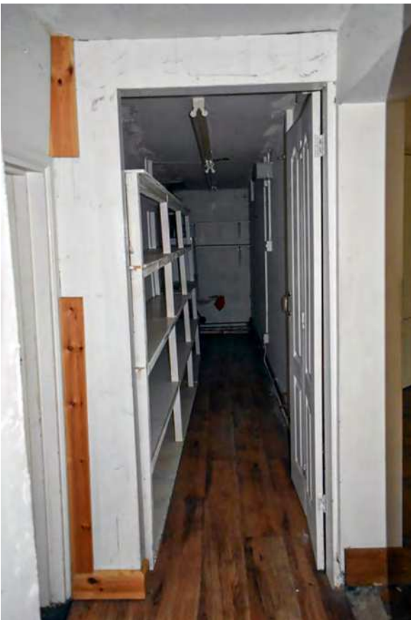
Plate 71: Passage between cottage and extension, north part
