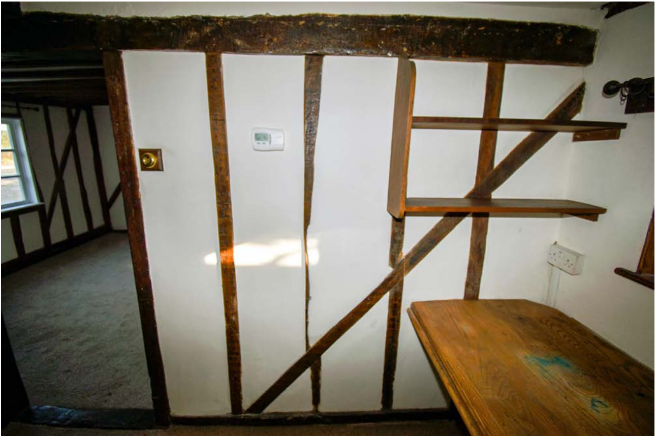
Plate 67: Ground floor, lobby, east wall
