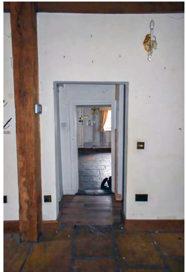
Plate 85: Extension, central bay, west wall, door opening
