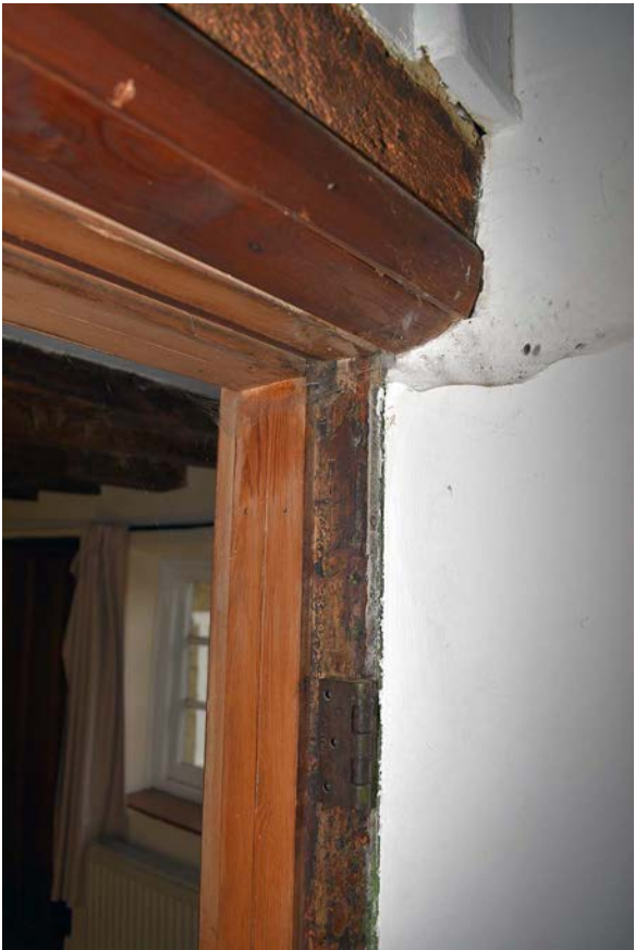
Plate 14: Doorway between the central reception room and the hallway
