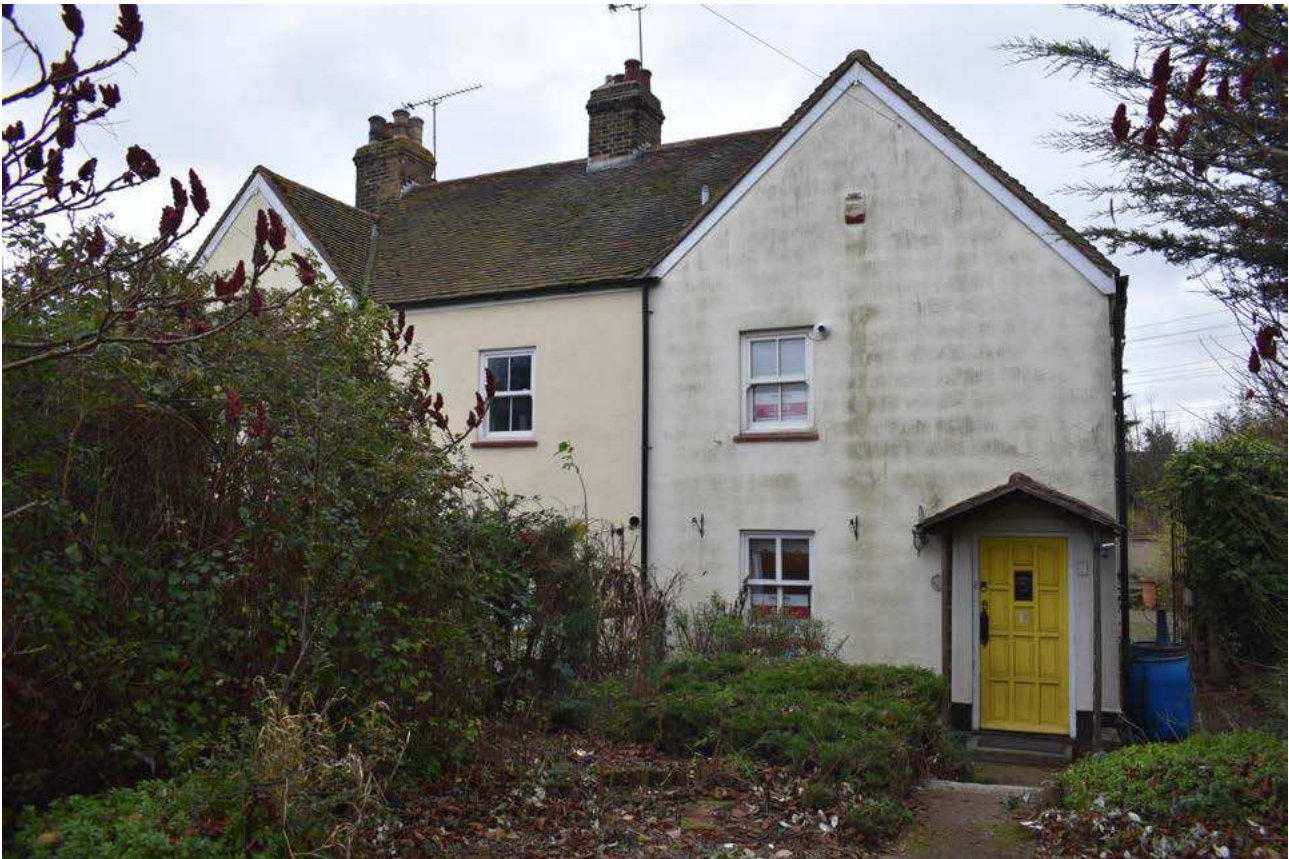
Plate 2: The north elevation of No. 2 Grays Corner Cottages
