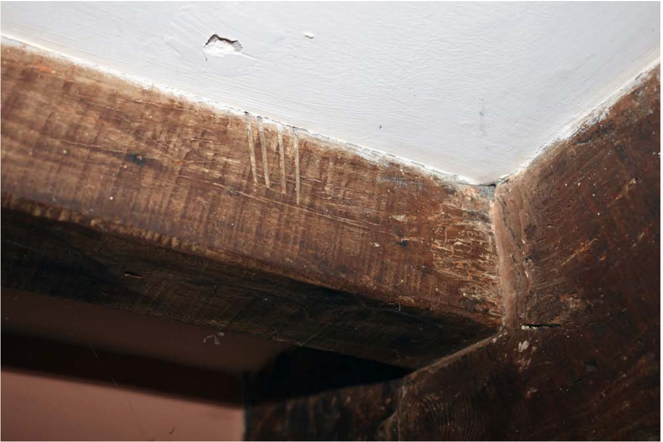
Plate 11: Carpenters' mark on a common joist of the central reception room
