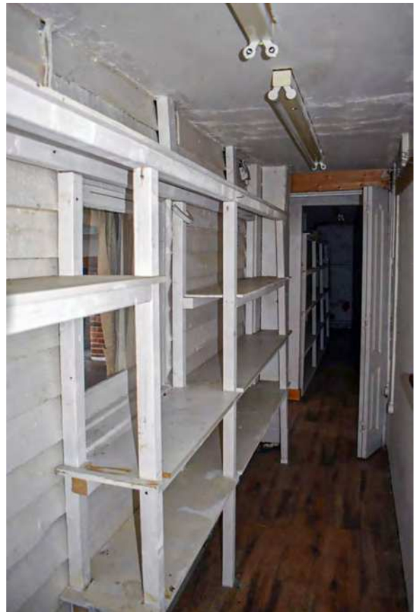
Plate 74: Passage between cottage and extension, south part
