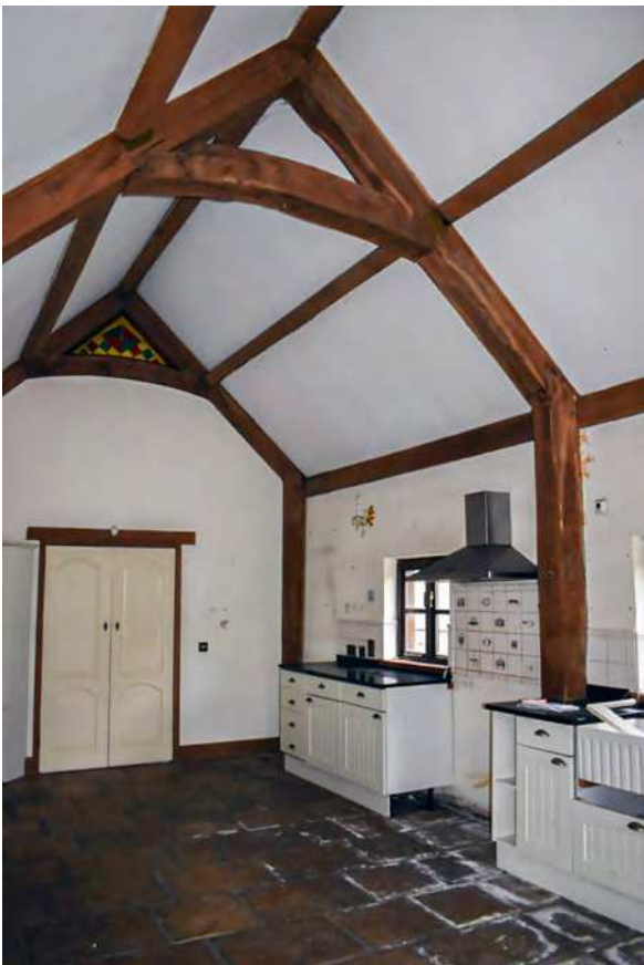
Plate 79: Extension, central bay, view to the north- east corner of the open space
