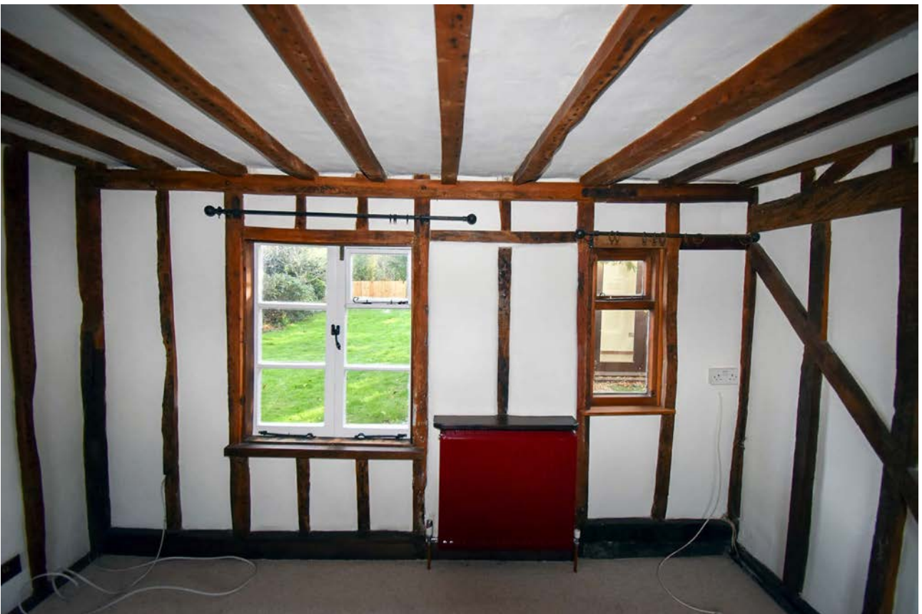
Plate 71: Ground floor, living room, south wall
