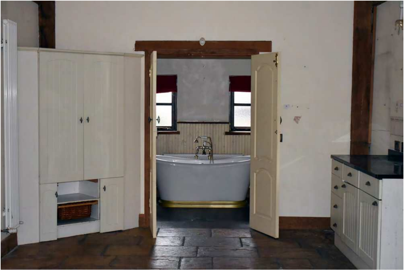
Plate 88: Extension, central bay, north wall
