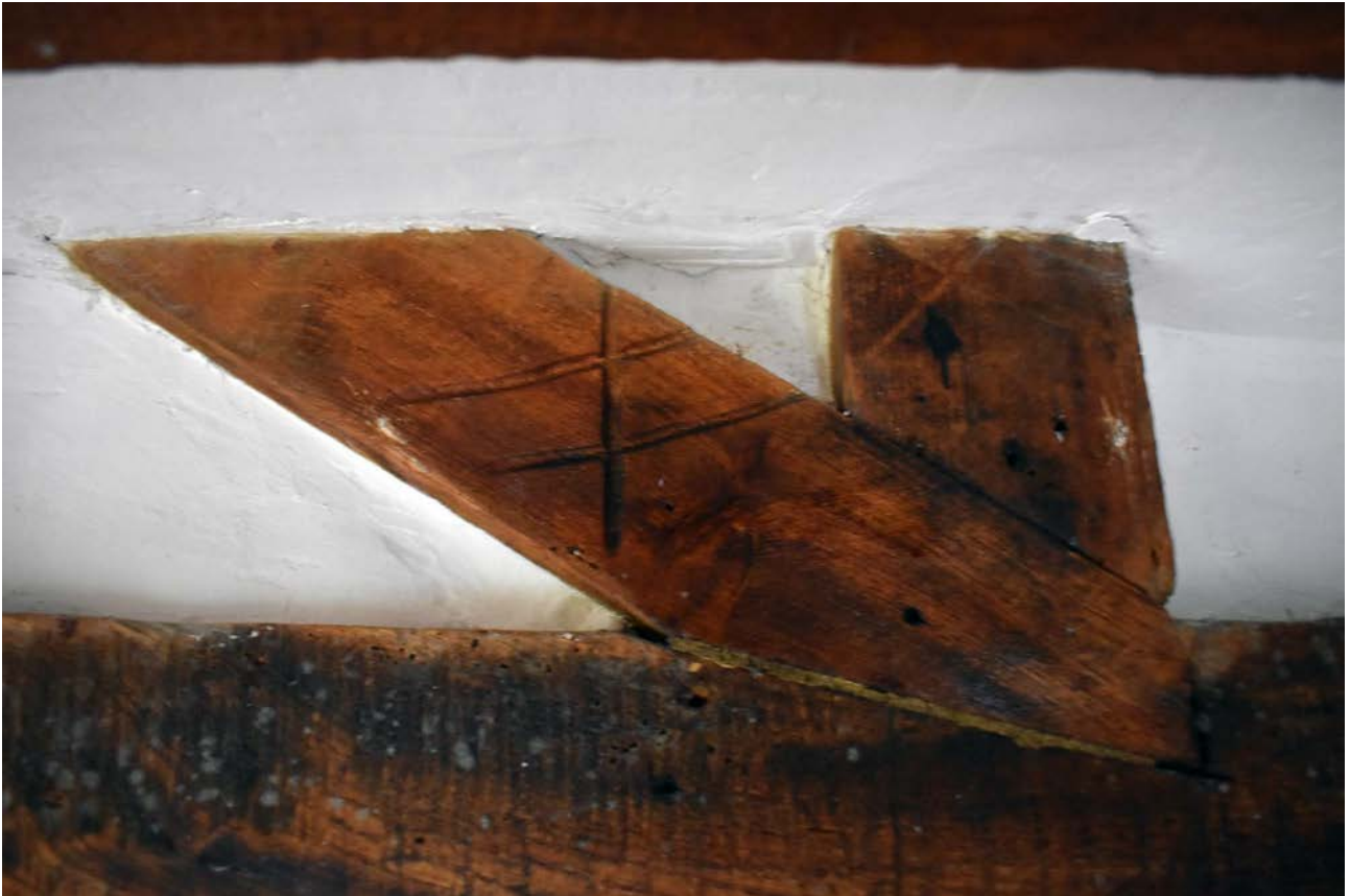
Plate 76: Ground floor, living room, north part, carpenters' marks
