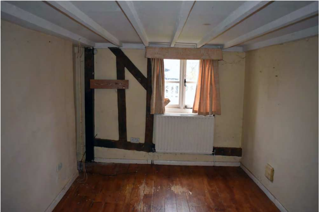
Plate 45: Ground floor, north bay, west wall
