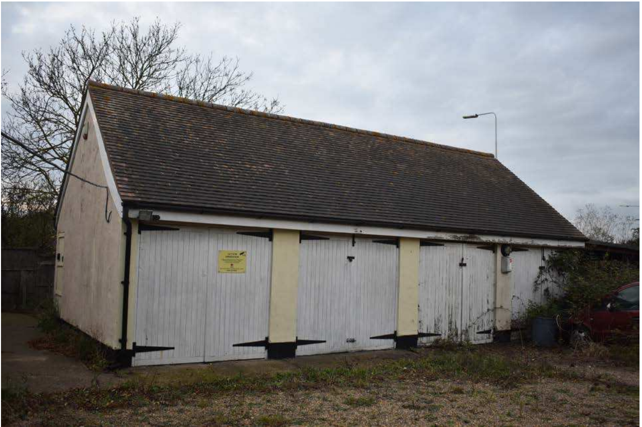
Plate 23: Garages belonging to Nos. 1 and 2 Grays Corner Cottages
