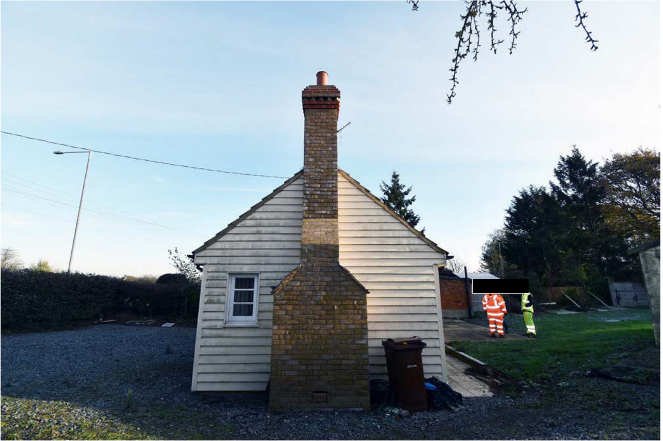
Plate 5: The west elevation of the extension to The Thatches
