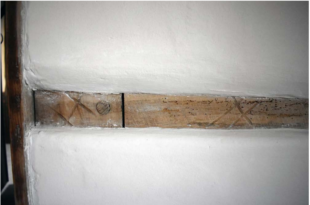
Plate 93: First floor, principal bedroom, west wall, north part, carpenters' marks
