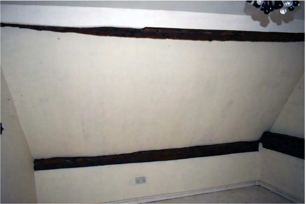
Plate 62: First floor, south bay, east wall
