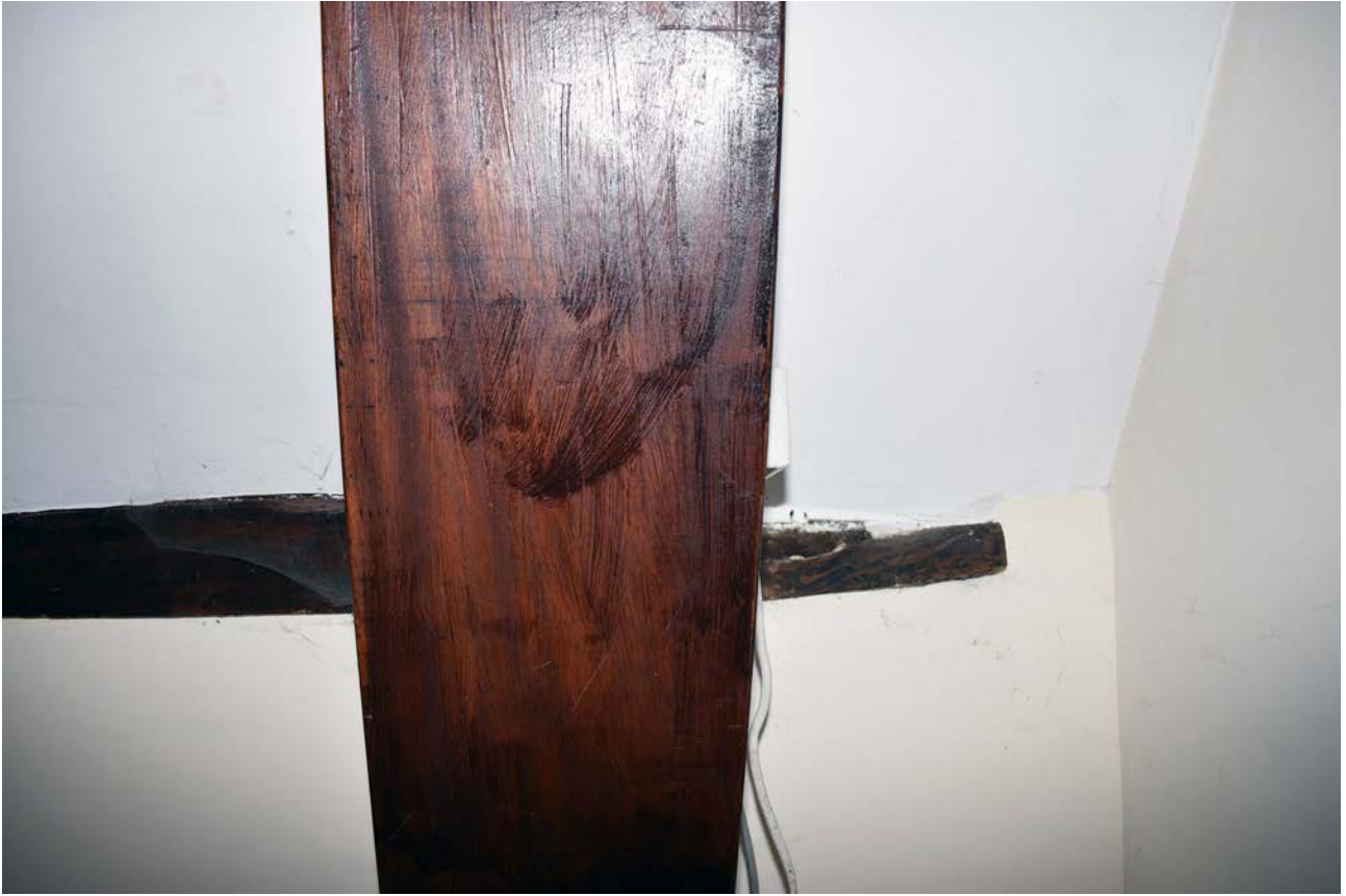
Plate 30: Encased timber and terminating wall plate in the south-west bedroom
