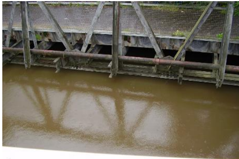
P716011/Tank Hill Bridge (Source: Environment Agency)
