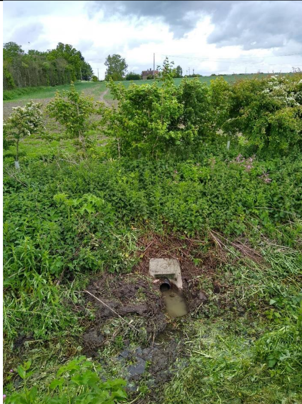
Photo ref. 6 – Direction north. Headwall in ditch – West Path. Outfall into ditch from drainage beneath hill.
