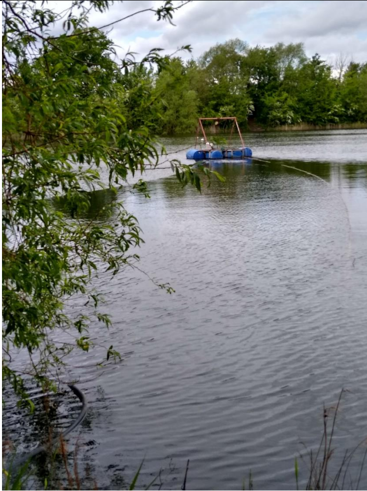
Photo ref. 3 – Direction east. Irrigation reservoir. Surface water abstraction pumps set up on blue float in centre of reservoir.
