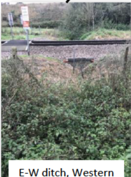
E-W ditch, Western end point, dry, heavily vegetated
