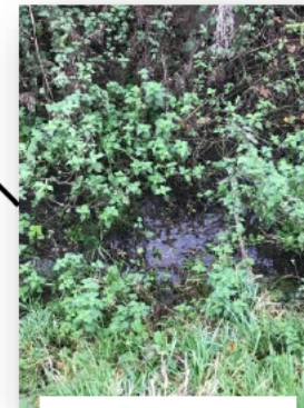
Mild flow noted on the outfall of deep drain – seeps and disappears within 10 meters to west.
