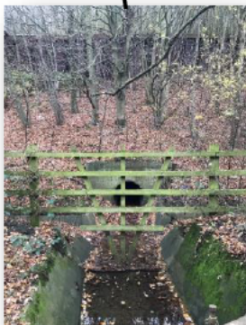
M25 Culvert outfall Looking East
