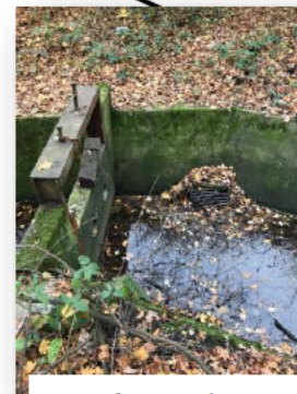
W of M25 Culvert No flow
