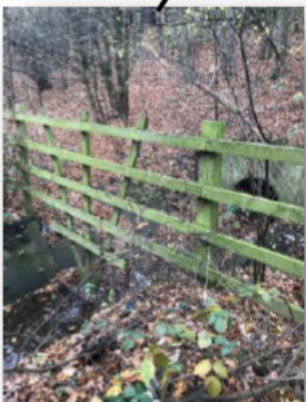
M25 Culvert outfall Looking North
