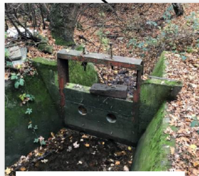
M25 Culvert outfall Looking West
