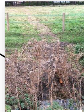
There is a small drainage pipe entering E-W ditch running N-S under the adjacent field.
