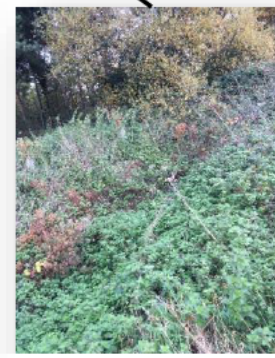
E-W ditch running from corner of pond is heavily vegetated and has a small patch of stagnant water at base
