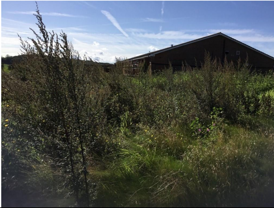
GD-2S05ZZZ1– Possible location of a discharge to ground, between the reception and the abstraction borehole, dense vegetation.
