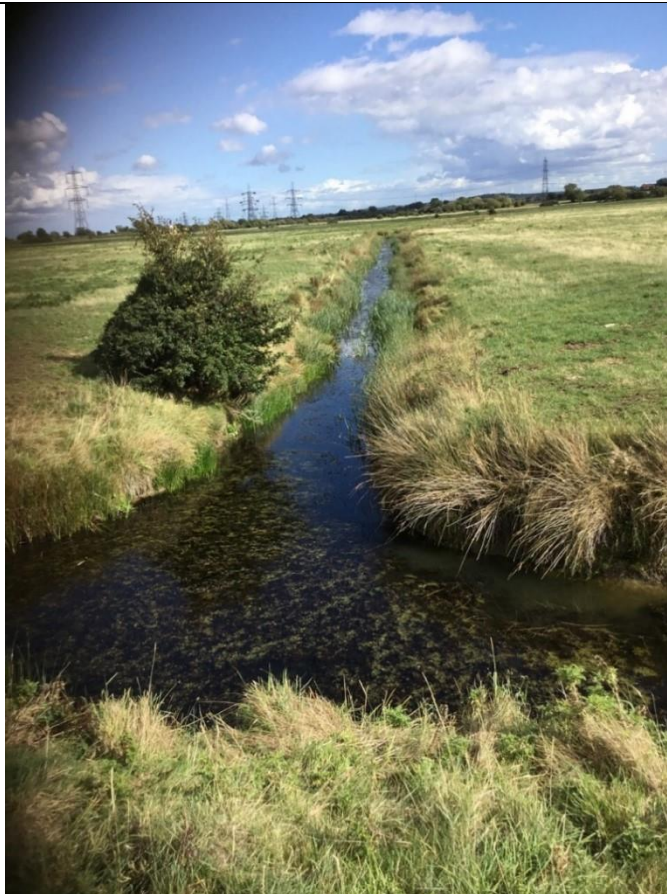
DI-1S06ZZZ1 – Filborough Marshes drain network. Algae and small trees present on southern ditches
