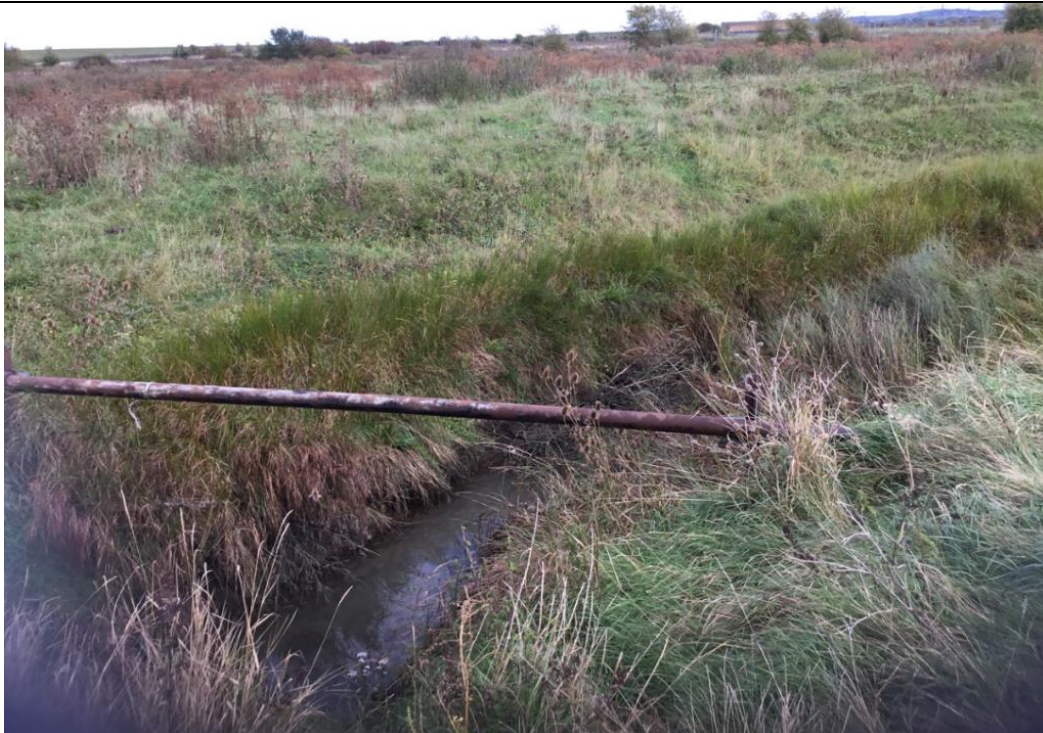
AS-1S05ZZZ1– Gravesham Borough Council, between the Firefighting training centre and the Milton Rifle Range. Drainage ditch, unused pipe
