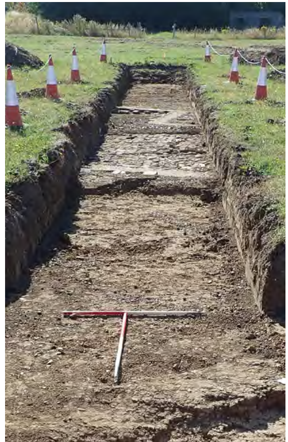
Plate 23: Trench 97 showing concrete foundations and brick floor of airfield building, facing south-east
