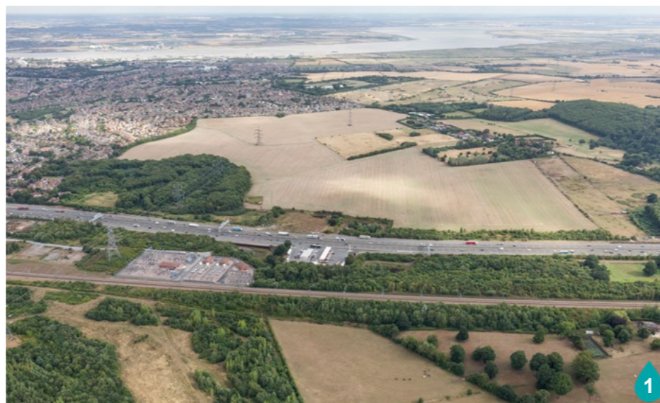
View of proposed M2/A2/Lower Thames Crossing junction location
