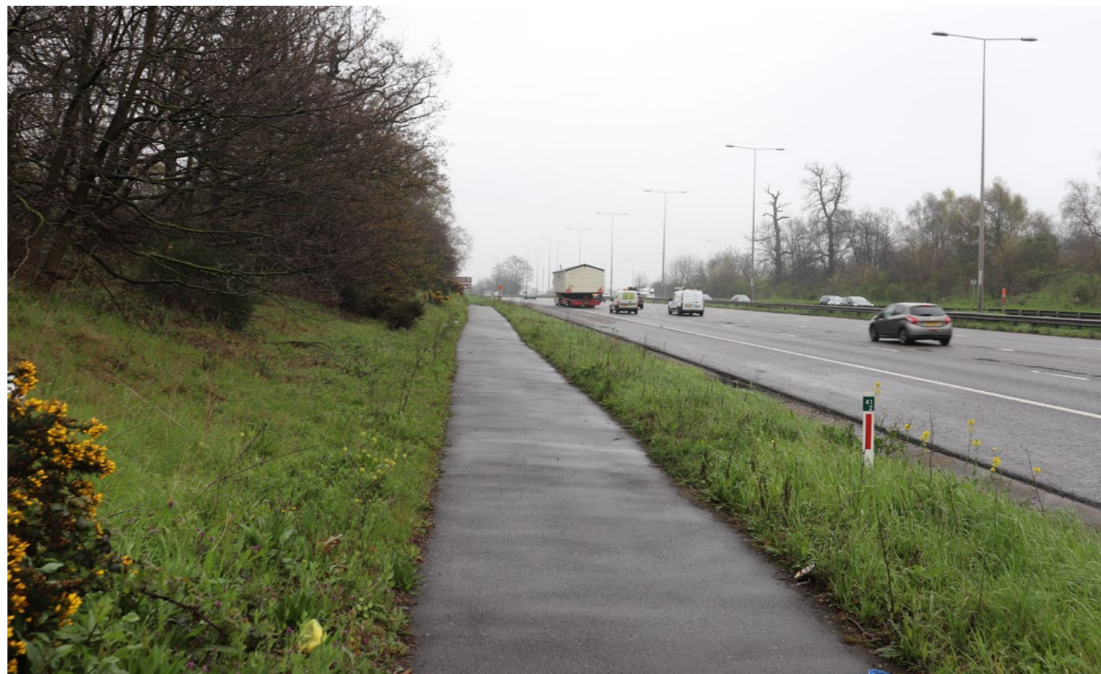
Existing vegetation along the A2/M2 Corridor
