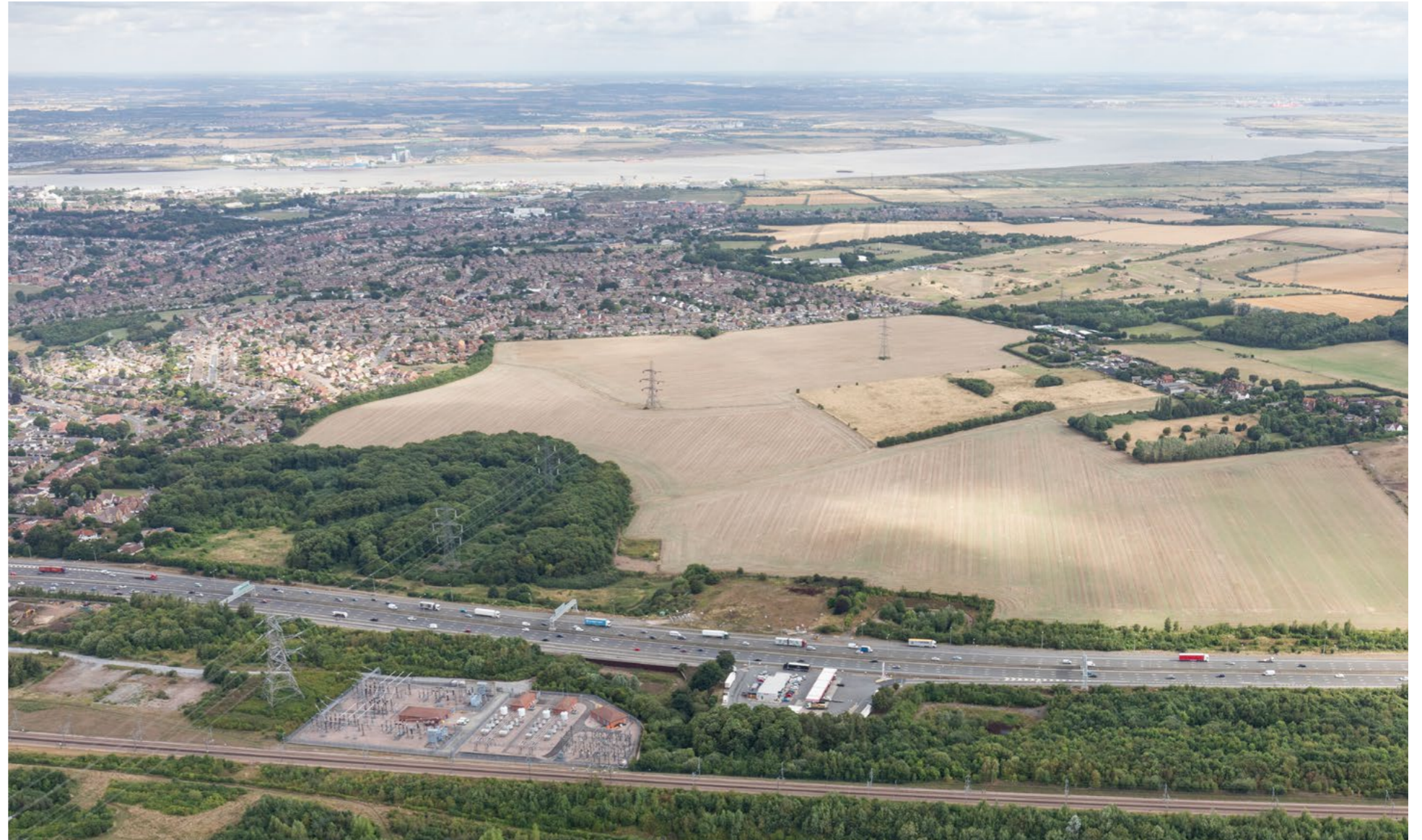
Existing view of overhead powerlines, looking north towards the River Thames, with the A2/M2 Corridor in the foreground
