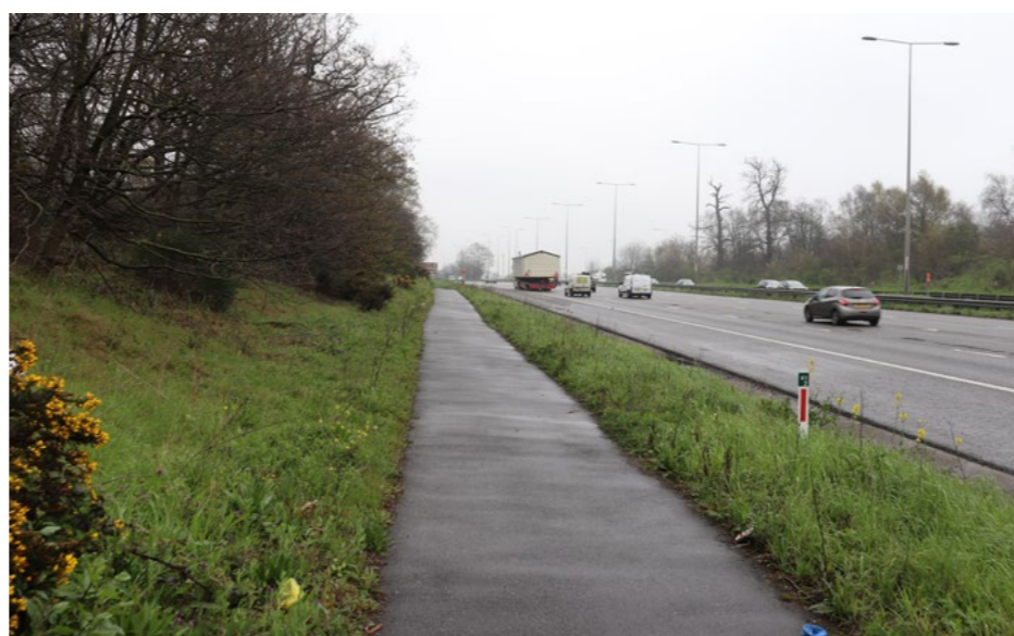
Existing WCH route adjacent to the A2
