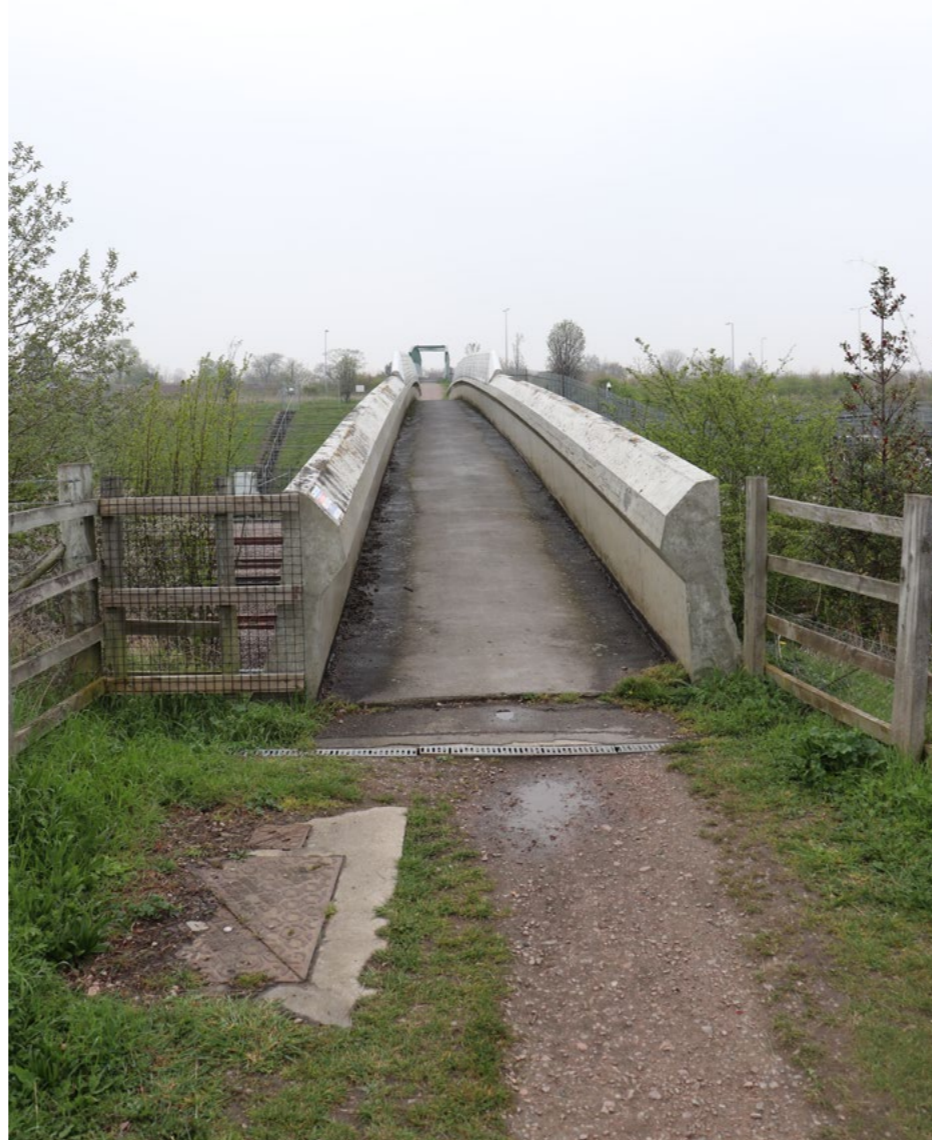
Existing WCH bridge over HS1
