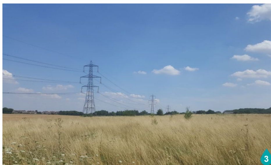
Views of overhead powerlines
