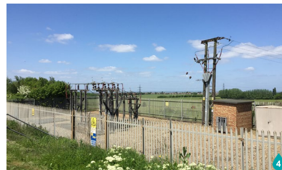
Existing view of switching station adjacent to A2
