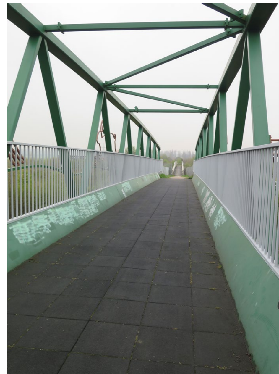
Existing Hares bridge over the A2
