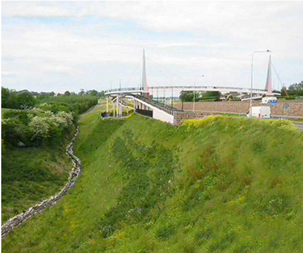
Figure 2-2 - Seeded Reinforced Earth Embankment
