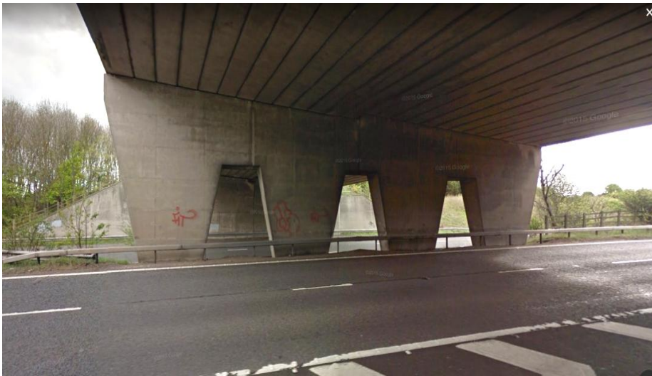
General View of Pier
