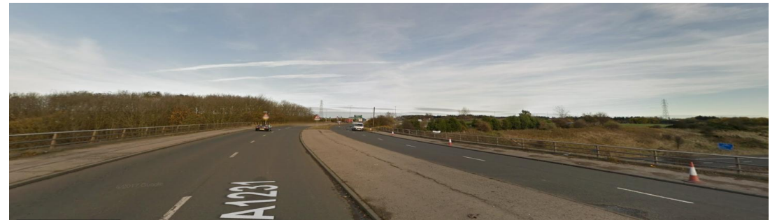
General View of Carriageway
